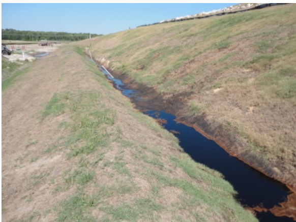
South Side Slope Toe Drain
