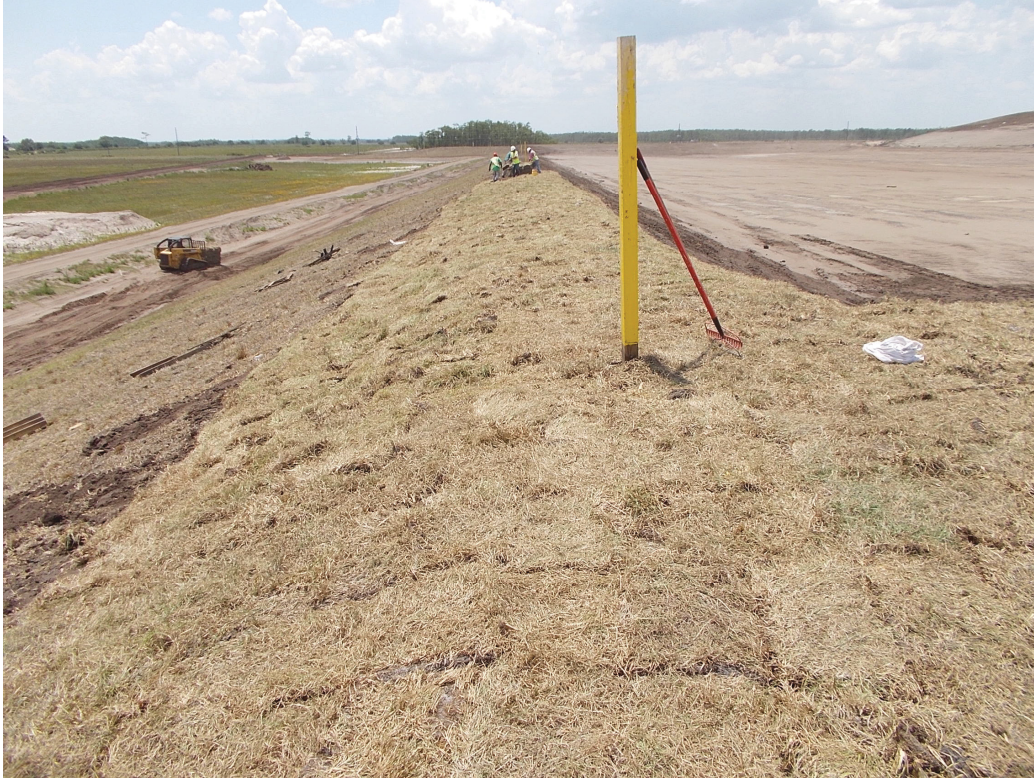
Replacement of Sod on Intercell Berm
