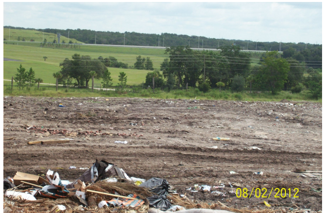
Compacted and Covered Waste
