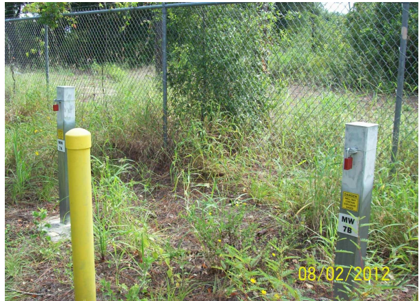
Perimeter Monitoring Wells
