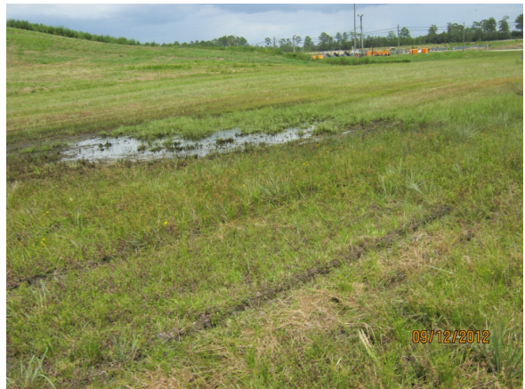
Ponding on closed, Class 1
