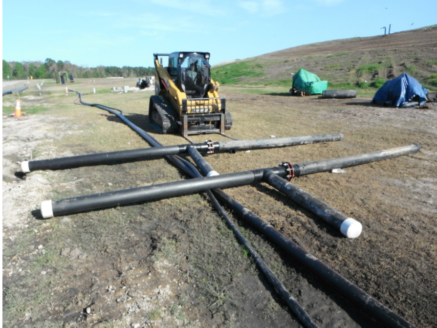
Horizontal Well Drip Trap Fabrication
