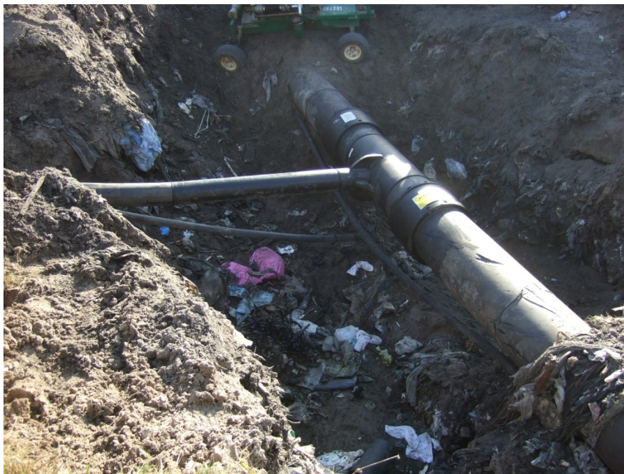
Lateral Connection to Header via Electrofusion Collar
