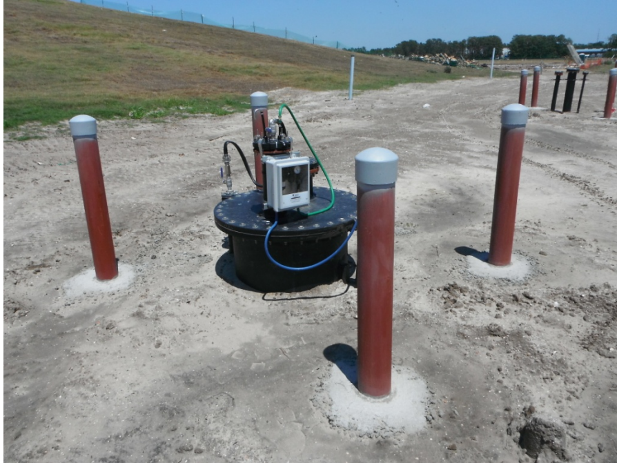
Condensate Sump Completion
