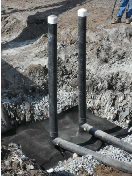
Horizontal Well Drip Trap Riser
