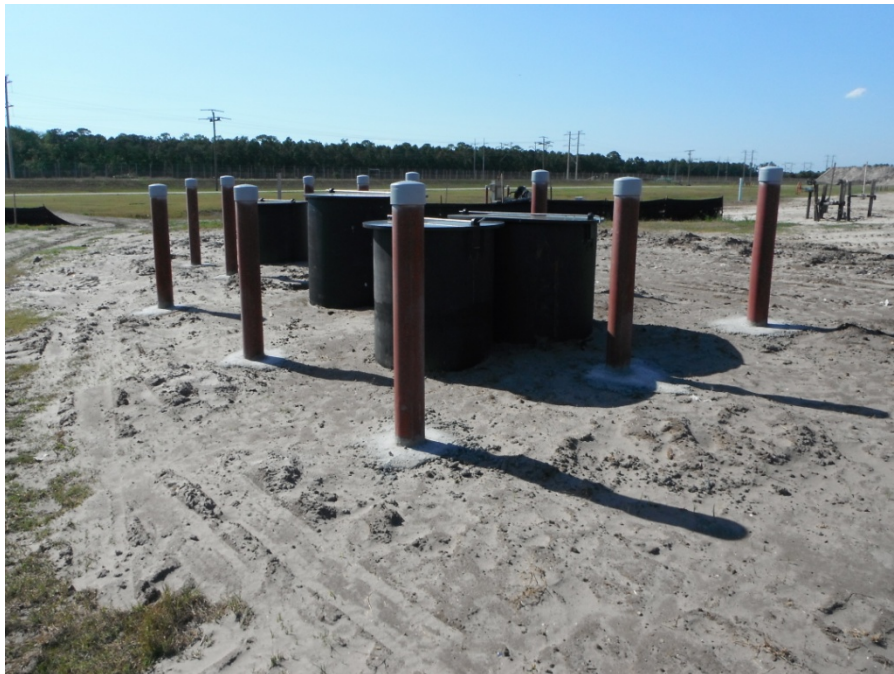
Isolation Valve Vaults
