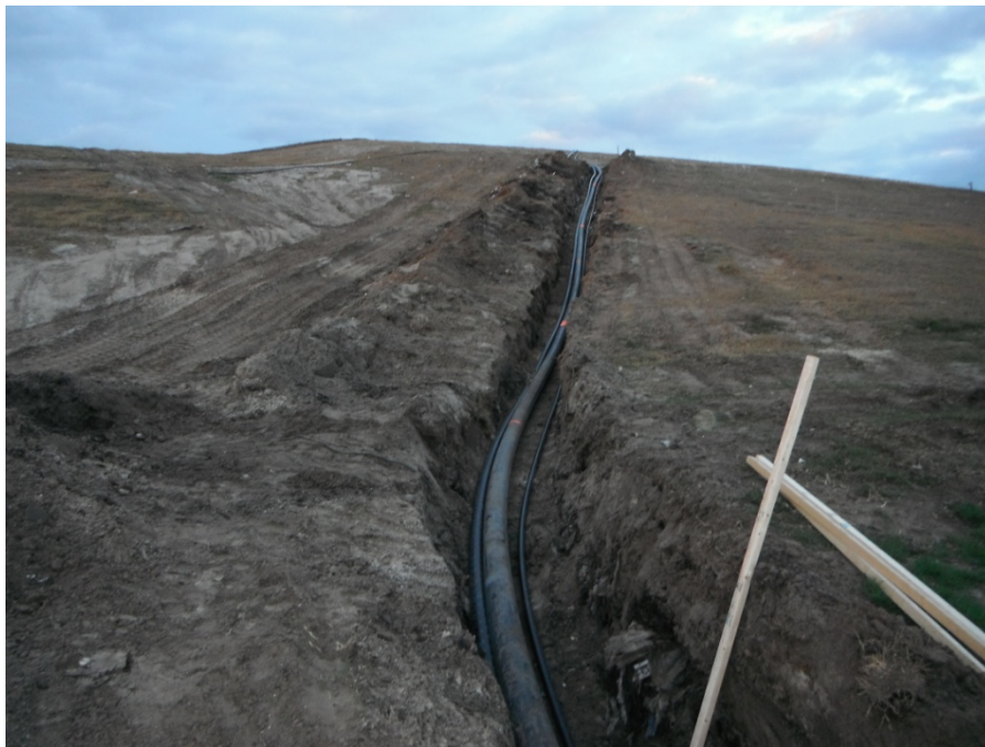
8" Sub-Header Installation
