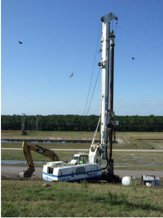
Vertical Well Installation
