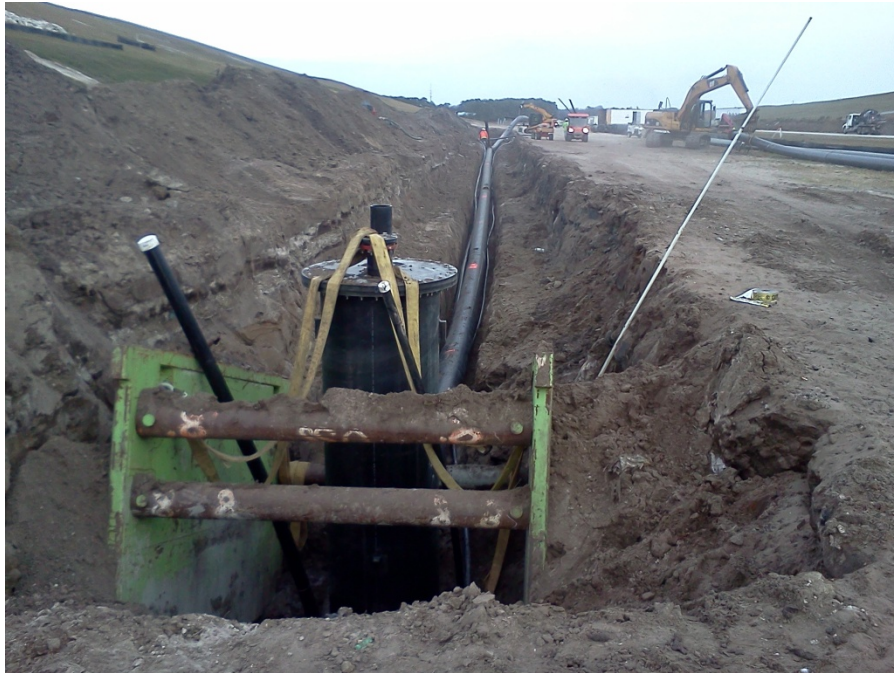
South Slope Condensate Sump Installation
