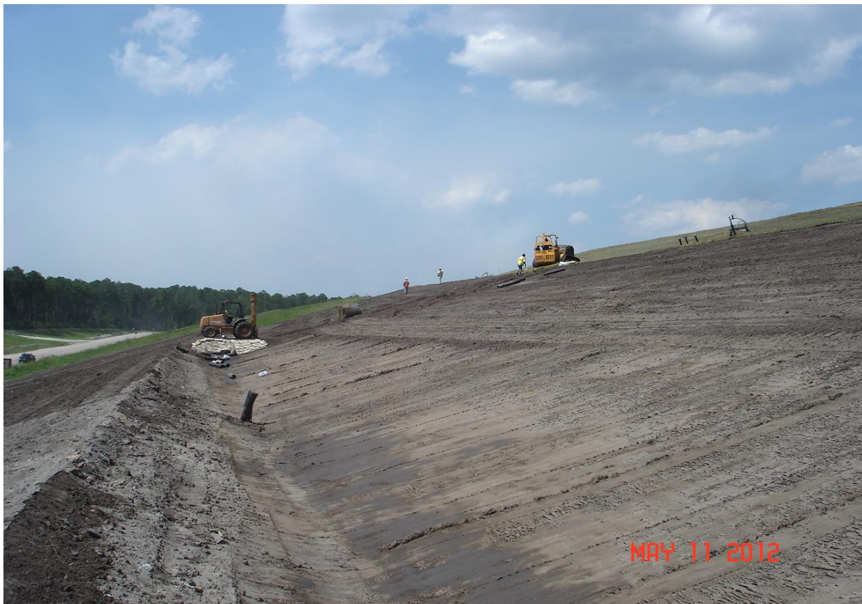
Placing Sod (Phase IV)
