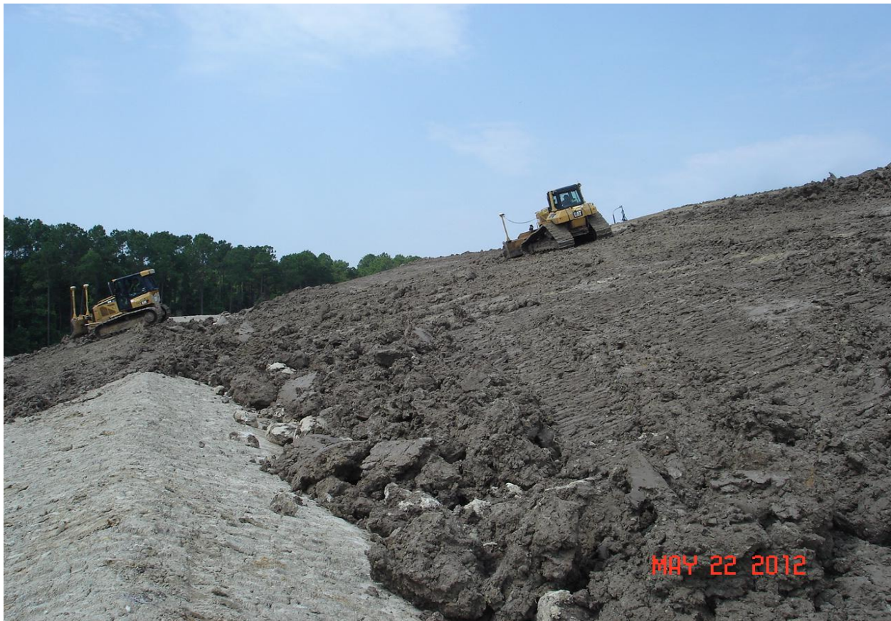
Grading 2 nd Lift Clay (Phase I)
