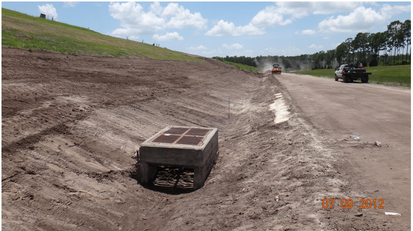
Regraded Perimeter Road Swale - Phase IV
