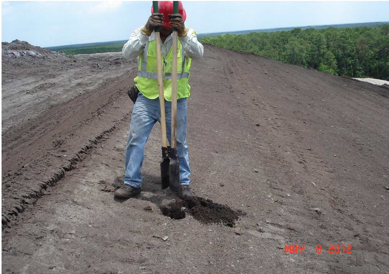
Top Soil Thickness Checks (Phase II)
