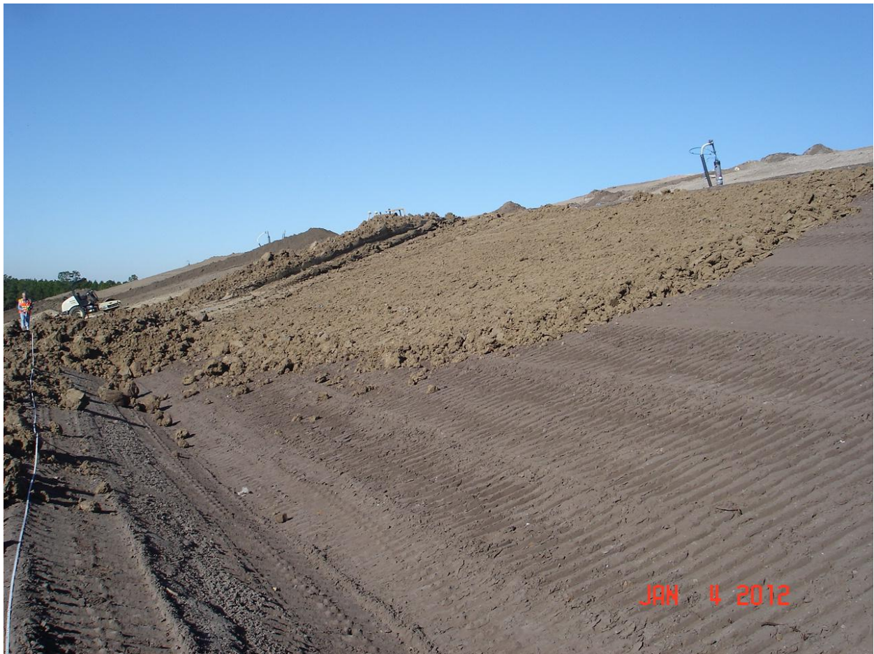
Placing First Lift Clay (Phase 3)
