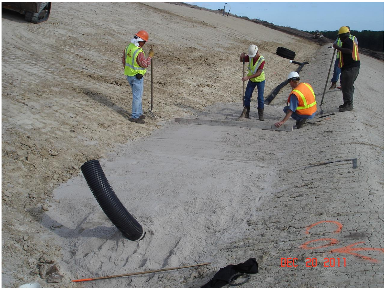
Underdrain Sand Leveling Terrace 3 – Phase III
