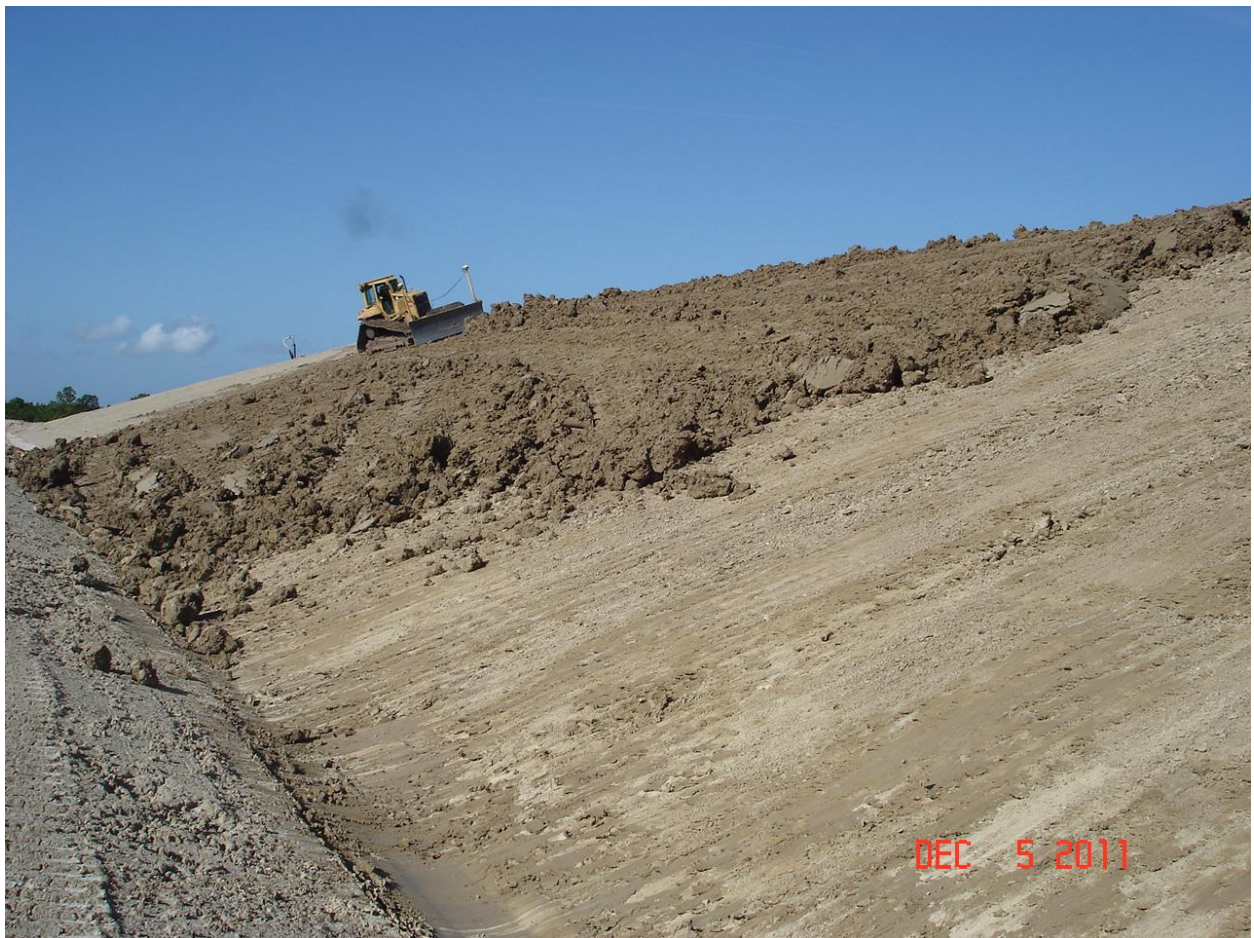
Second Lift Clay Placement – Phase III
