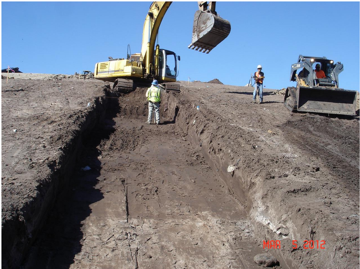
Excavate Initial Cover at Downcomer D-38 (Phase II)
