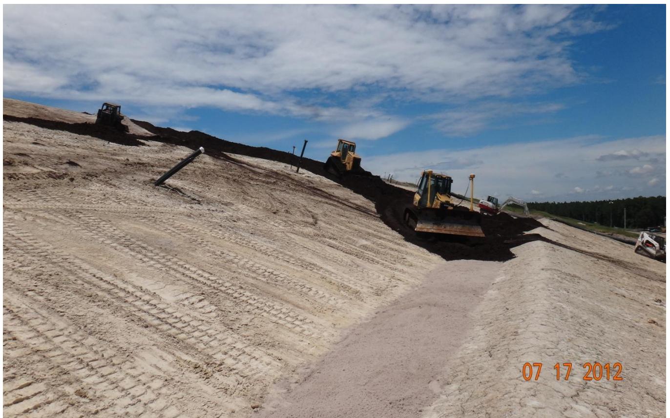
Placing Top Soil – Phase I
