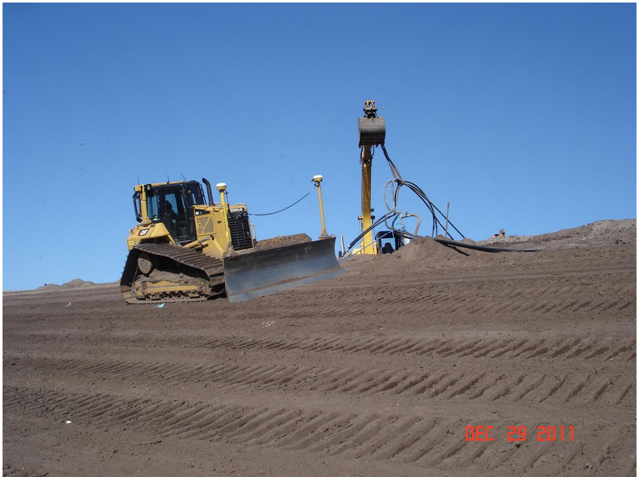
Final Grading Initial Cover around Air Lines – Phase III
