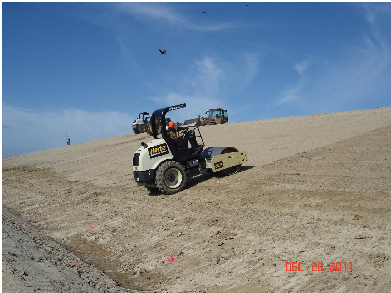
Seal Second Lift Clay – Preparation for Underdrain - Phase III
