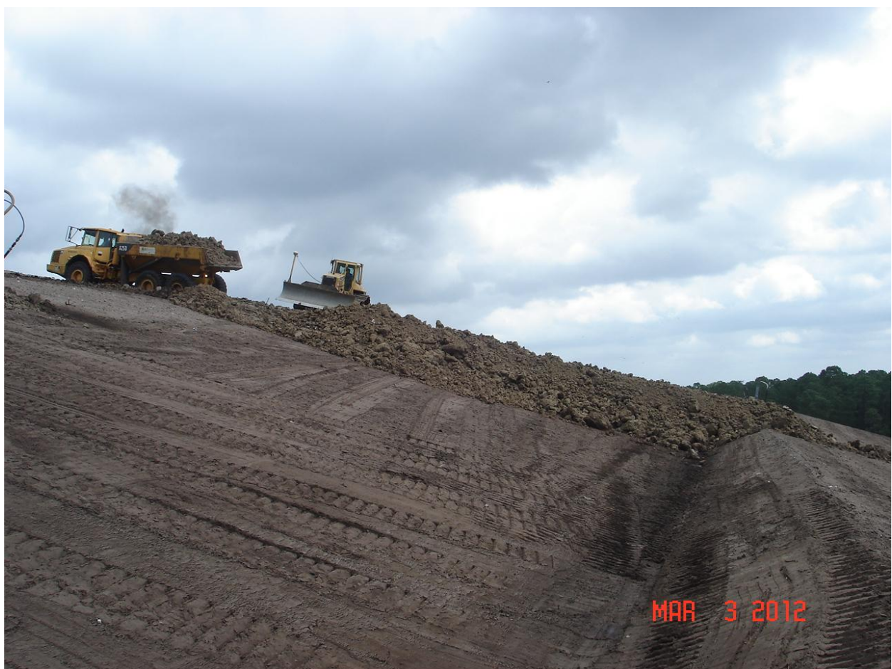
Placing First Lift Clay (Phase II)
