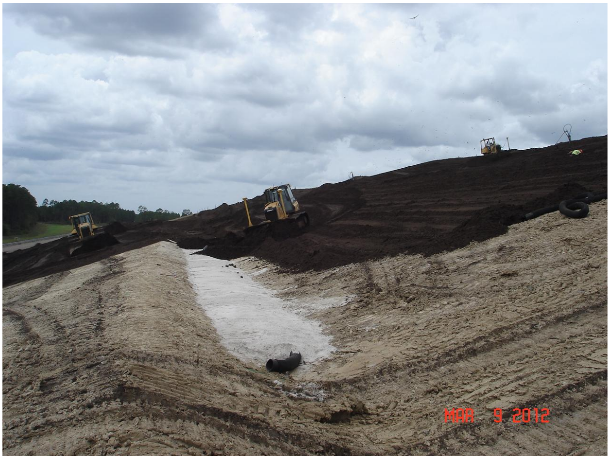
Top Soil Placement (Phase II) Terrace Underdrain installation (Phase II)
