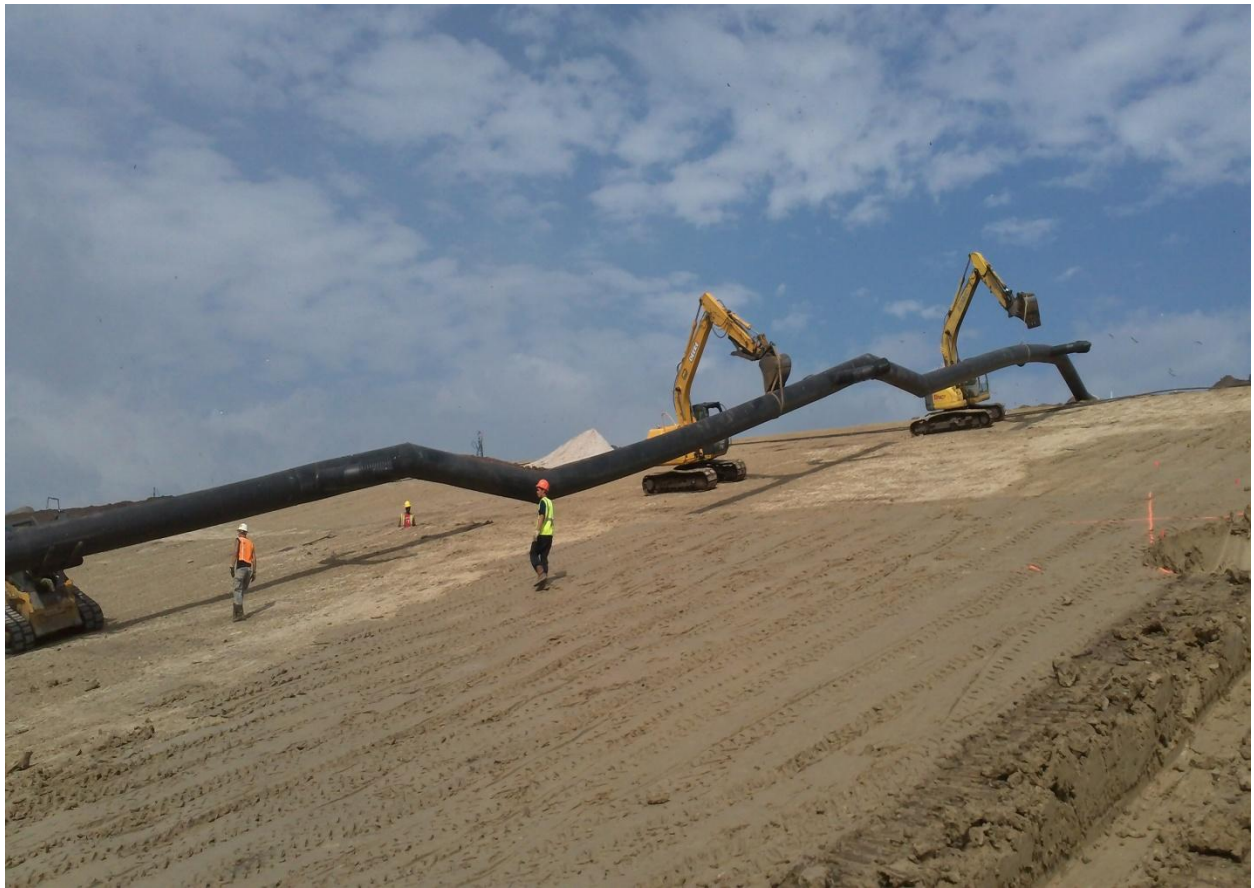
Moving Downcomer D-41 to Trench (Phase II)
