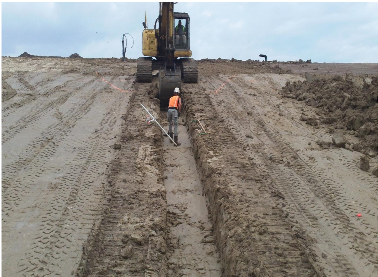
Clay Excavation for D-41 (Phase II)
