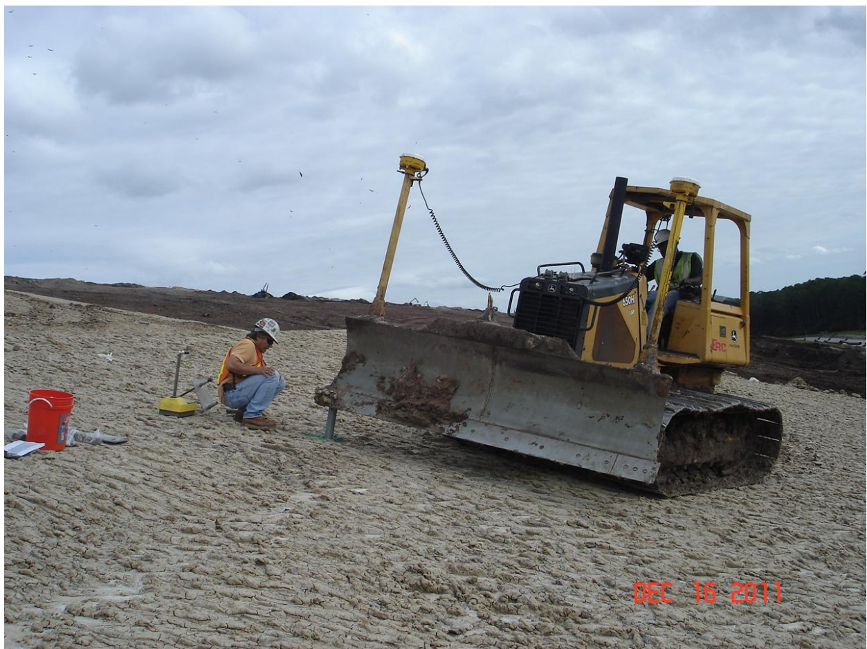
Pushing Permanent Tube Second Lift Clay – Phase III
