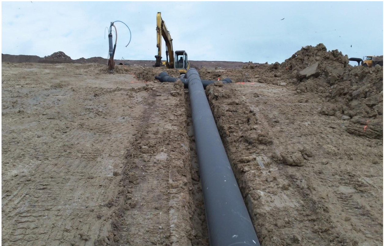
Downcomer D-41 in Clay Trench (Phase II)
