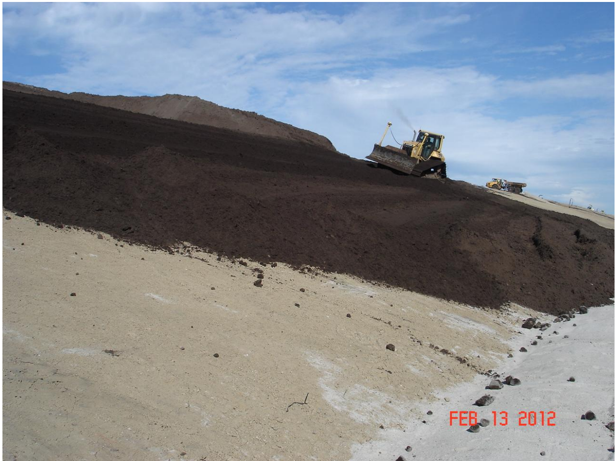
Placing Top Soil (Phase III)
