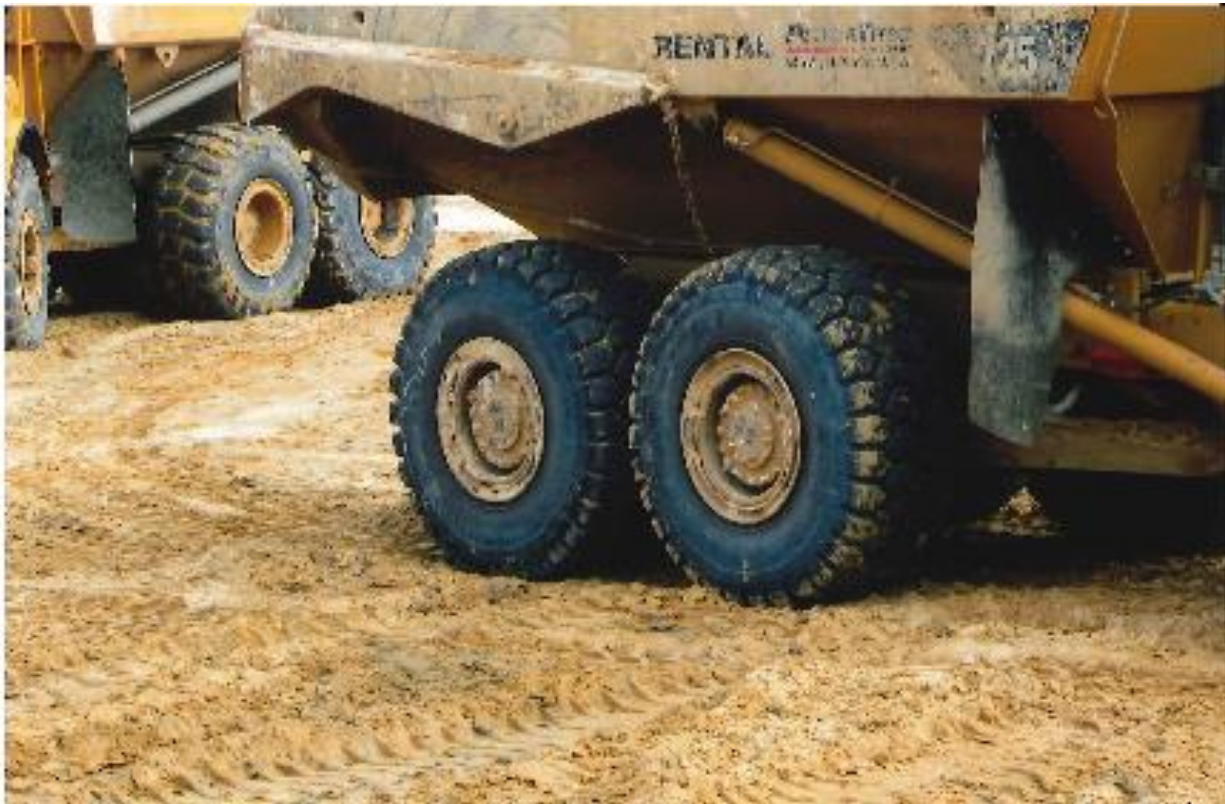
Proof rolling was performed throughout Cell-3 Placement.
