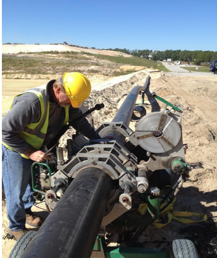
Fusing the forcemain pipe.
