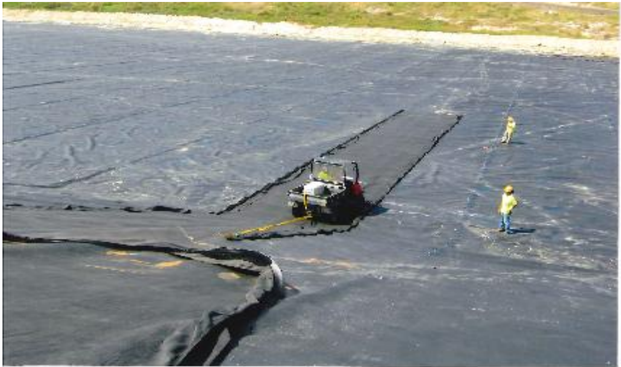
Geocomposite being pulled into place using an ATV.
