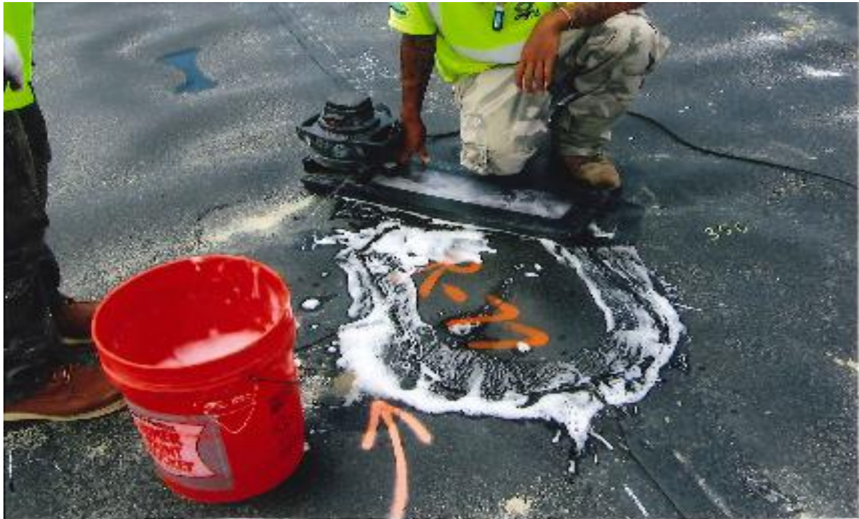
All extrusion welds including tie-in seams and repairs were vacuum tested.
