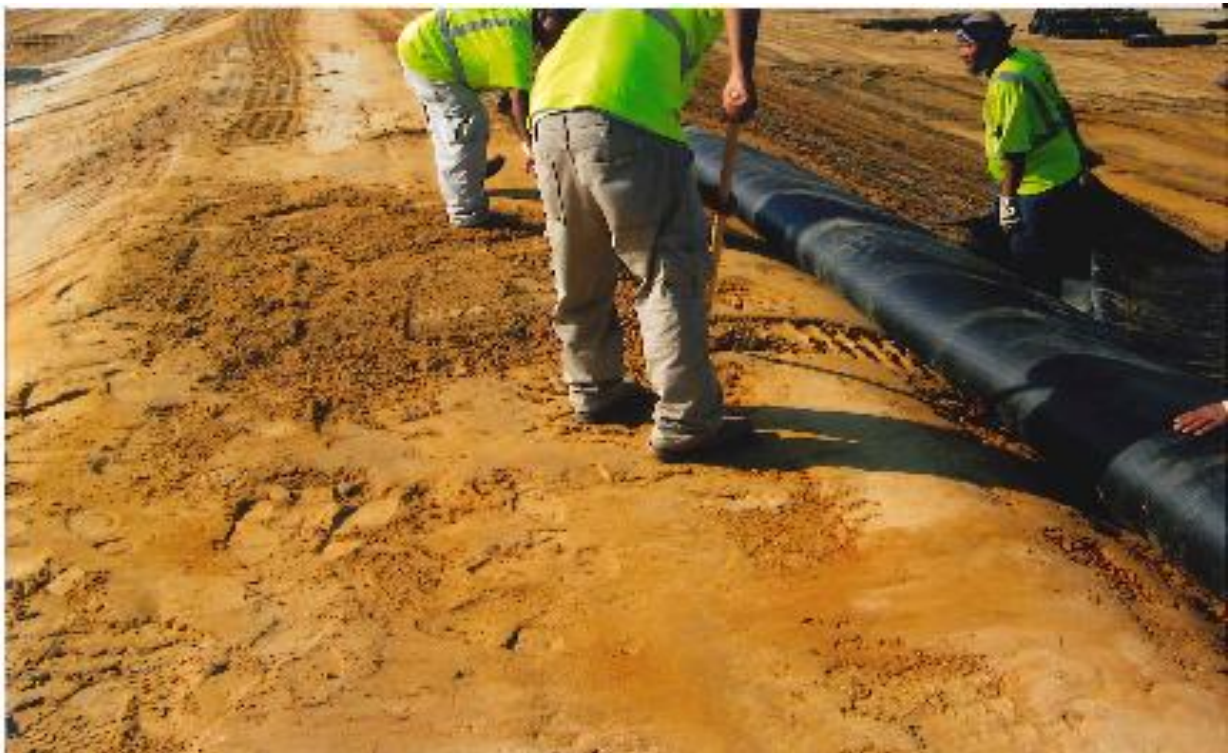
Tracks made in sub base was hand raked to ensure a smooth surface.
