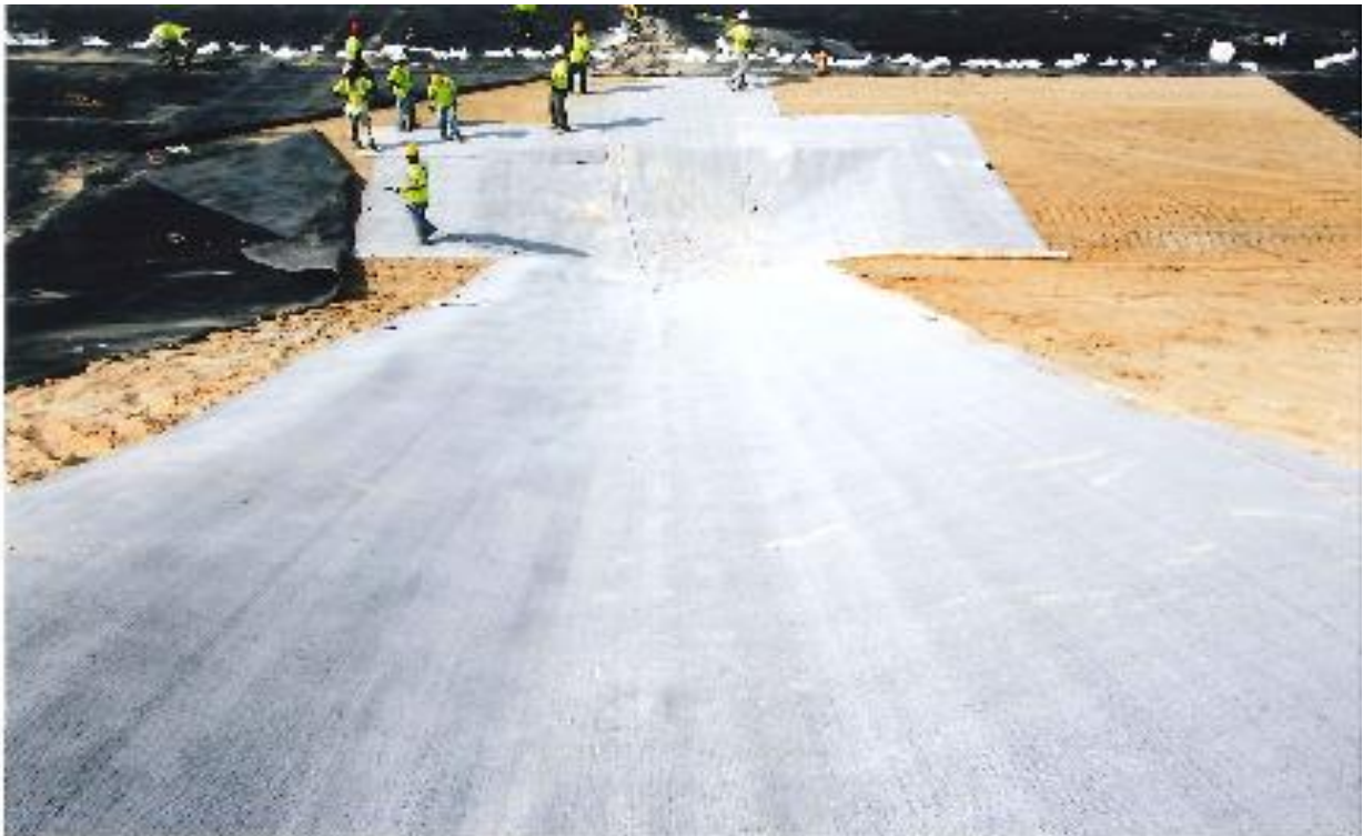
GCL in the sump and up the south berm riser trench.
