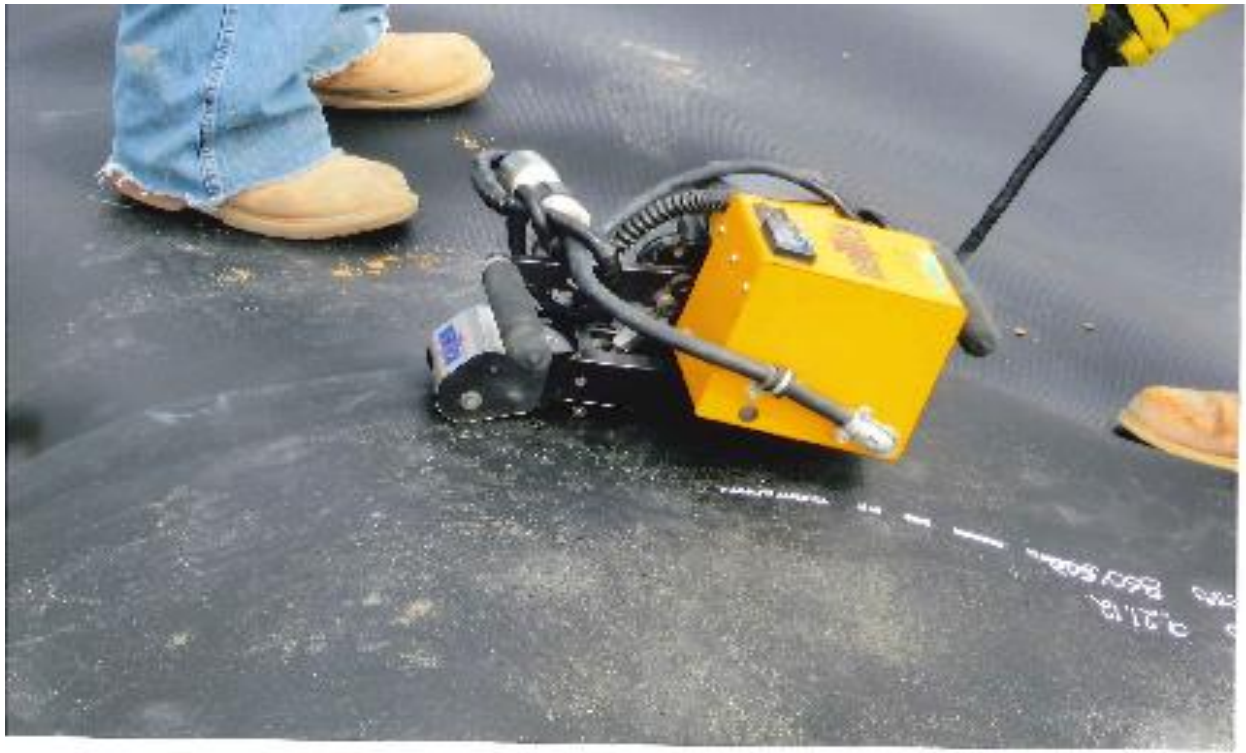
Panel seaming was performed using a double track wedge welder.
