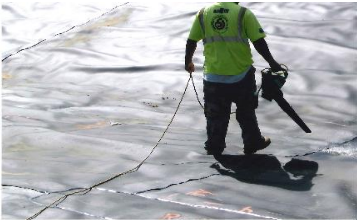
A leaf blower was used to clean the liner in front of the geocomposite installation.
