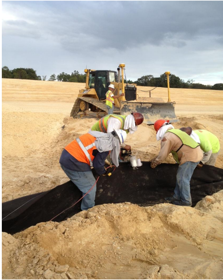
All geotextile around the drainage and sump stone was wrapped closed and then sealed by sewing.
