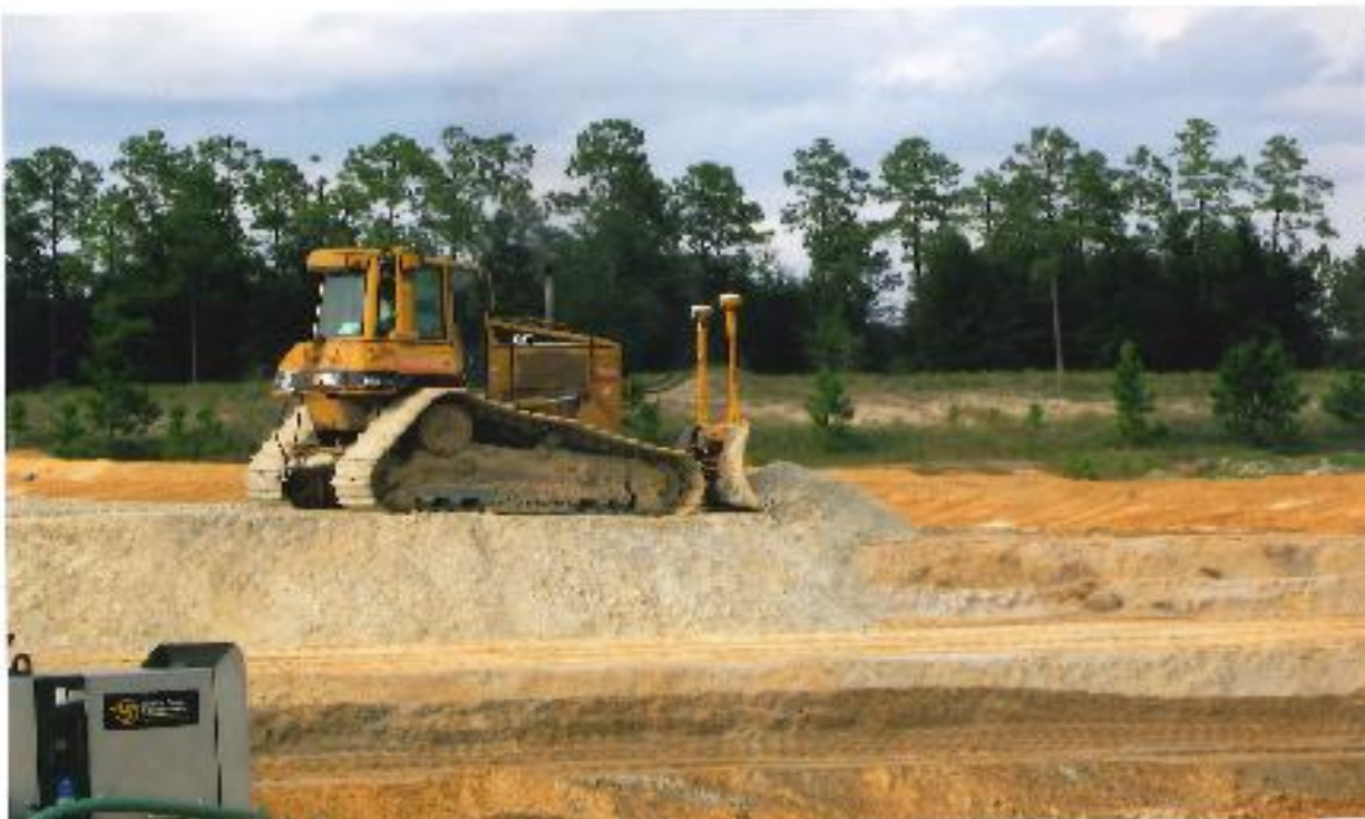
A D6 Dozer with GPS was used to control lift thickness and soil elevations
