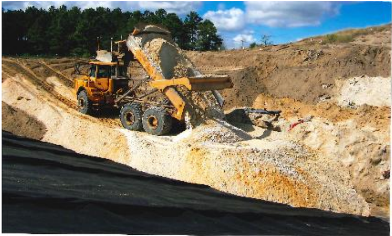
Protective soil placement started at the Southwest corner of Cell-3. All trucks were kept on a minimum of 3.5 feet of sand.
