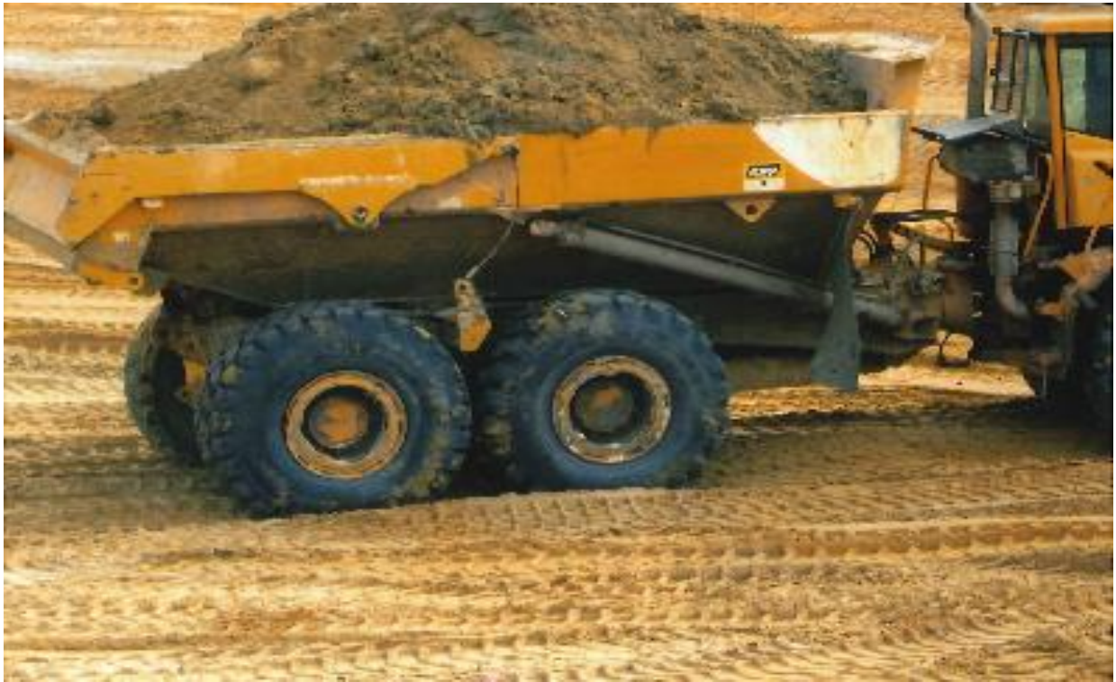
View of a loaded truck on the cell floor, proof rolling.
