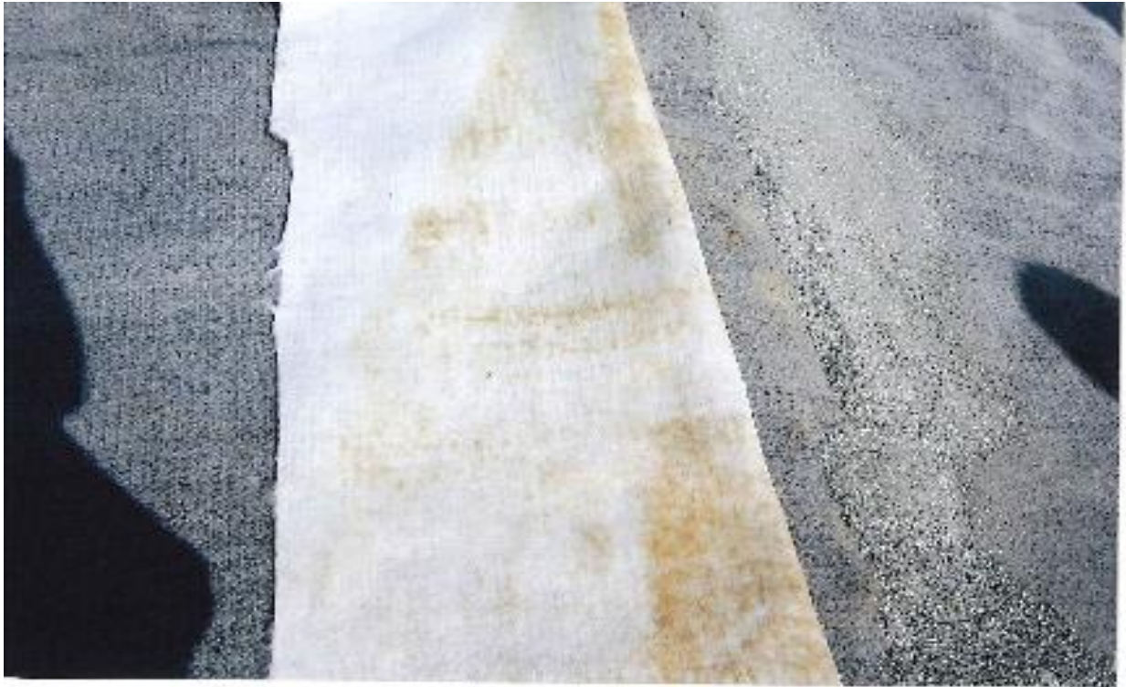
Powder bentonite was placed where the GCL panel overlaps.
