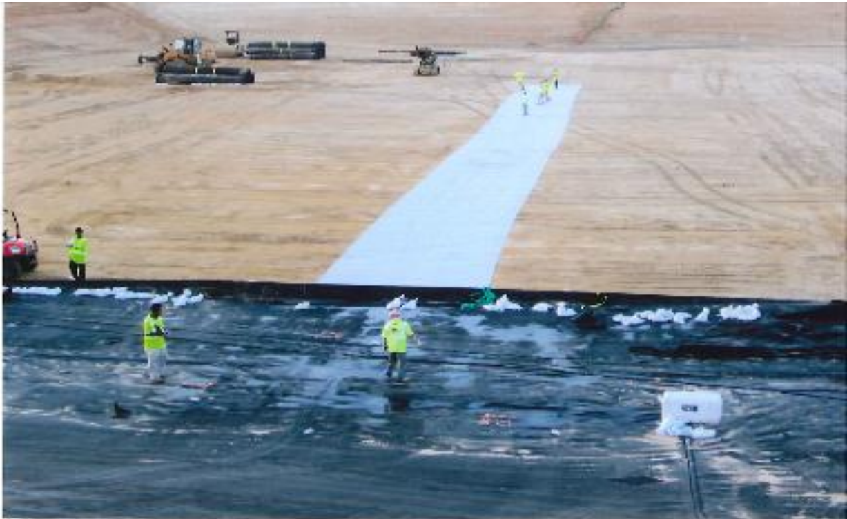
View of geosynthetic clay liner (GCL) at the center of Cell-3 under the leachate trench.
