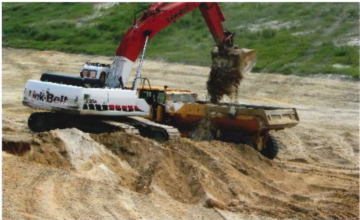
Excess fill in Cell-3 was used for berm construction at the North and South Sides of Cell-3.
