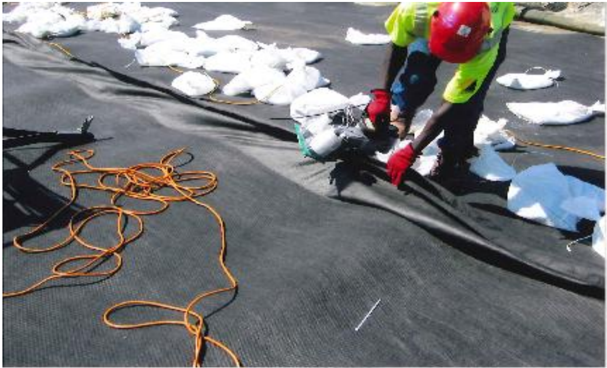
All geotextile seams were sewn.
