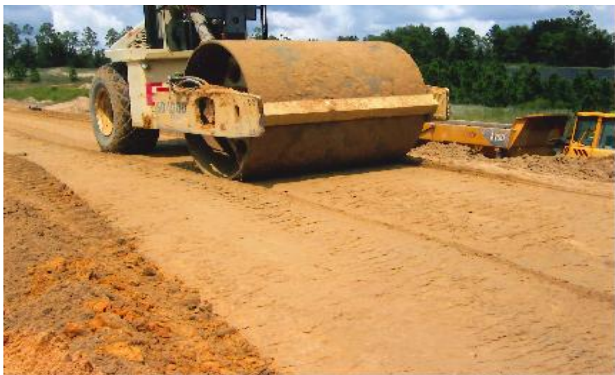
Each lift was compacted with a Drum Vibrator Roller.
