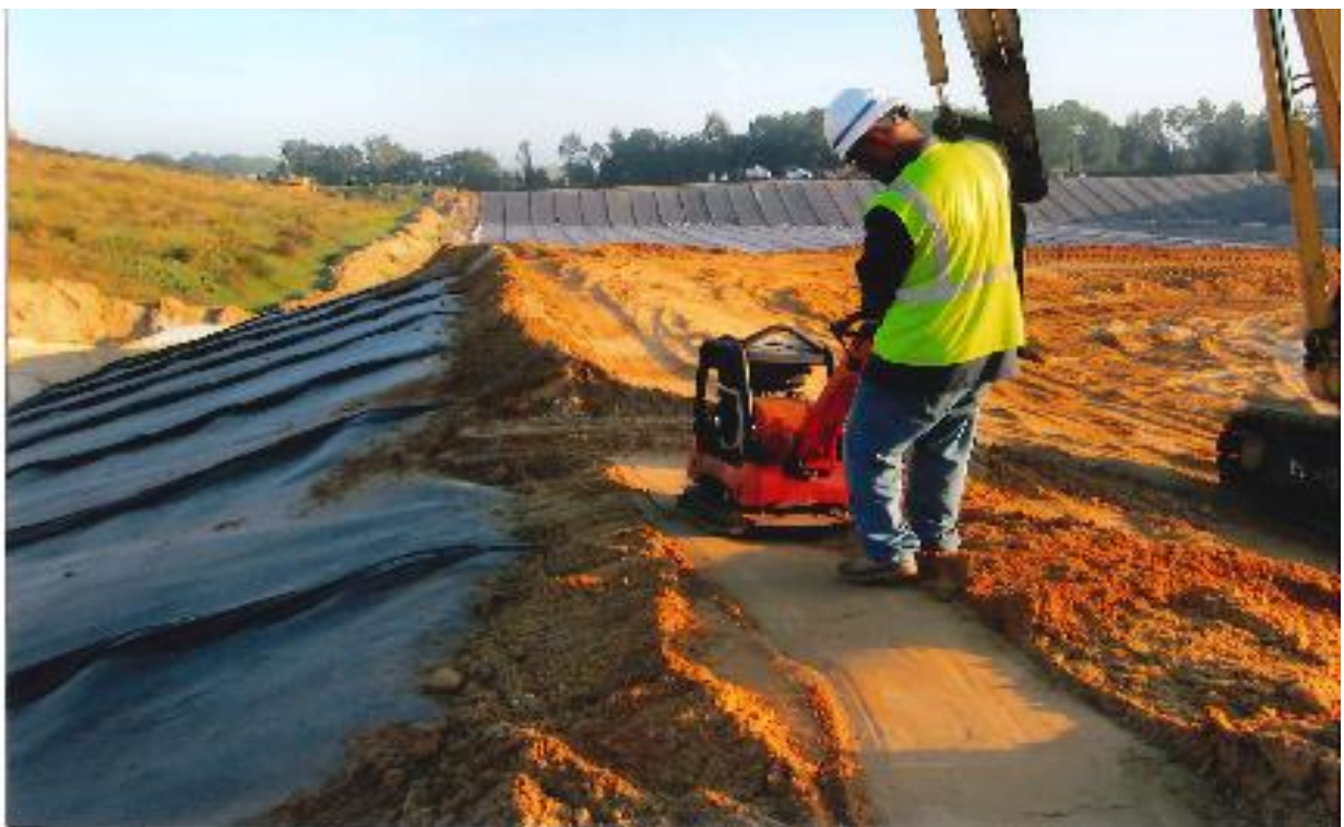
Protective cover sand in the anchor trench was compacted and tested.
