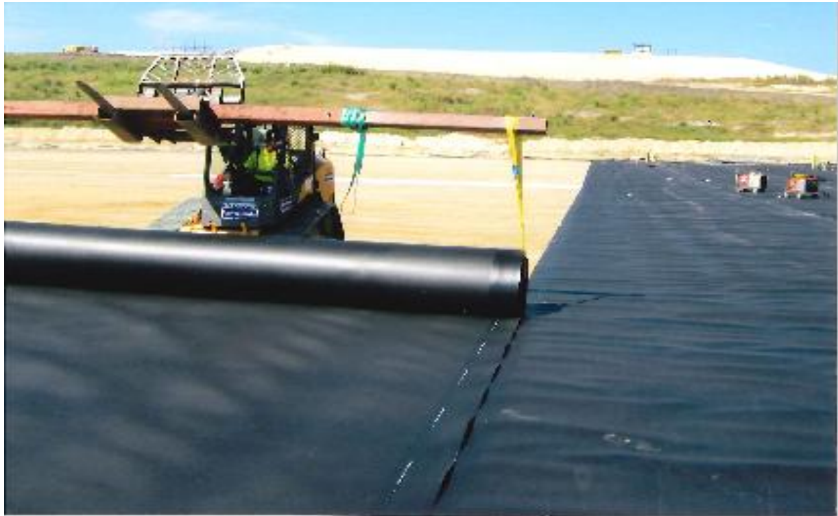
The liner crew deployed rolls of liner using a skid steer with a spreader bar.
