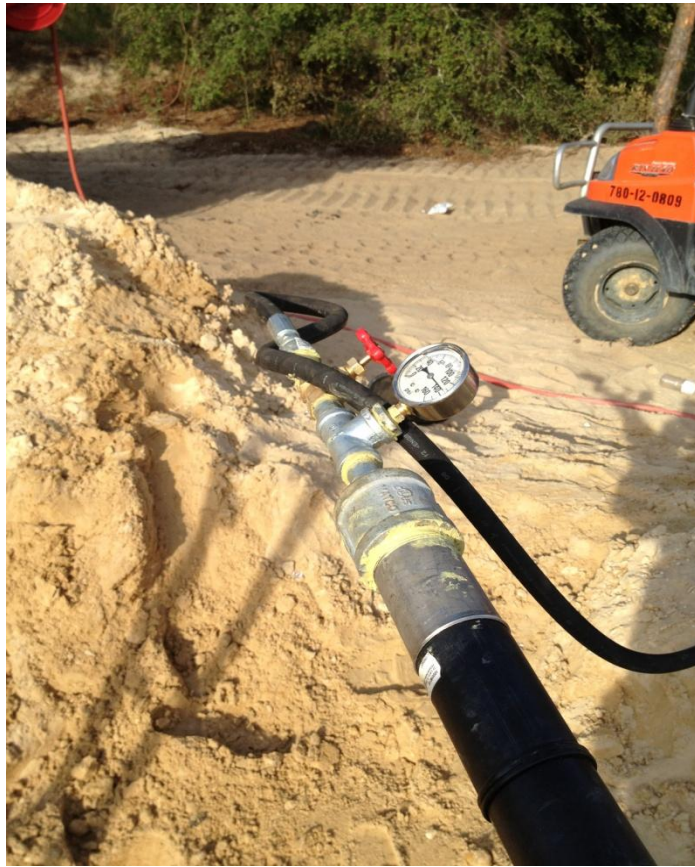
Hydro testing the forcemain pipe in place.
