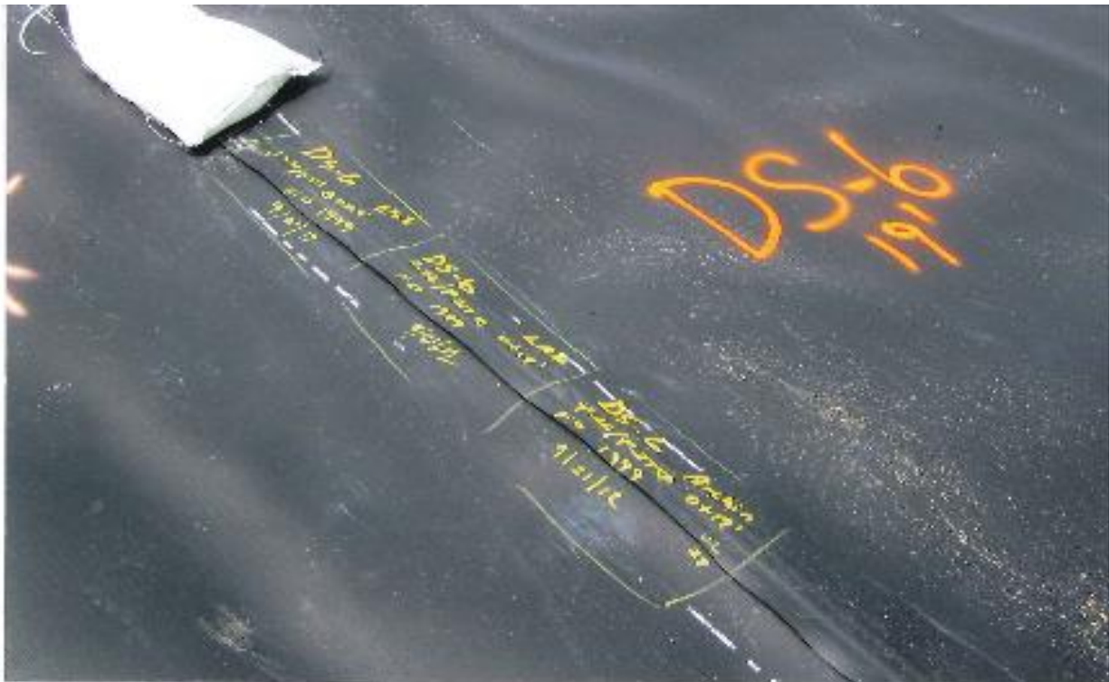
Destructive seam samples were marked on completed seams.
