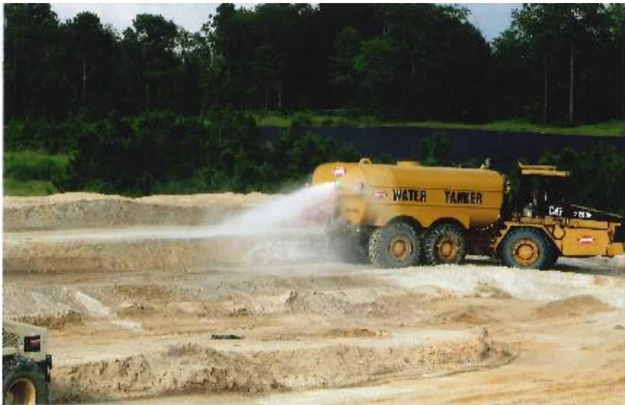
A Water Tanker was used to add moisture to the fill as it was placed.
