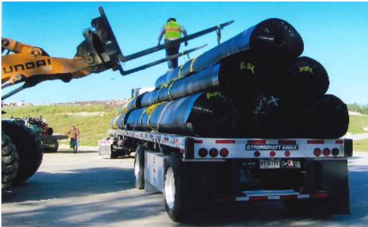
Geosynthetic materials were unloaded and stored until used. Inventor was made as the materials were unloaded.
