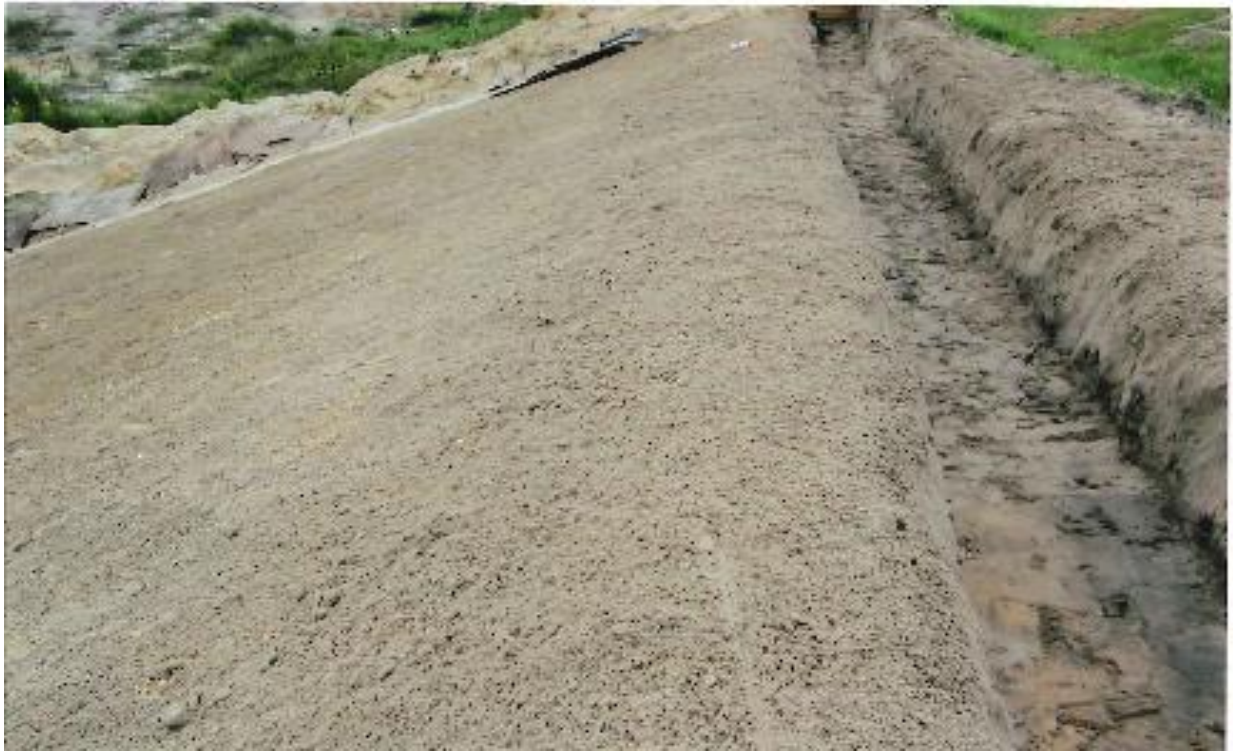
The completed anchor trench.
