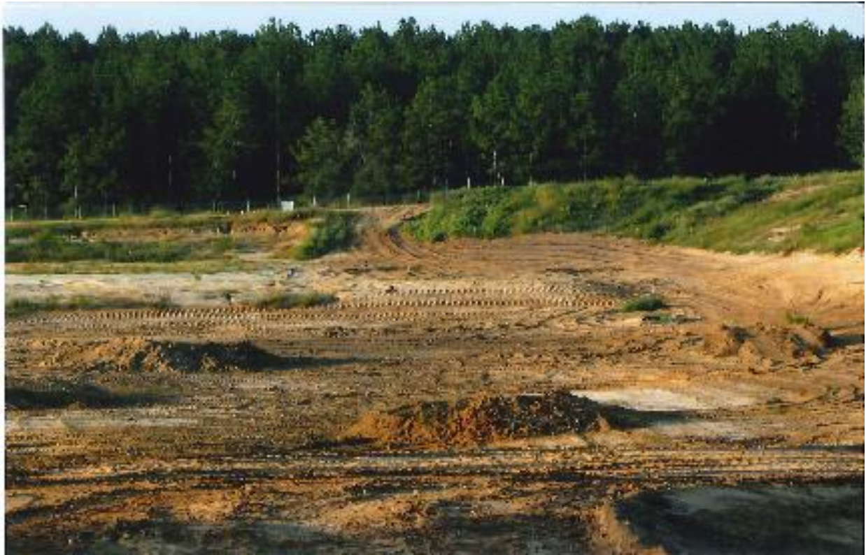
Cell-3 prior to excavating to subgrade elevation.
