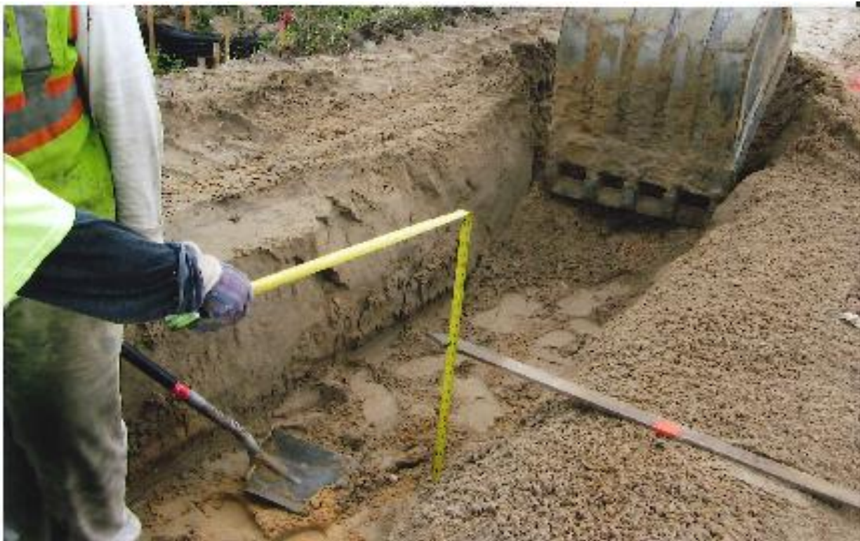
Anchor trench excavation. The 2 foot elevation was checked during excavation.
