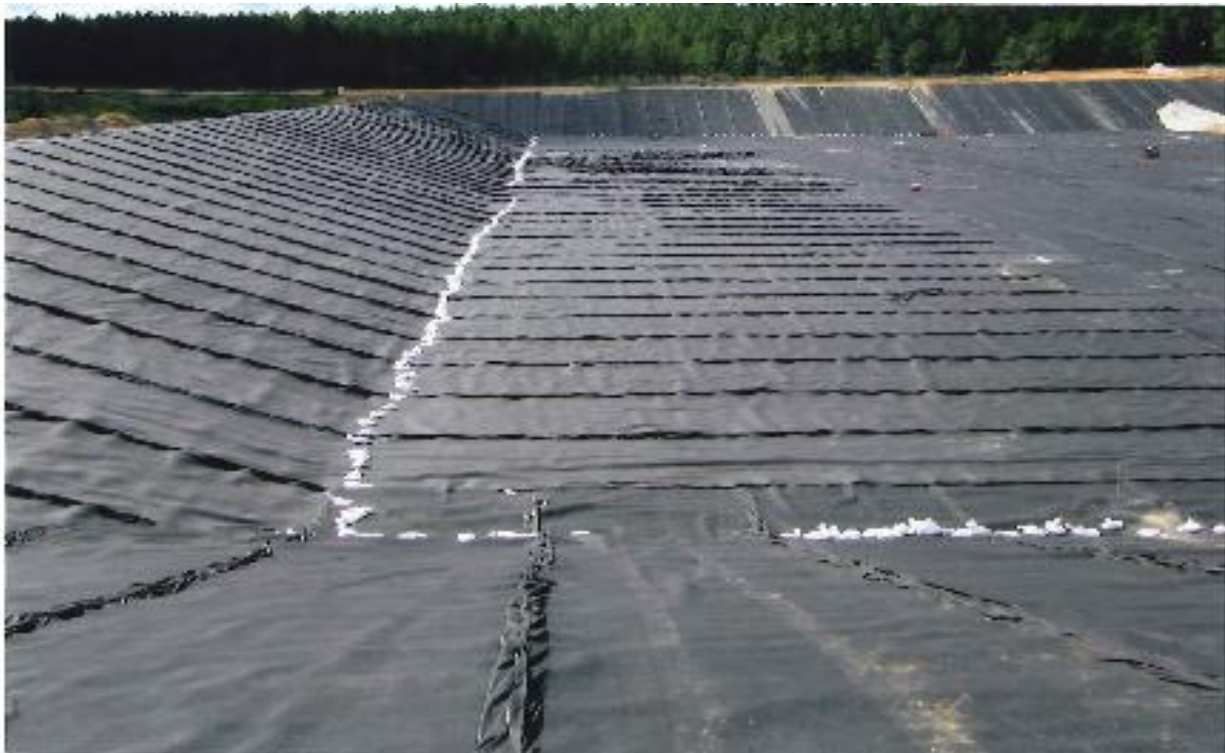
View of Cell-3 with completed geocomposite.
