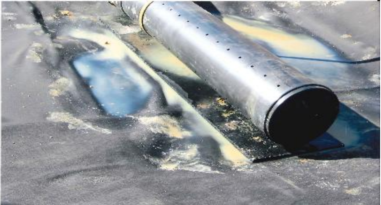
The Cell-3 sump with the 1 inch HDPE plate and sump riser pipe in place.
