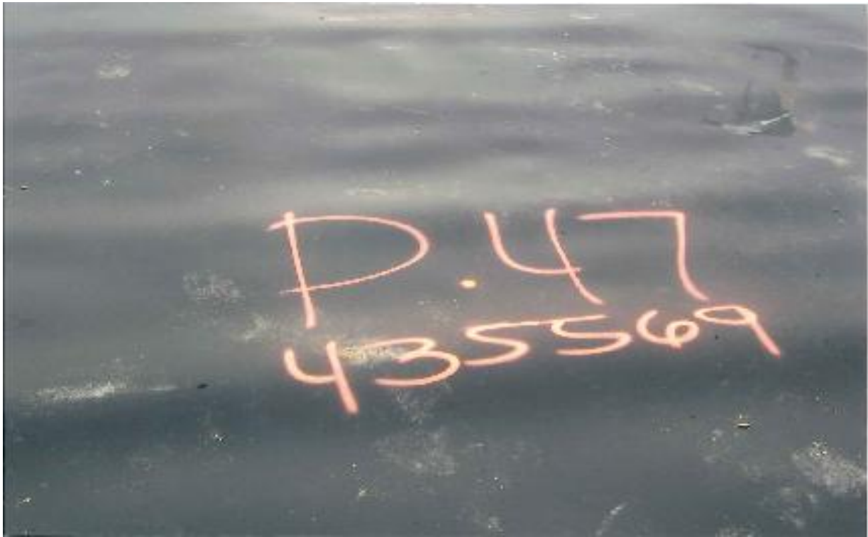
Each panel was numbered and roll numbers were recorded.
