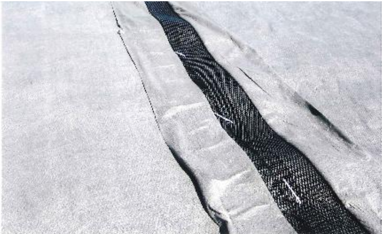
Geocomposite seams were overlapped and plastic ties were used to connect the net.
