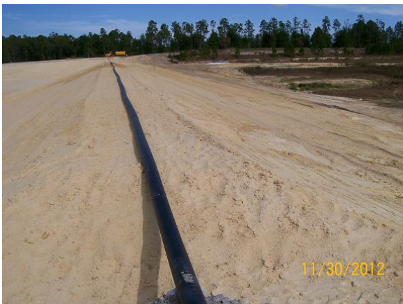
Temporary Header - pic 2
