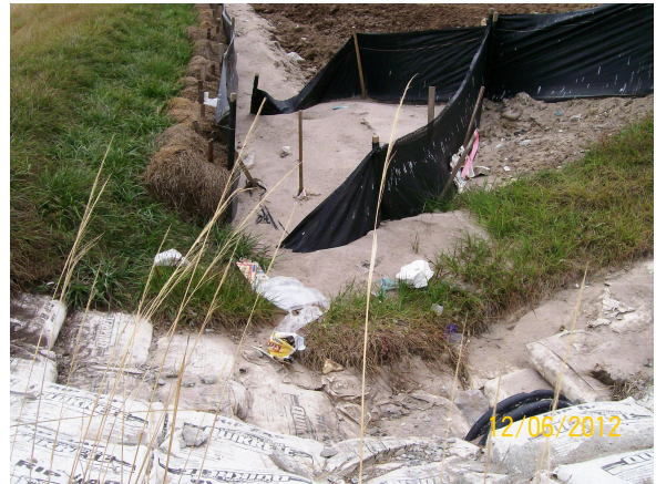
Stormwater pipes clogging
