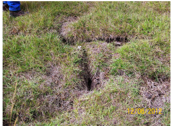
Erosion on Side Slope Units 44-47
