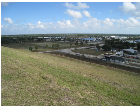
Sideslope showing tack-on berm
