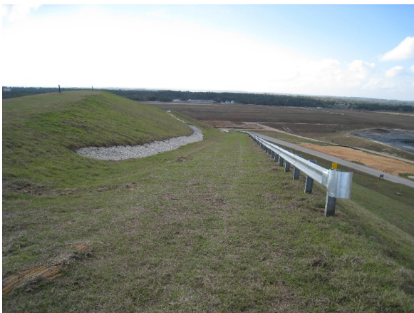
Access Road & Toe Drain
