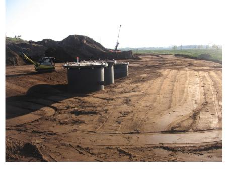
At 3:30 pm G4 complete 12<sup>th</sup> lift finish the dirt face and the area is ready to concrete and electrical work.
