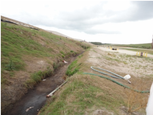
Toe Drain Area
