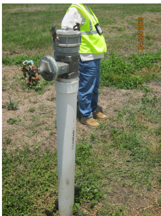
SW-1 stand pipe, since abandoned
