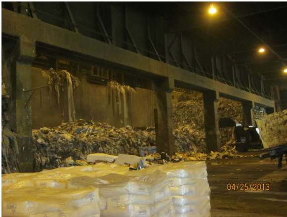
WTE tipping floor
