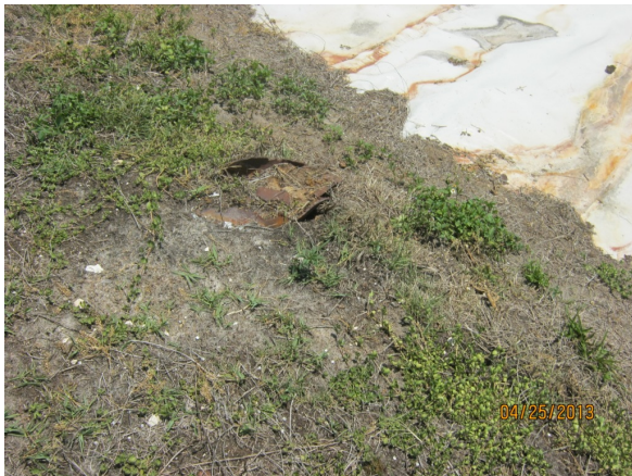
SW-1 exposed waste
