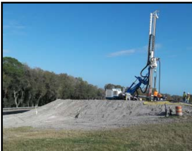
Photograph 3: Typical View of Drilling Operation and Platform
