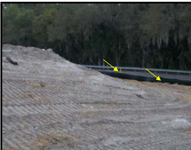
Photograph 6: Silt Fence Around Earthen Work Platform
