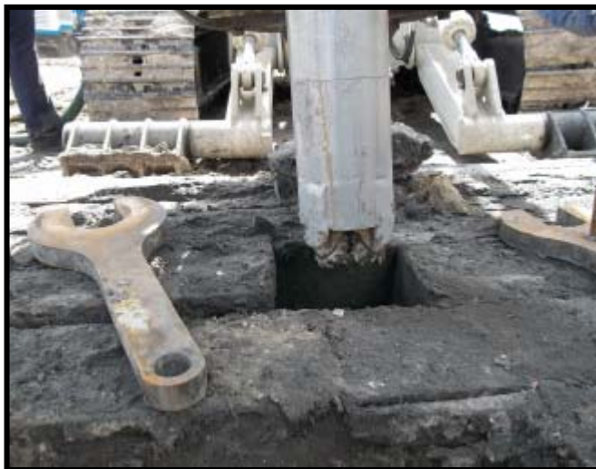
Photograph 14: Typical View of Duplex Bit System
