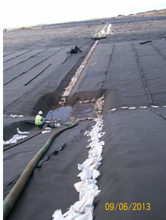
Leachate Corridor - pic 2
