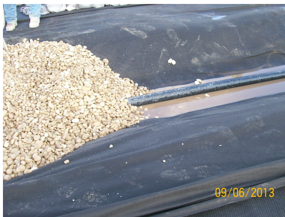
Leachate Corridor - pic 1
