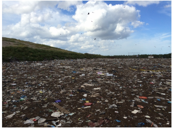
Waste Protruding Through Cover
