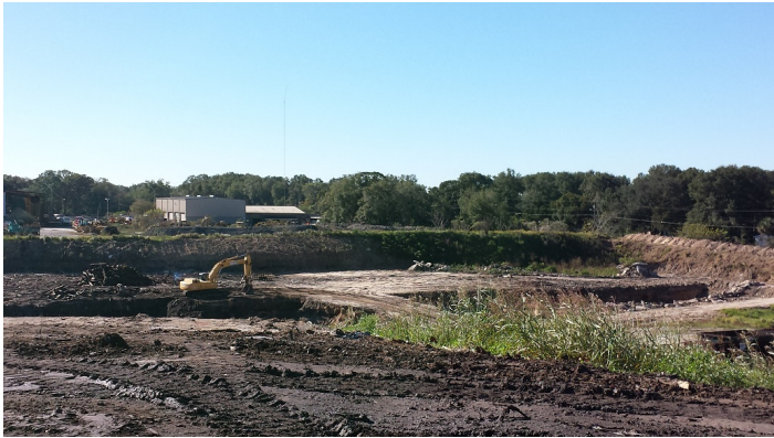
Cell 2B- construction
