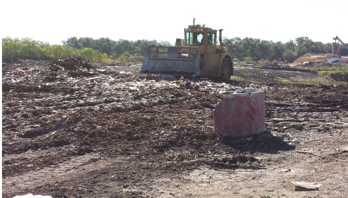
A portion of the working face
