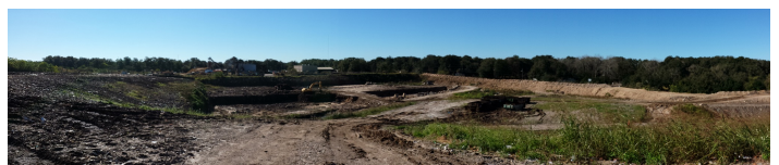
Over view of Cell 2B
