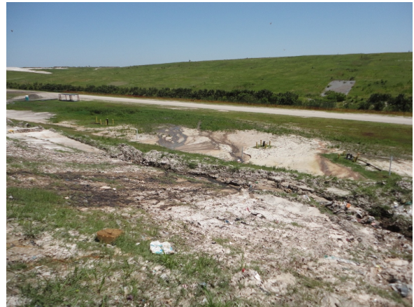
South Side Slope Leachate
