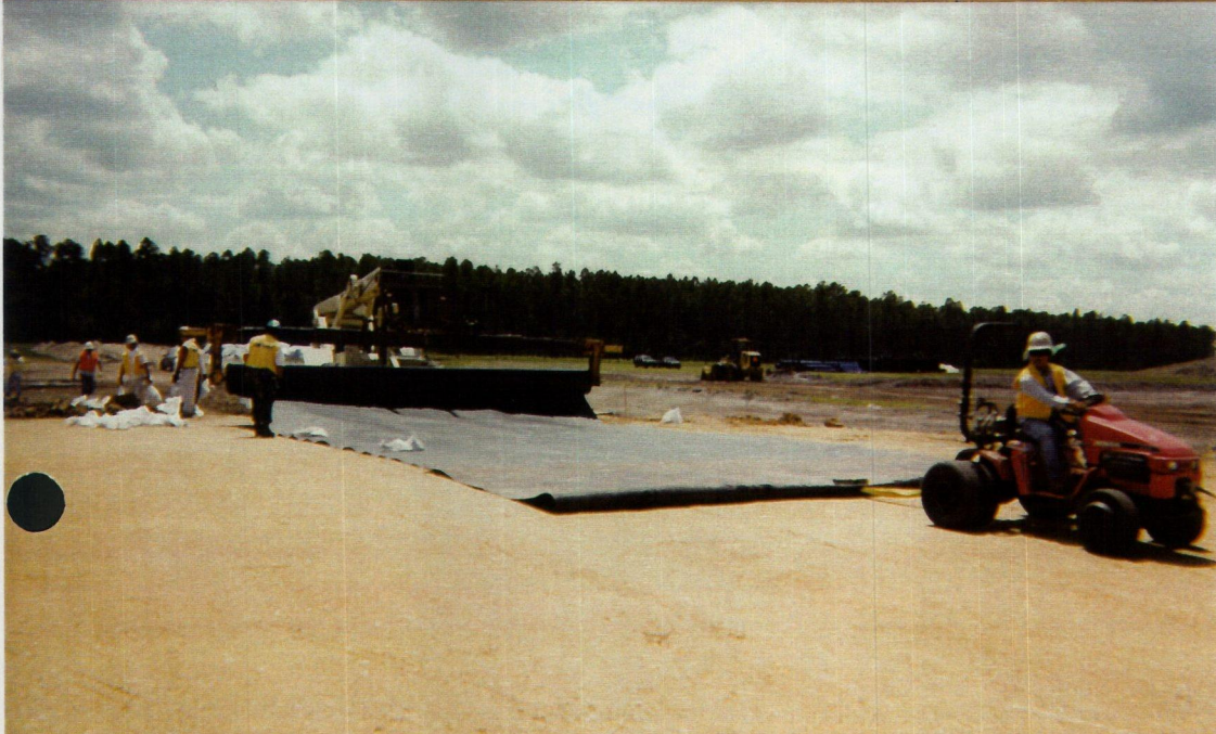
Secondary Geomembrane Liner Placement
