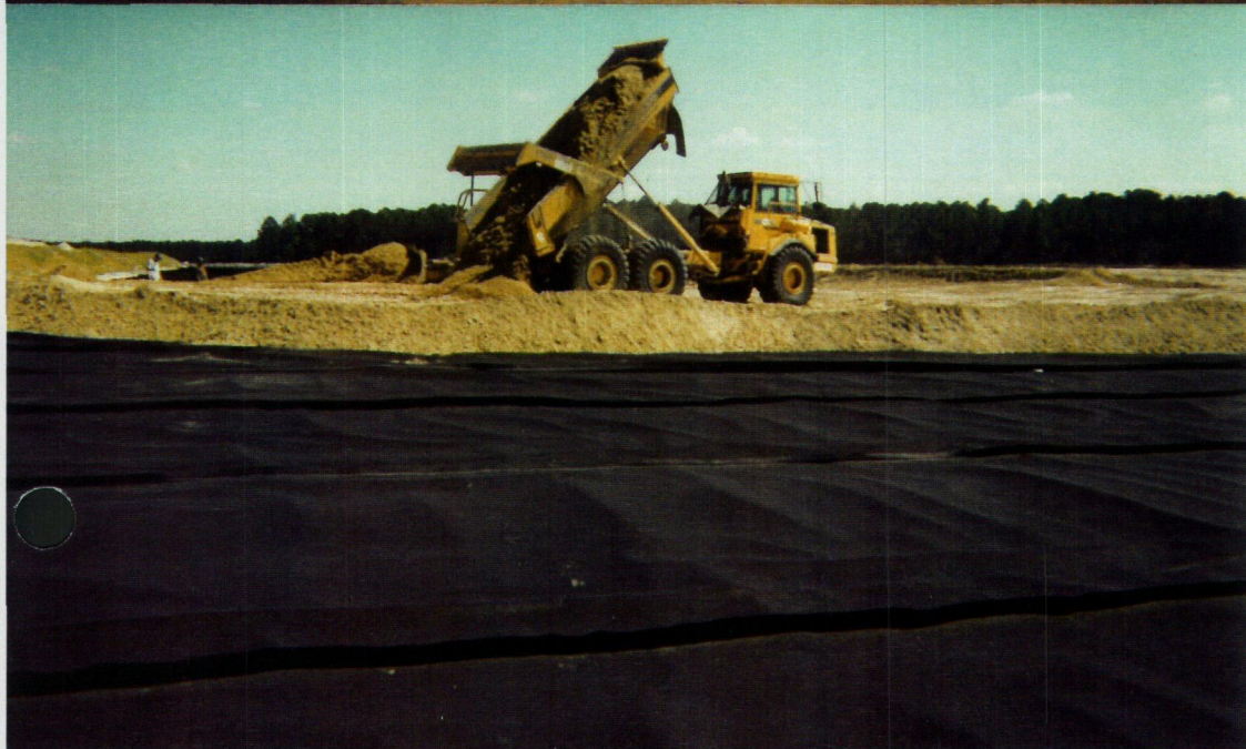
Placement of sand onto the Geosynthetic Liner System
