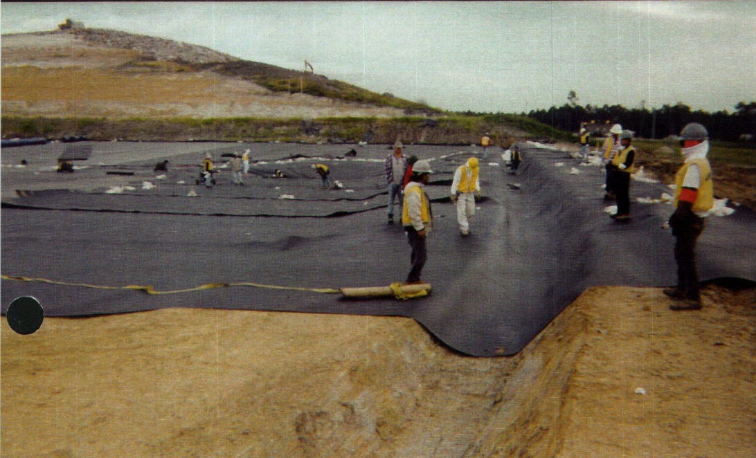
Installation of Secondary Liner in Anchor Trench
