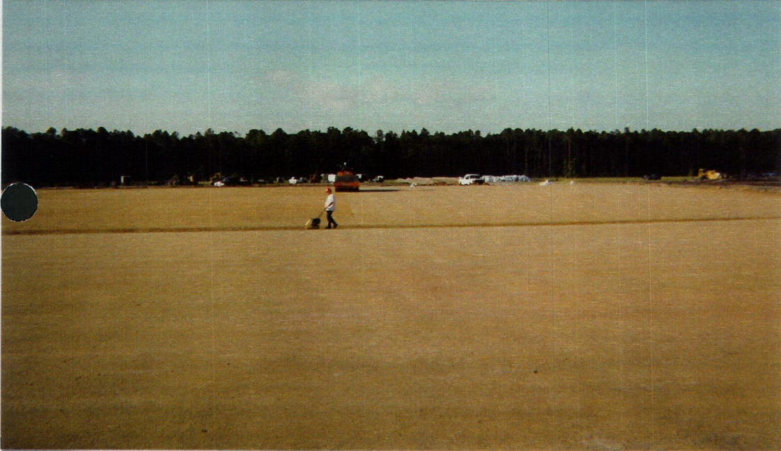
Detailing and Sealing Finished Clay Layer
