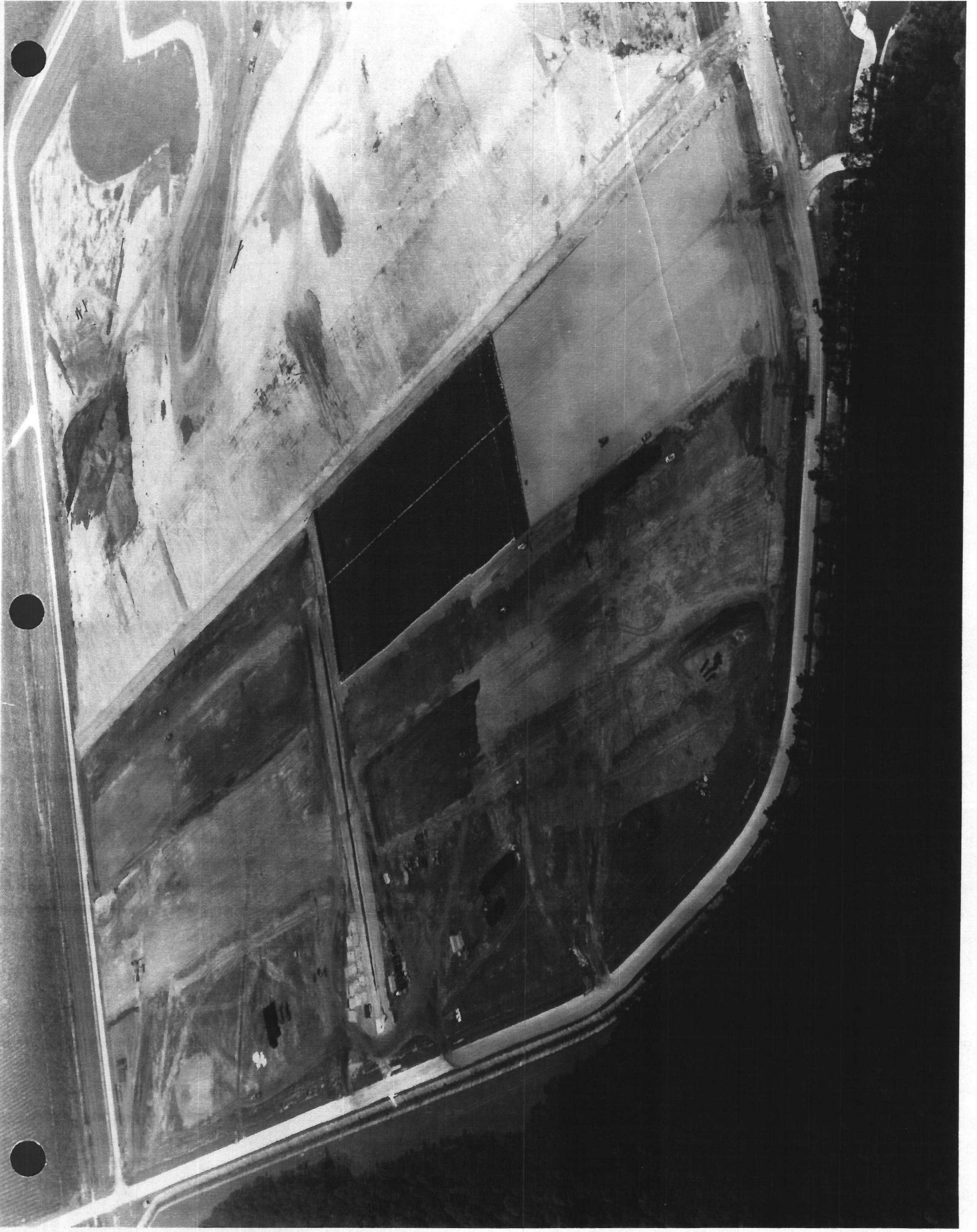
August 28, 2000 - Phase III Construction Site (View looking west)
