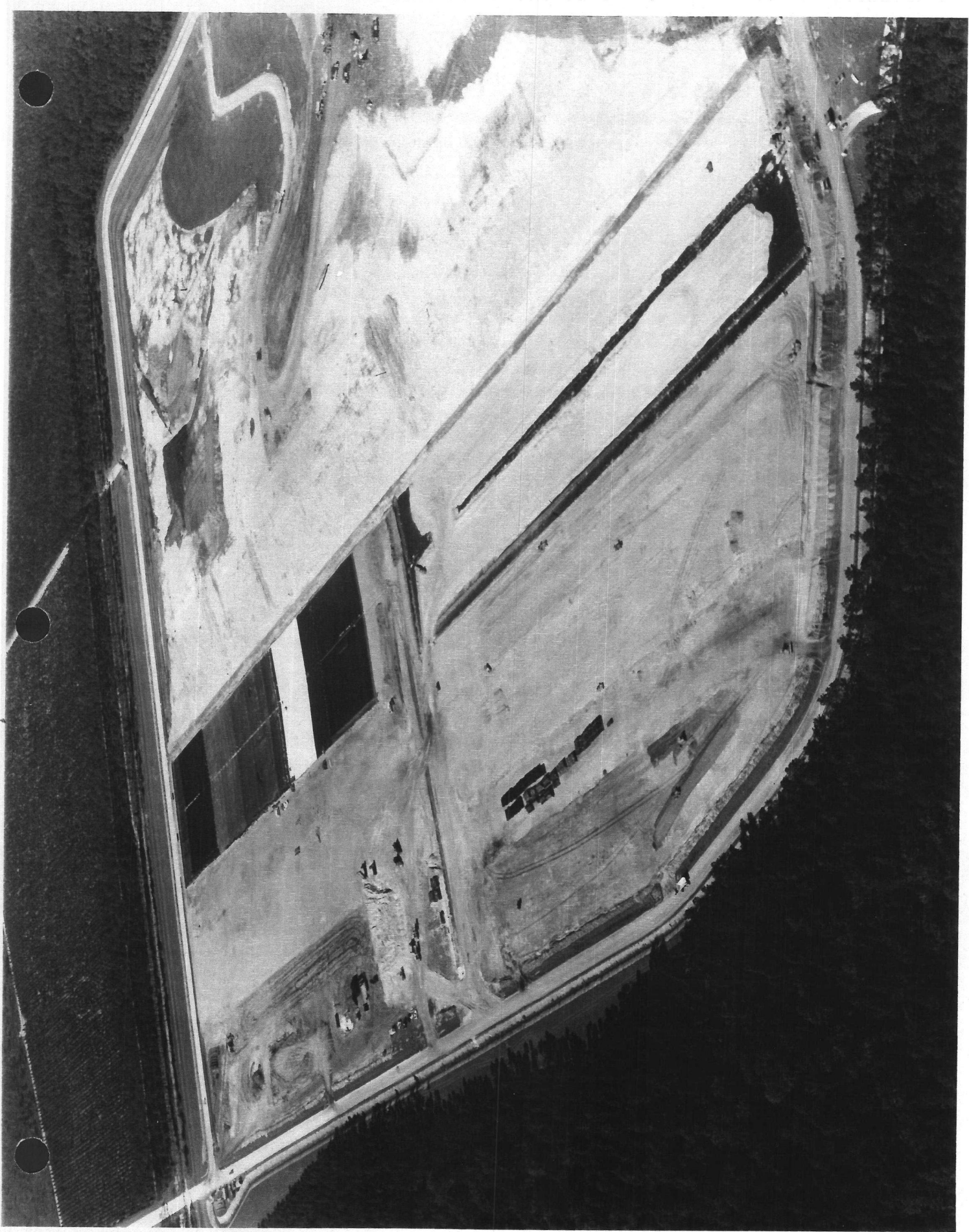
October 27, 2000 - Phase III Construction Site (View looking west)
