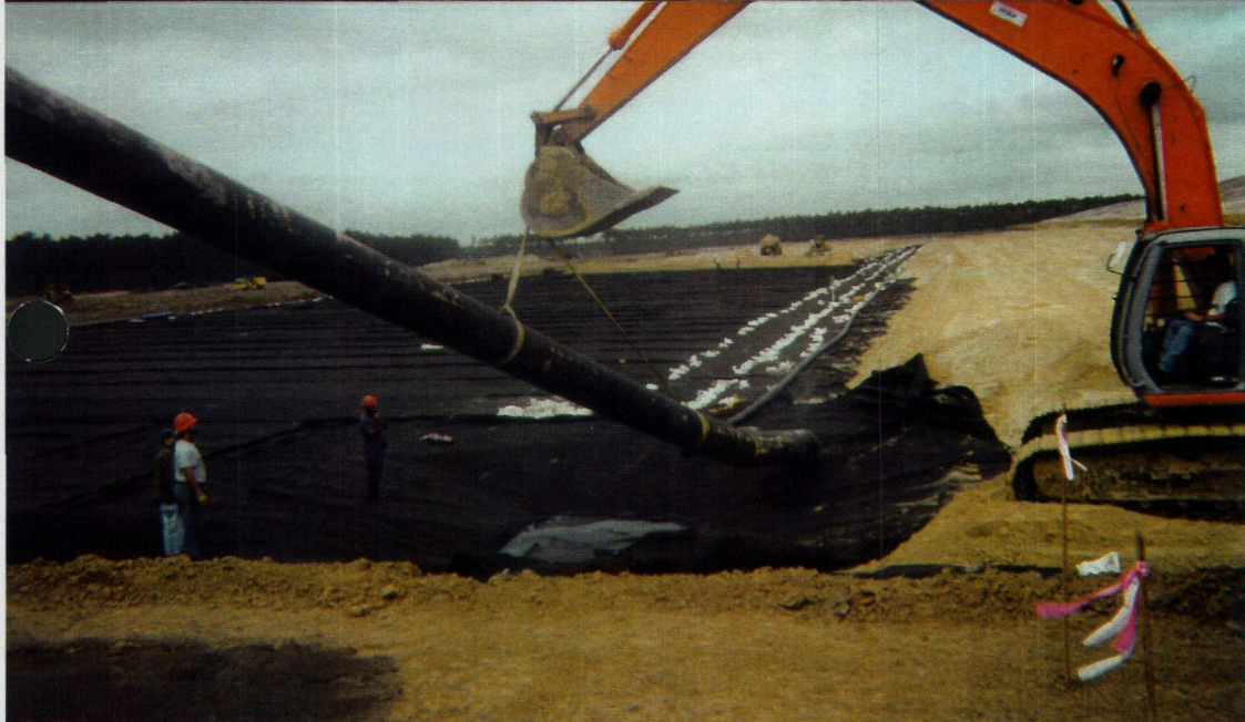
Placement of the Primary Riser Pipe into the Sump
