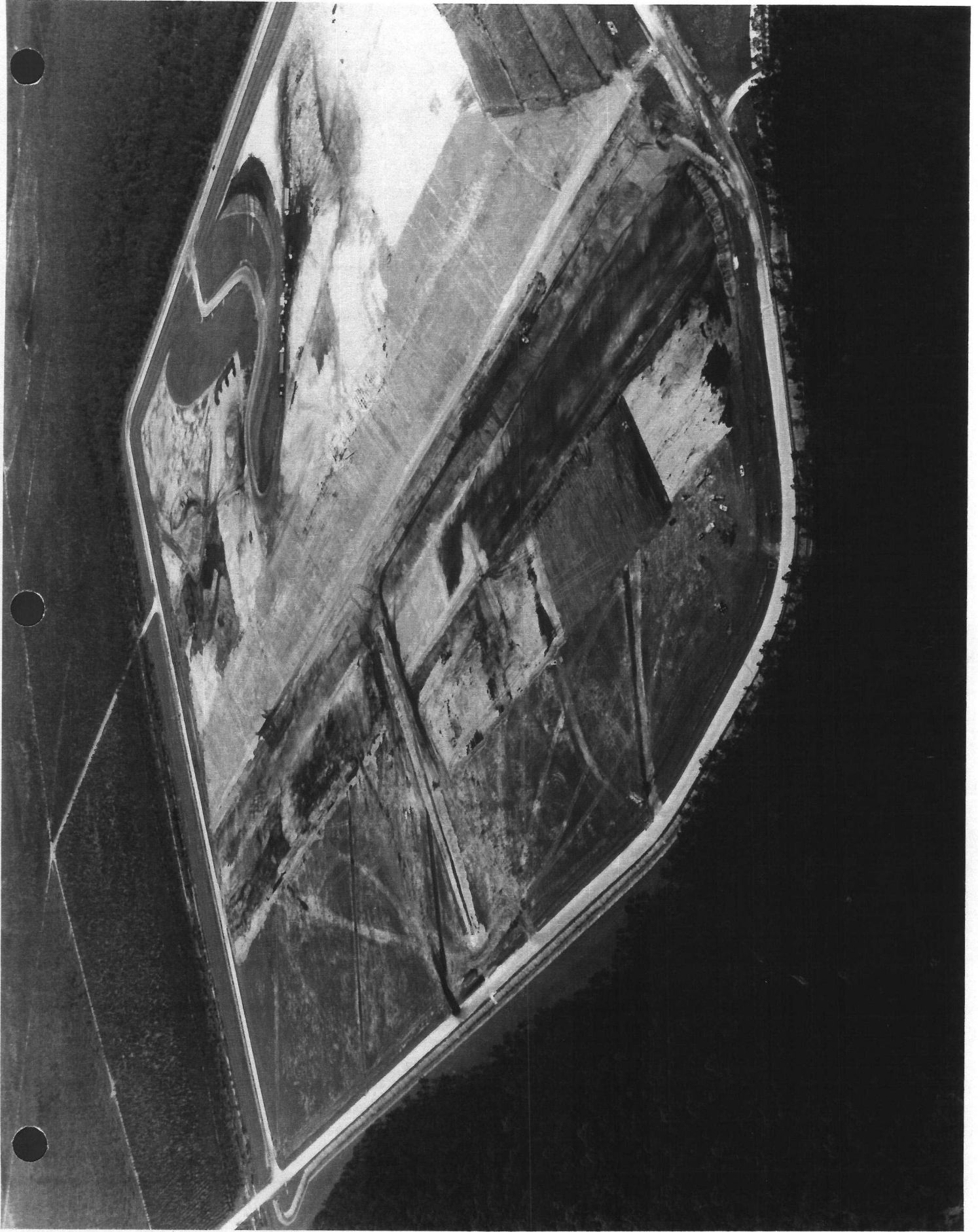
July 26, 2000 - Phase III Construction Site (View looking west)
