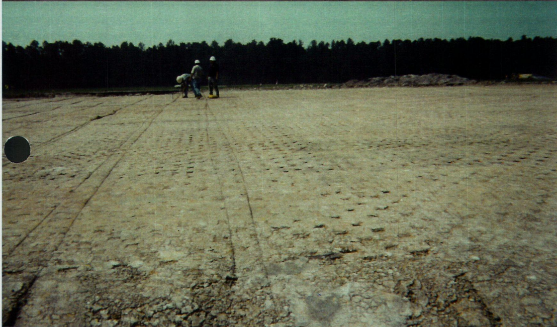
Test Strip after rolling sheep-foot roller prior to final grading
