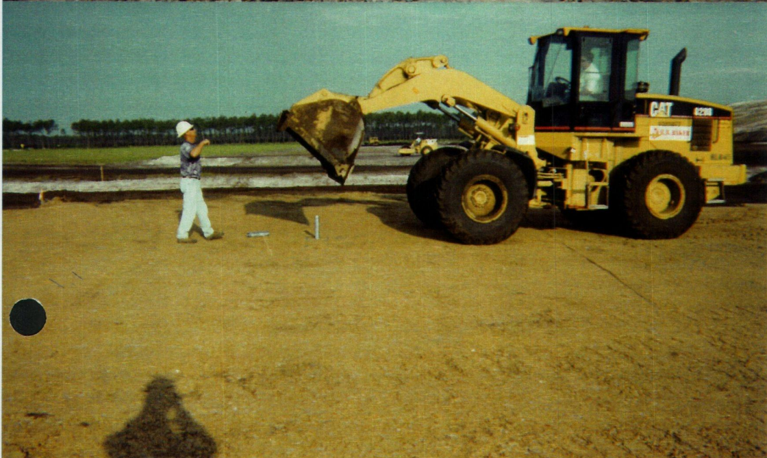
Obtaining samples of Test Strip for Laboratory Testing
