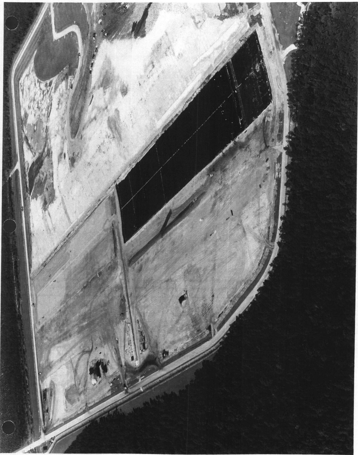
October 2, 2000 - Phase III Construction Site (View looking west)
