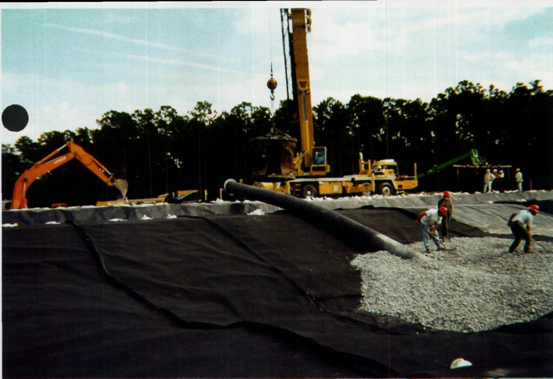
Placement of Aggregate around the Secondary Riser Pipe
