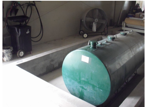
HHW - used oil tank
