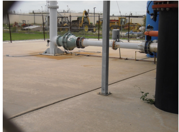
staining @ bottom of flare
