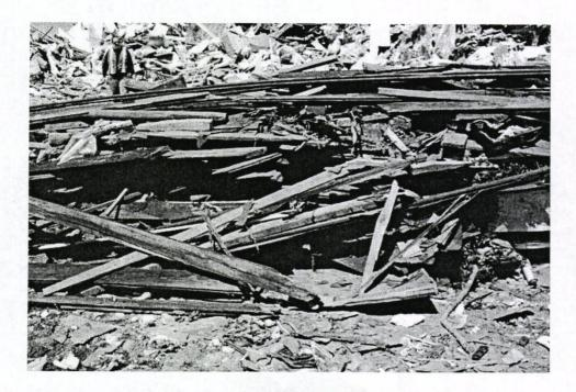
Loads from the demolition of outdoor structures will typically contain CCA-treated wood. Pole at the upper left is treated. Complete recovery of untreated wood from this pile will likely require testing in addition to visual separation.
