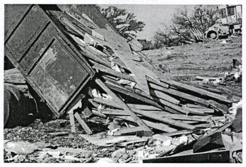
The green colored pole in the front of this pile is treated. Complete recovery of untreated wood from this pile will likely require testing in addition to visual separation.
