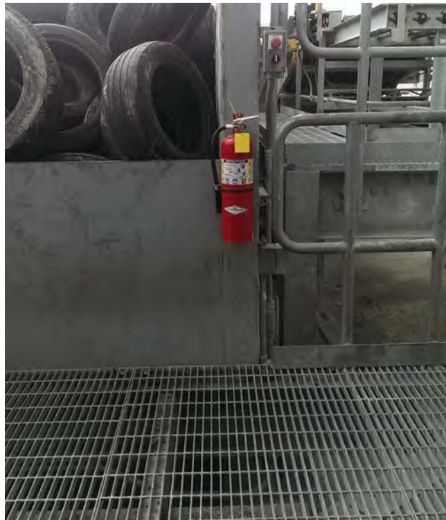
Picture of Fire Extinguisher Installed
