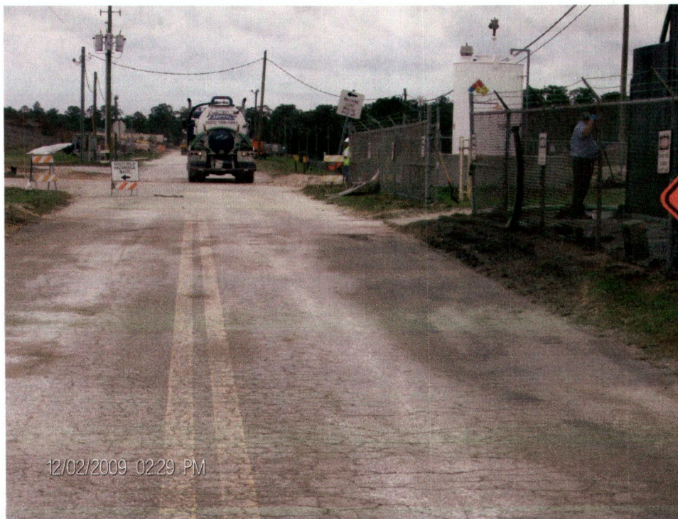
Clean up completed
