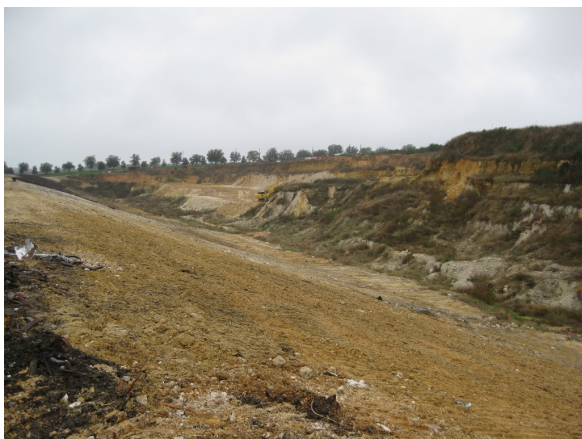
Leachate ditch filled with soil
