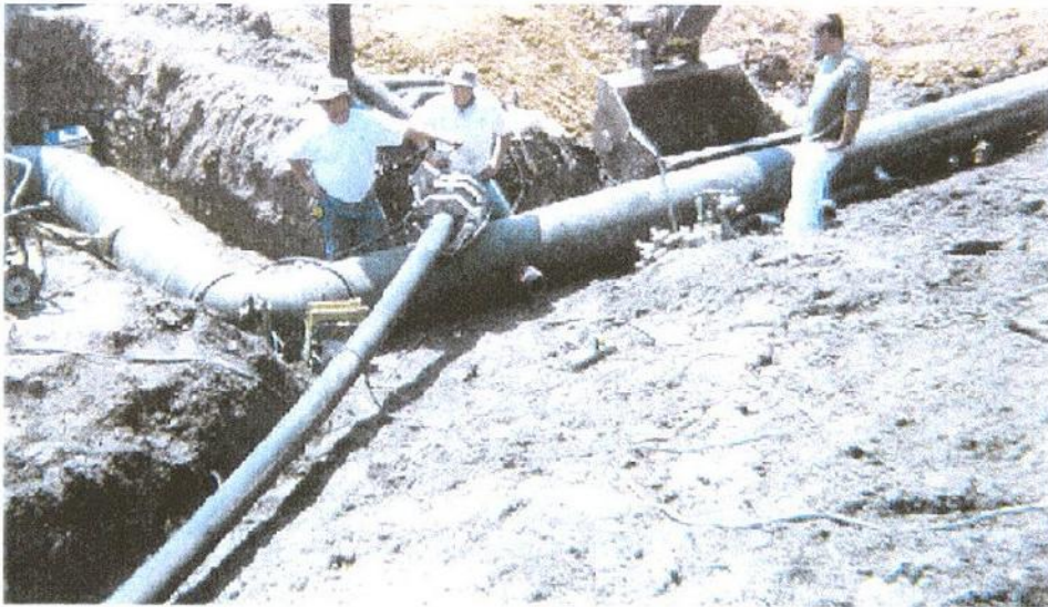
Tie-in of 6 inch header to 22 inch header pipe.
