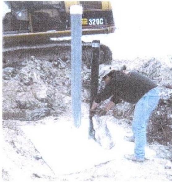
Placement of Bentonite Mat.
