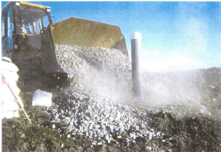
Aggregate placement for Well W-27.
