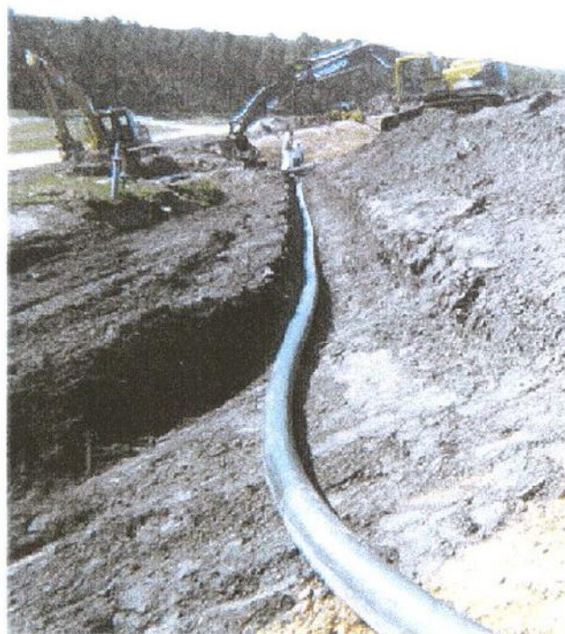
Placement of six inch header line.
