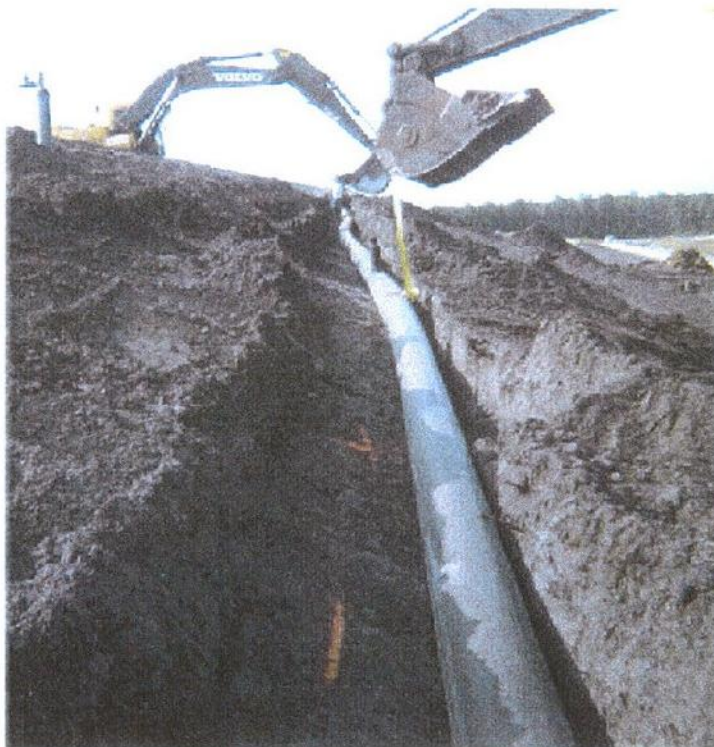
Placement of 22-inch header line.
