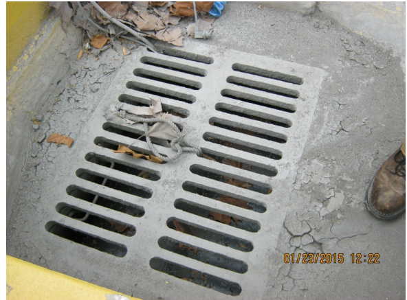
Ash handling runoff drain (fixed)
