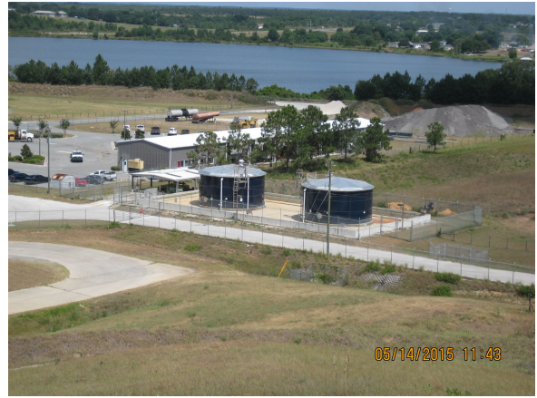
Leachate tanks for class I
