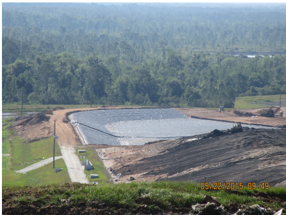
Liner installation Cell 11
