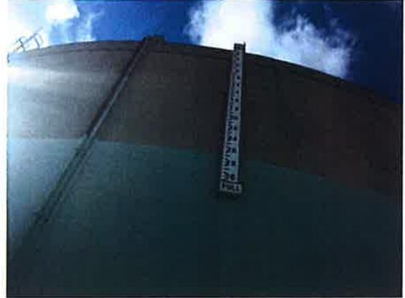
Liquid Level Indicator (LLI) on inner tank
