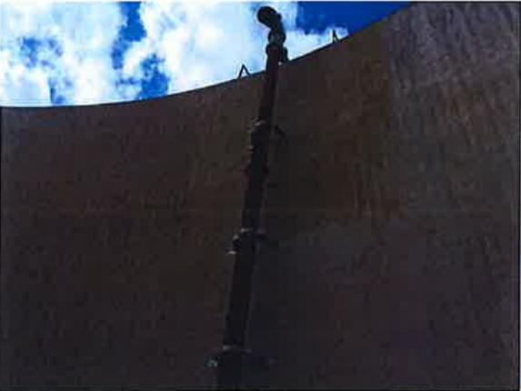
Piping and pipe brackets on inner tank
