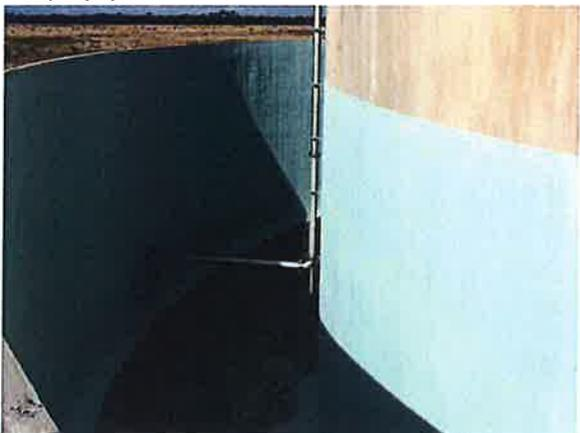
Coatings on interior wall of outer tank
