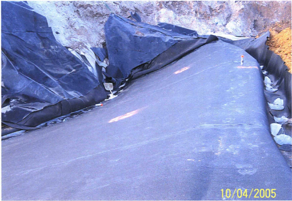
Attachment 7 – Secondary geomembrane tie-in in south west corner with Section 7
