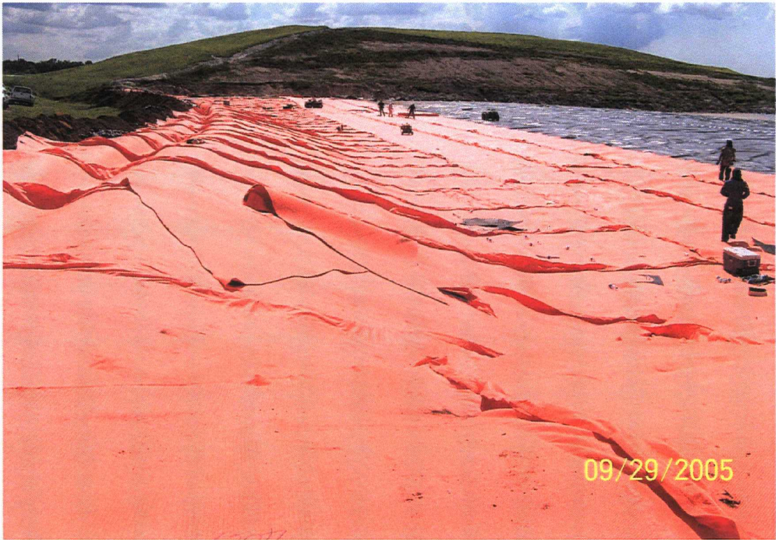
Attachment 7 – Secondary geocomposite deployed
