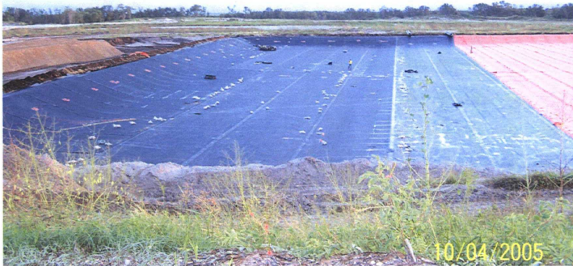
Attachment 7 – Entire secondary geomembrane deployed
