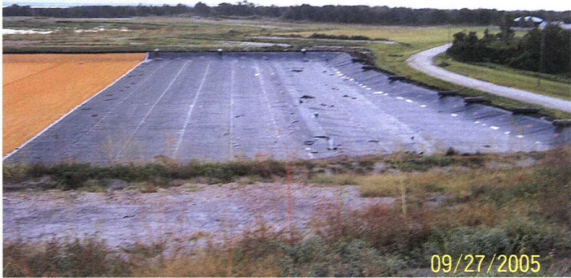
Attachment 7 – Secondary geomembrane deployed
