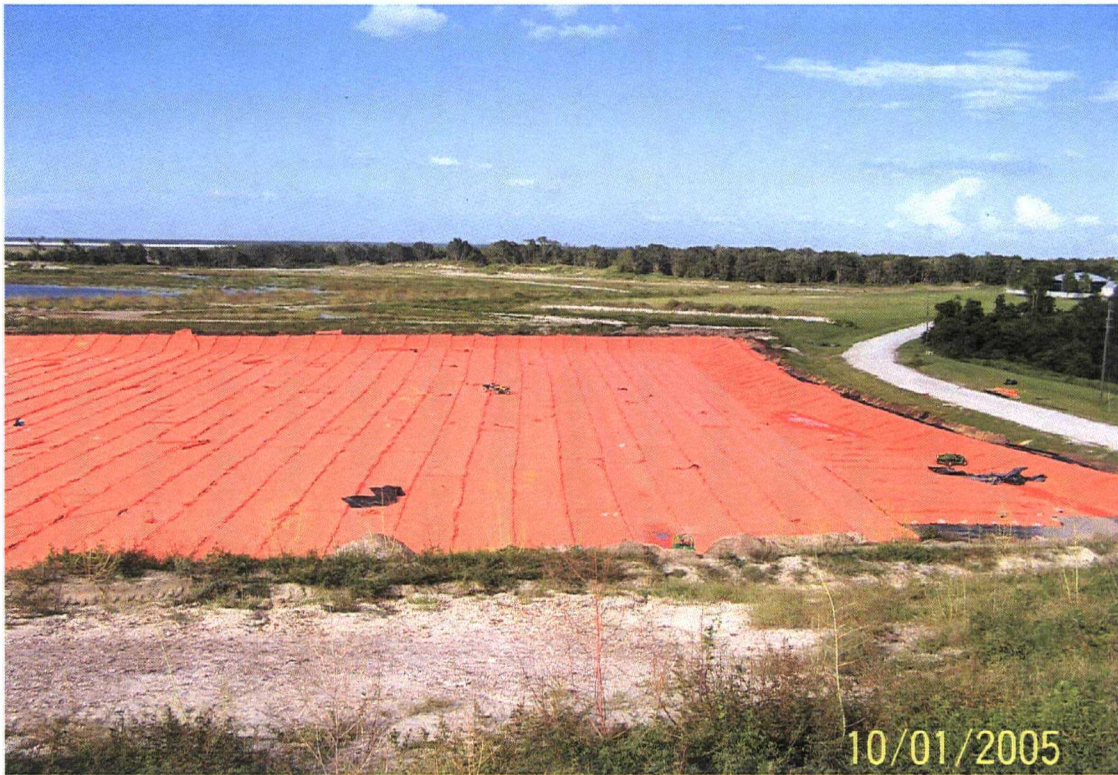
Attachment 7 – Secondary geocomposite deployed
