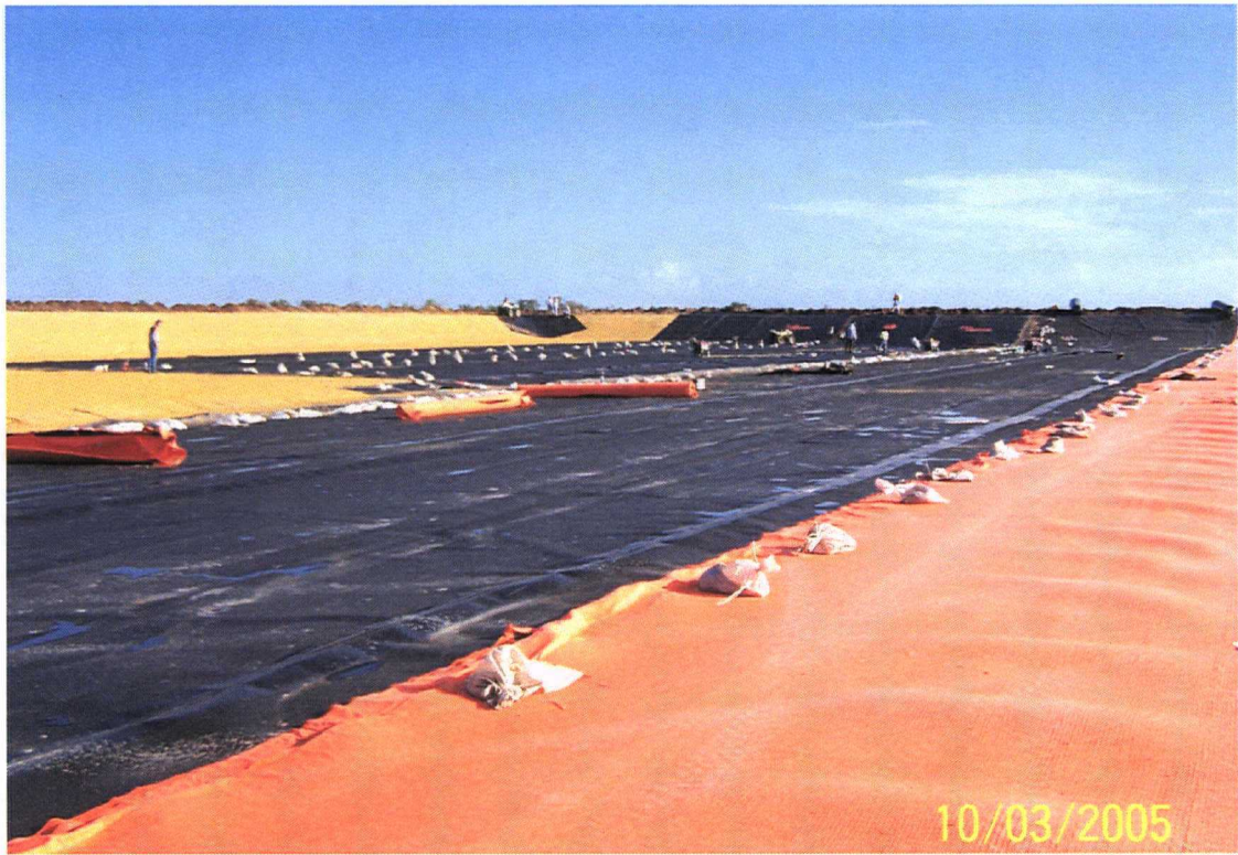
Attachment 7 – Geomembrane deployed on west side of Section 8
