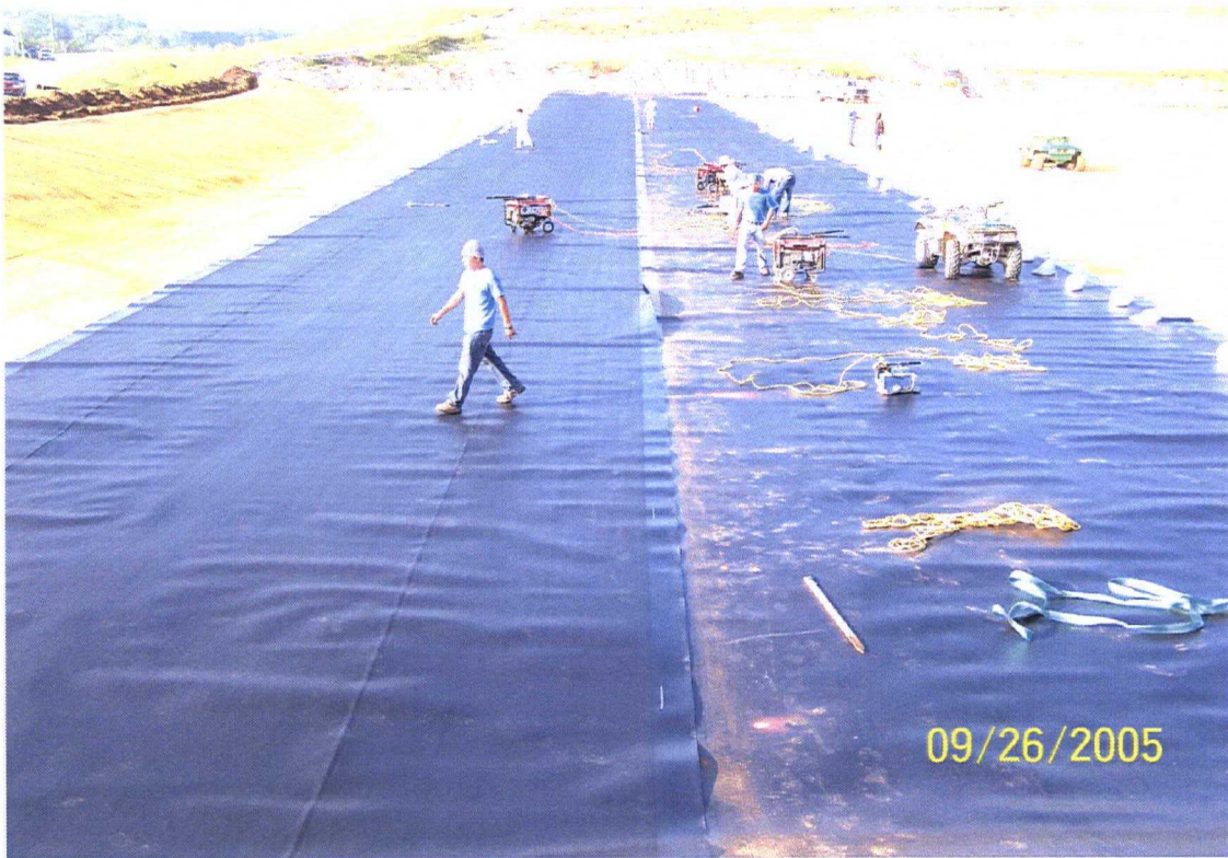
Attachment 7 – Secondary geomembrane deployment. Panels 1 and 27 shown
