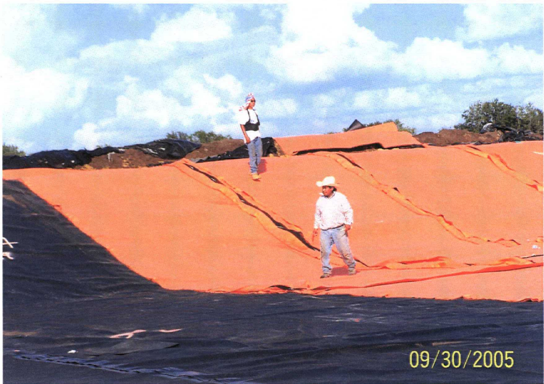
Attachment 7 – Secondary geocomposite deployed
