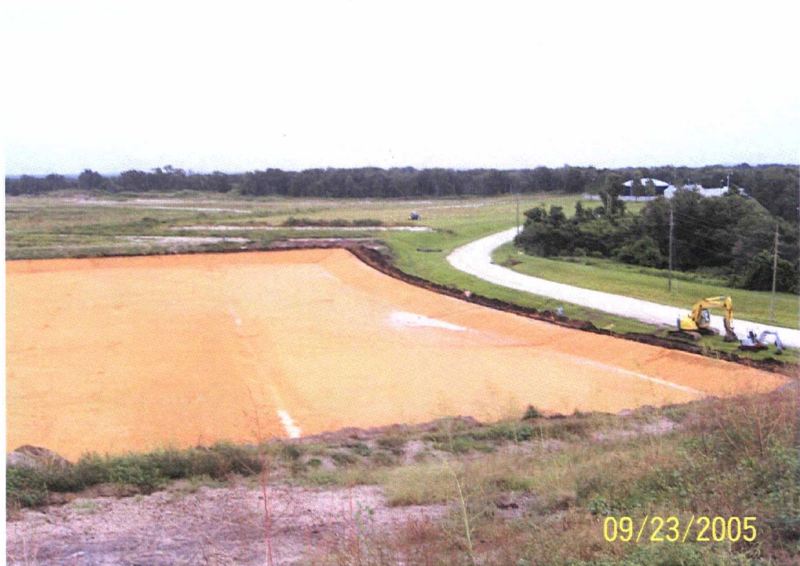
Attachment 7 – Subgrade prepared but rain delayed geomembrane deployment
