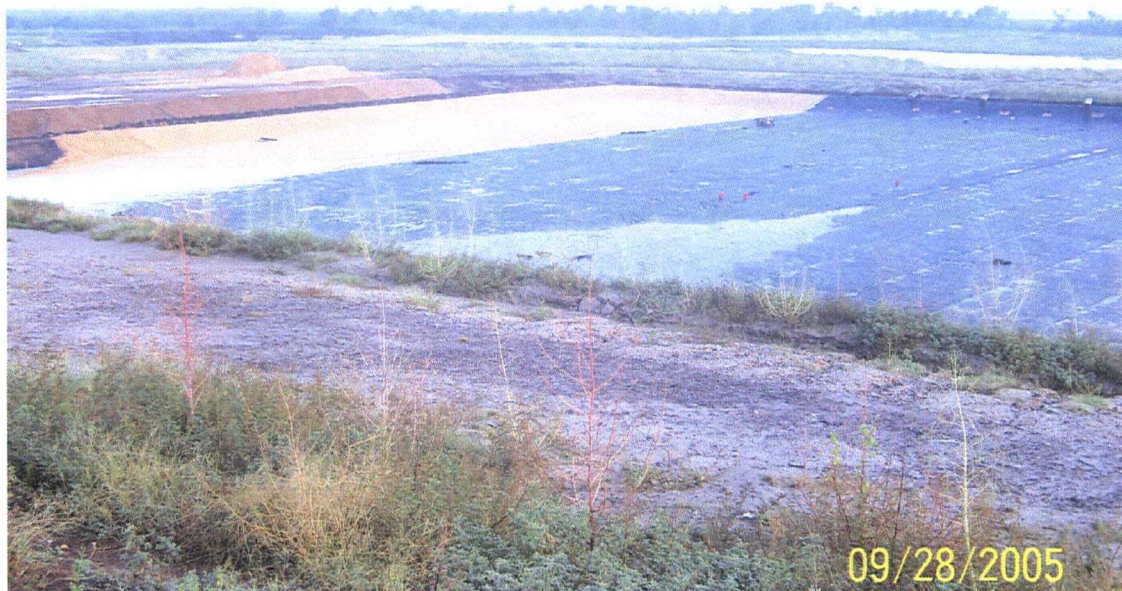
Attachment 7 – Secondary geomembrane deployed. Project delayed due to rain
