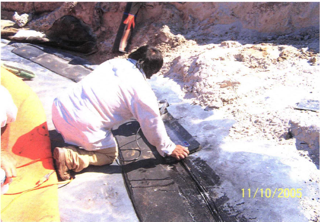
Attachment 2 – Vacuum box of repairs
