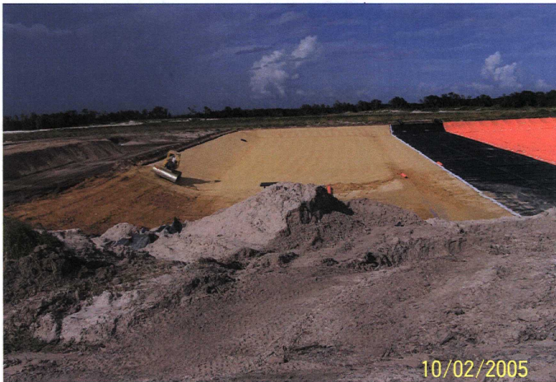
Attachment 7 – Subgrade reworked prior to geomembrane deployed
