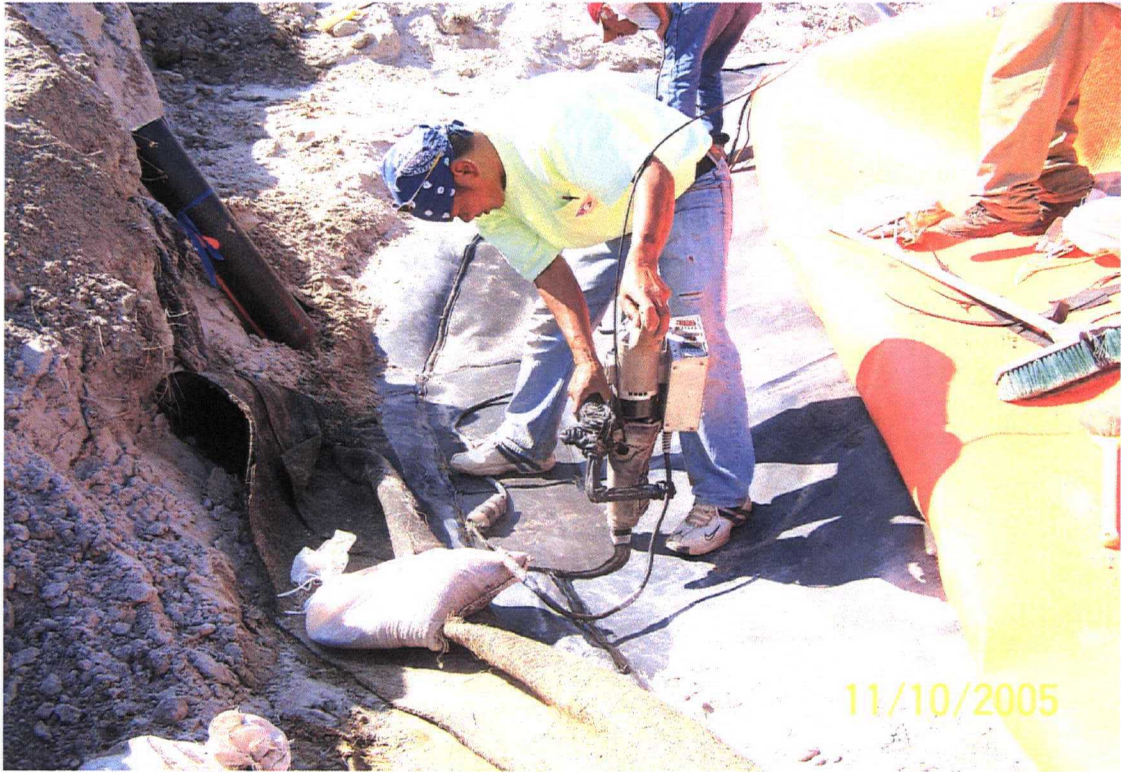
Attachment 2 – Repair of “Blow-out”
