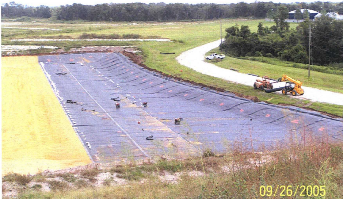
Attachment 7 – Secondary geomembrane deployment. East sideslope installed
