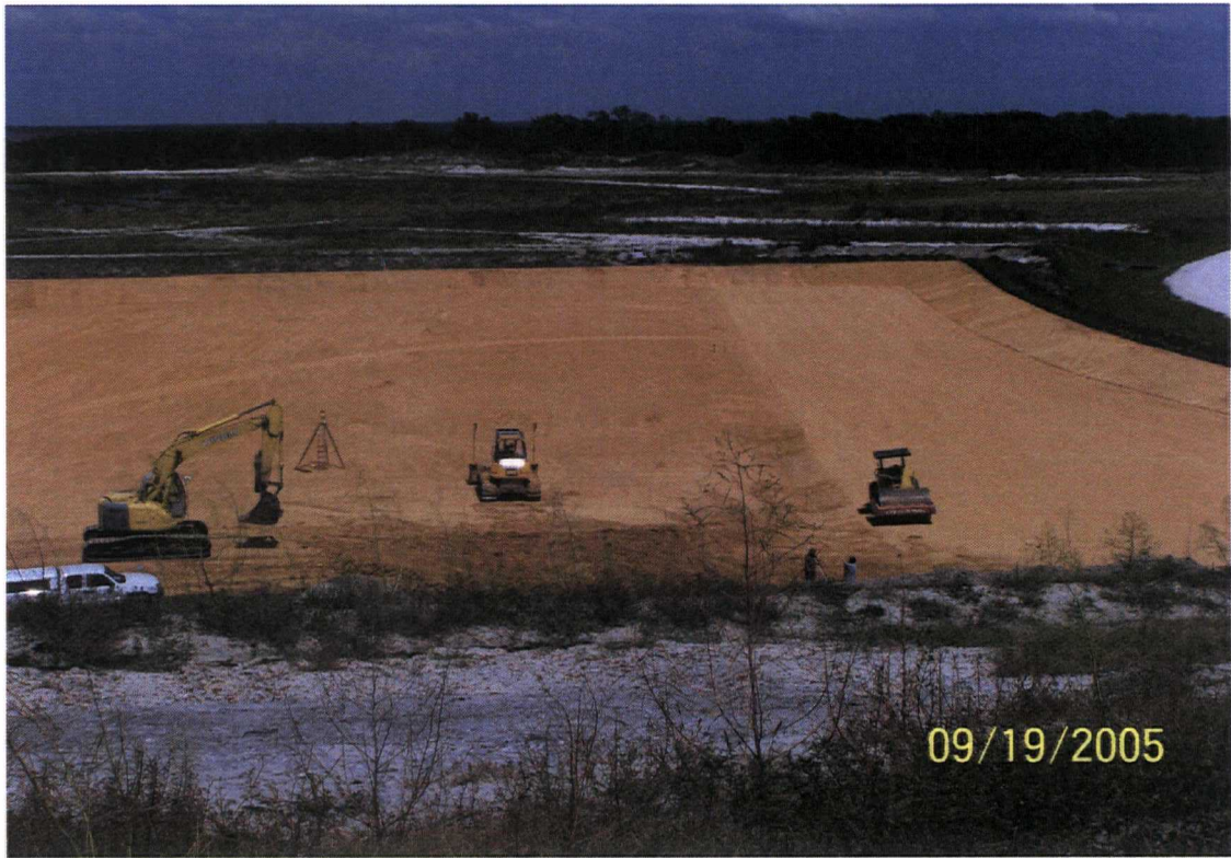
Attachment 7 – Preparation of subgrade
