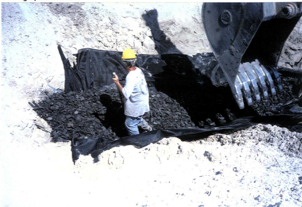
Date: May 17, 1999 Site: Southeast County Landfill, Hillsborough County, FL Description: Phase VI internal berm chipped tire Trench No. 12 (looking east).
