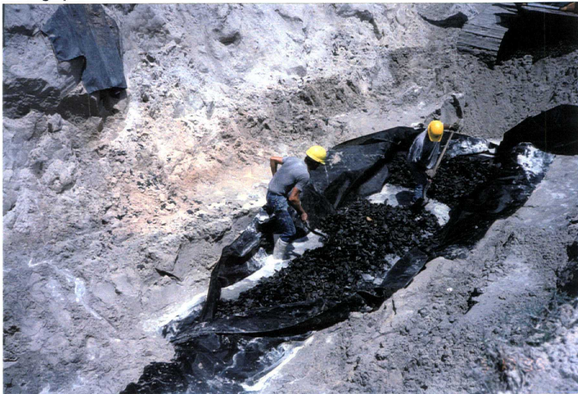
Date: May 17, 1999 Site: Southeast County Landfill, Hillsborough County, FL Description: Phase VI internal berm chipped tire Trench No. 13 (looking west).
