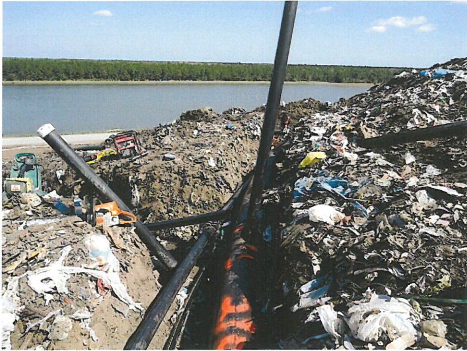
Lateral Connection from EW-8 to New Header
