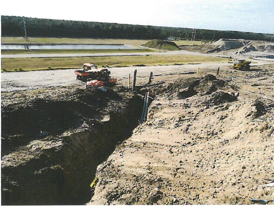
Running New Lateral Lines from EW-12A to EW-6
