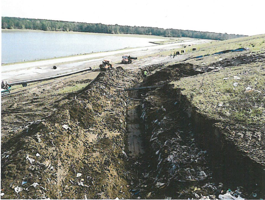
Trench for new 16" Header on North Slope
