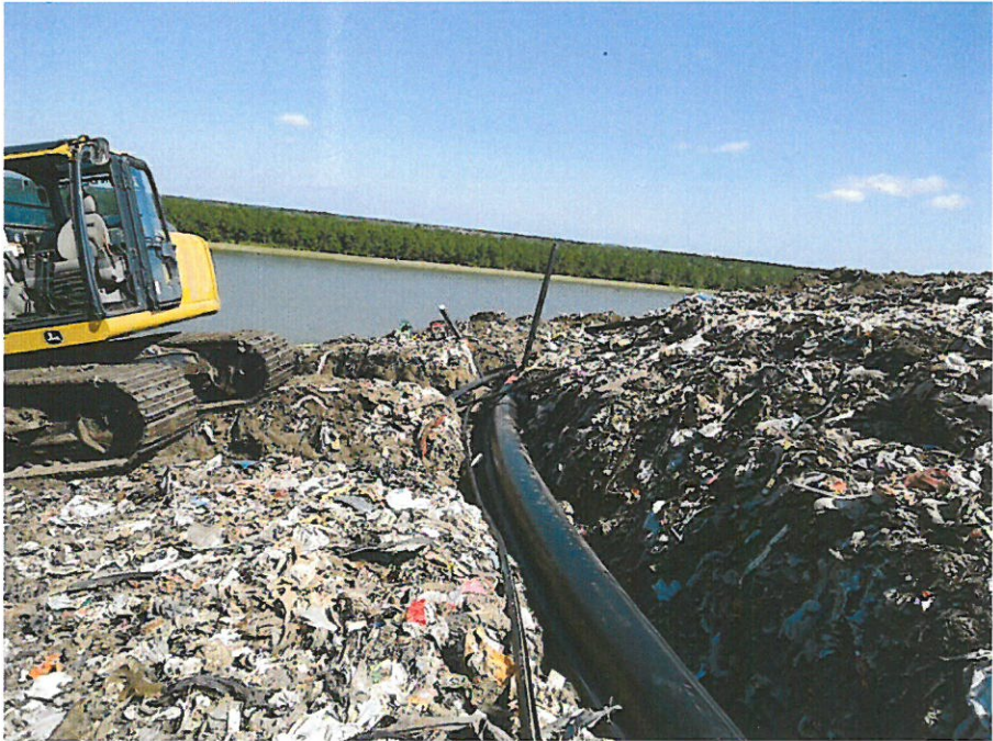
Lateral Connection from EW-8 to New Header
