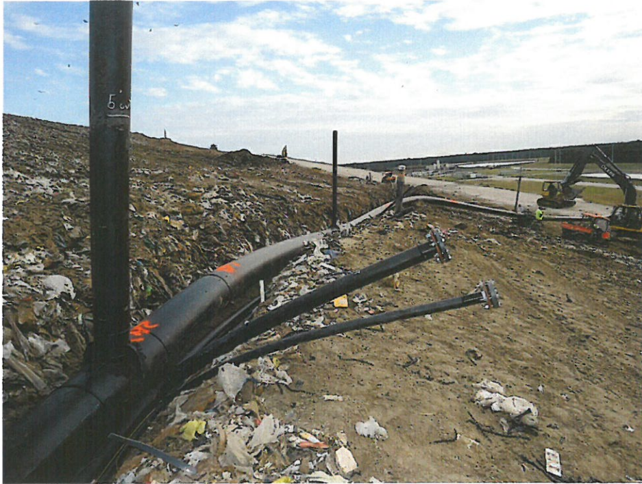
Access Point at High Point of New Header
