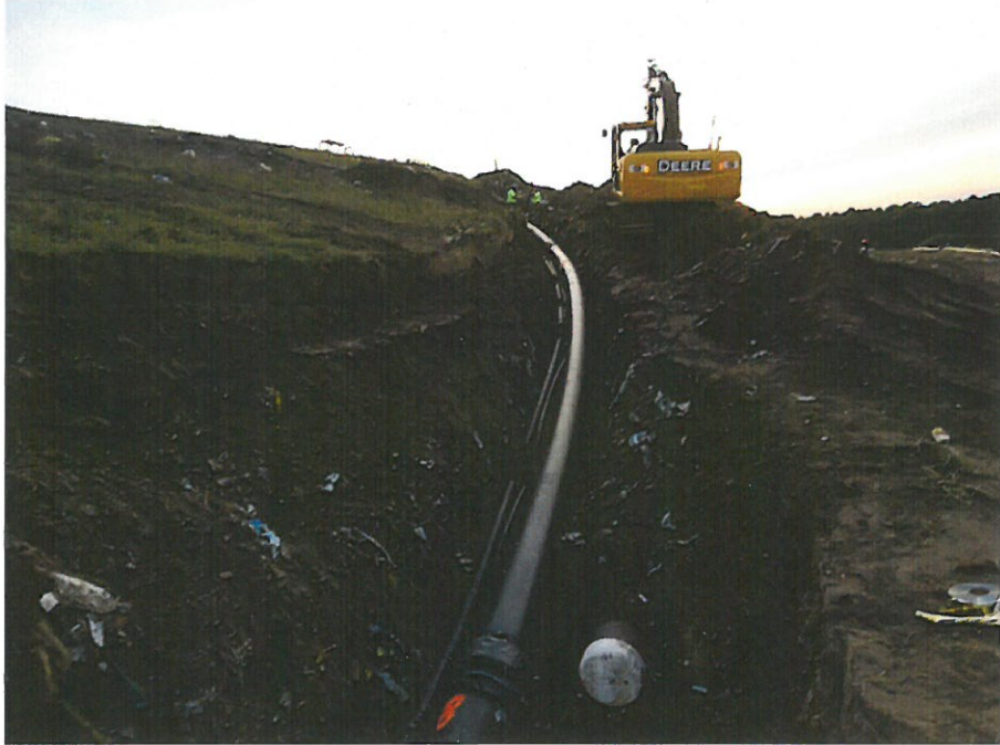
Installing New Header on North Slope
