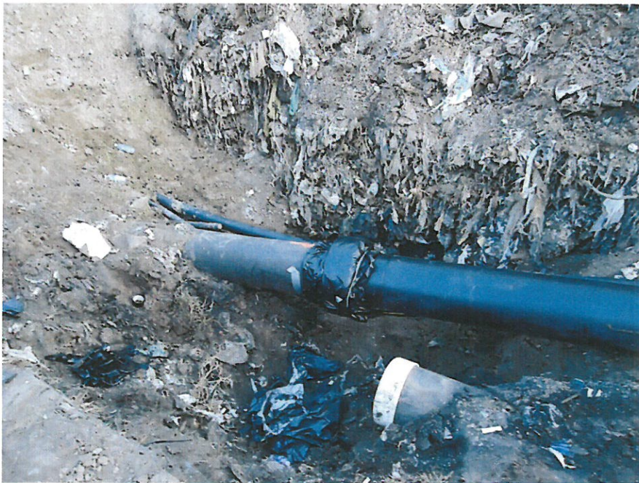
Header Tie-In on North Slope with Existing Header Abandoned
