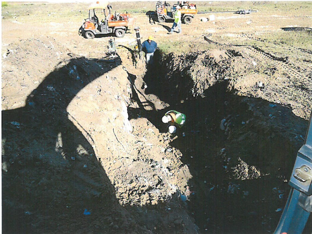
Converting to Existing Well to Remote Wellhead
