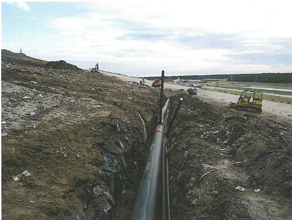
New Header Installation Along South Slope
