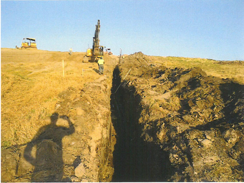
New Lateral Piping from EW-5 to Existing Header
