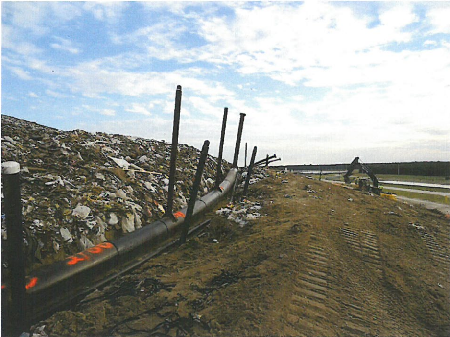
New Remote Wellheads on New Header
