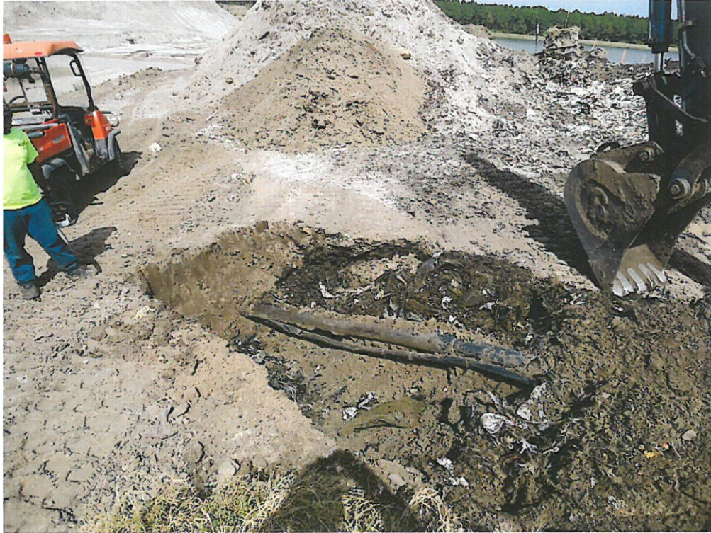
Expose existing lateral connection on West Slope
