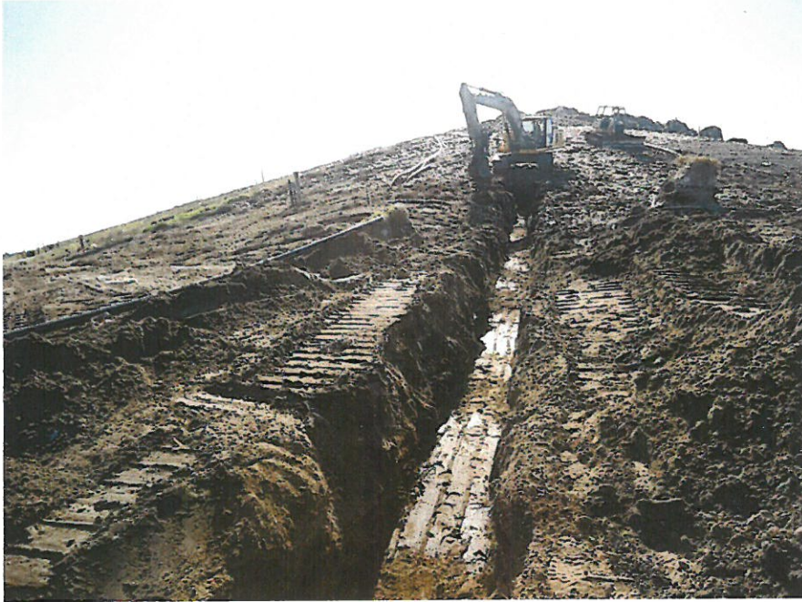
Trenching for New Lateral Lines
