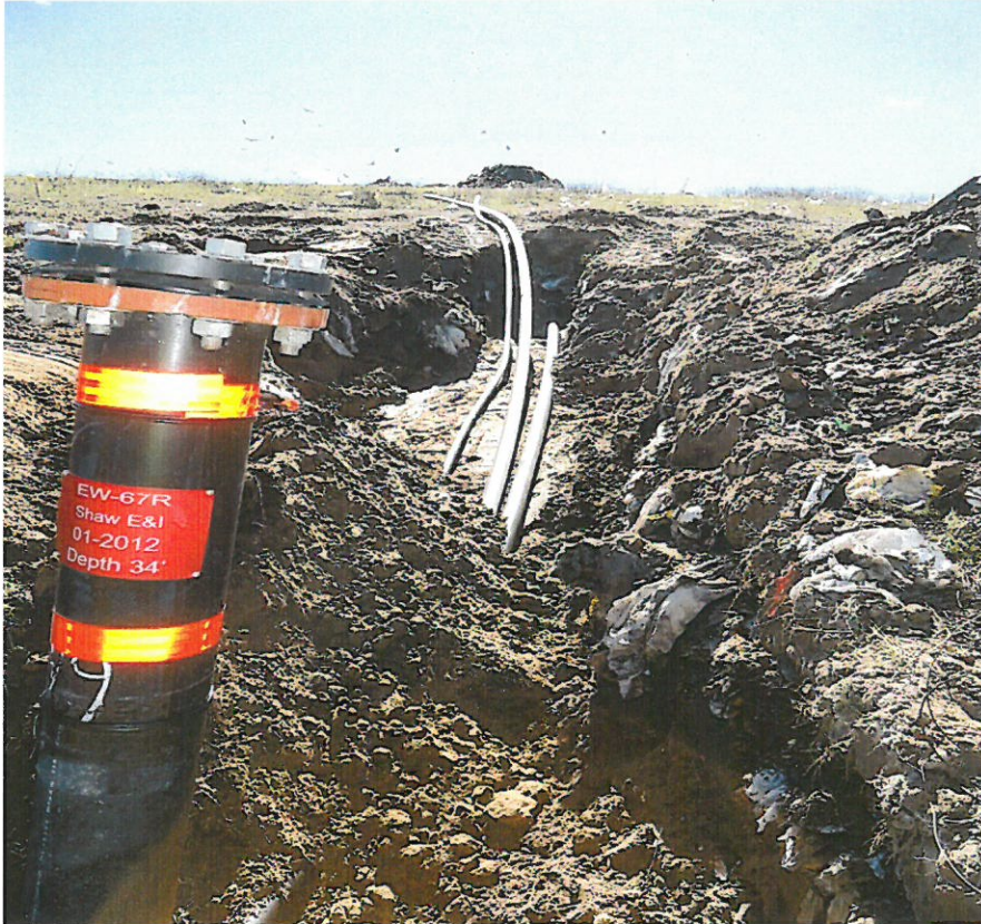
New Lateral lines from EW-67R
