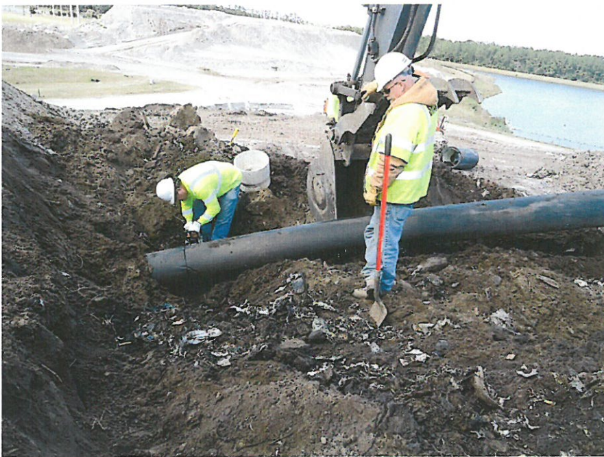
Installing new 16" Header Line
