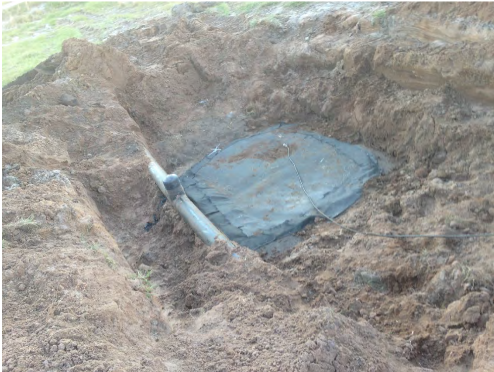
Photograph 66: Abandoned well geocomposite repair in progress (typical).
