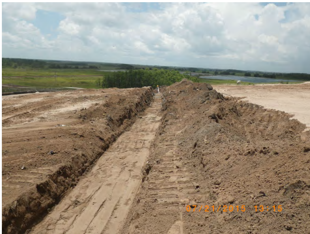
Photograph 12: Standard trench for lateral (typical).
