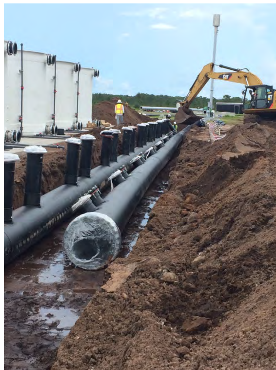
Photograph 32: Installing 30" "Treated Gas" Header.
