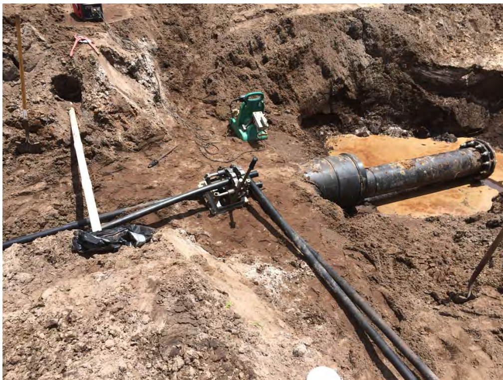
Photograph 38: Welding 2" air and 2" forcemain.
