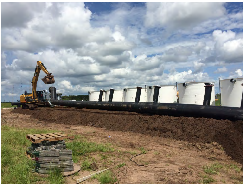
Photograph 31: Installing 30" "Untreated Gas" Header.
