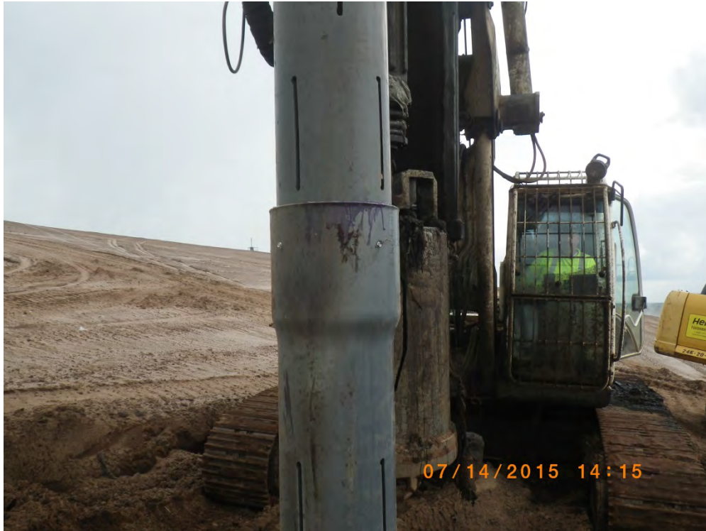
Photograph 7: Lag bolted joints to provide additional support (typical).
