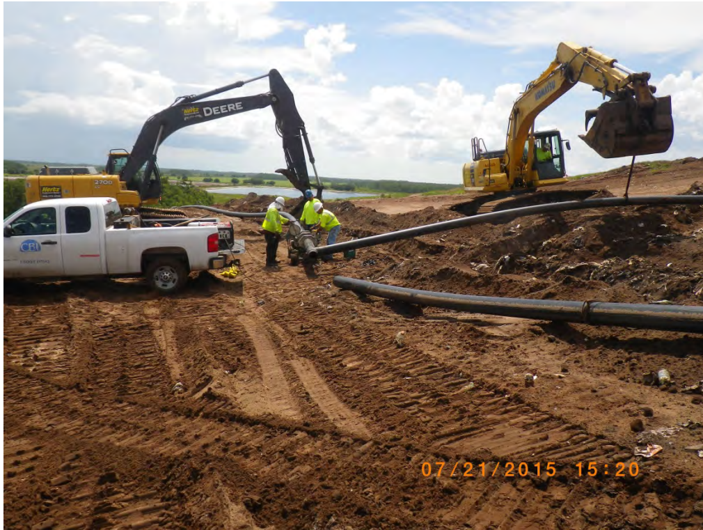
Photograph 13: Welding HDPE lateral piping (typical).
