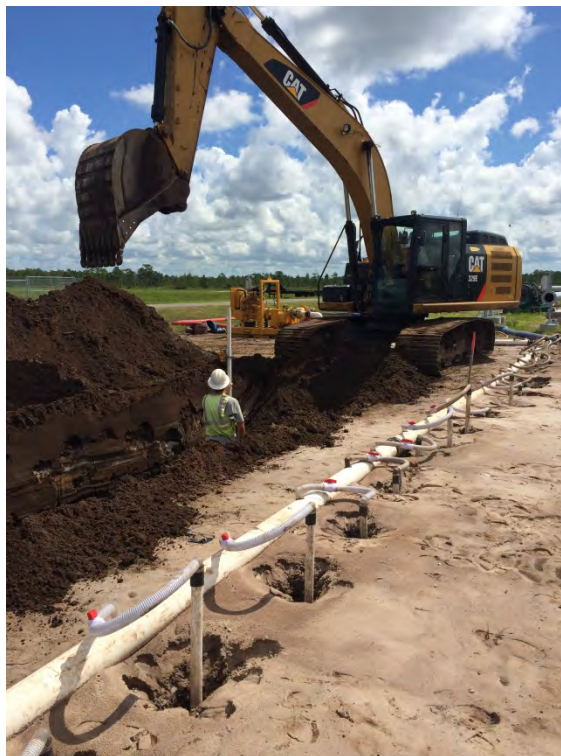
Photograph 30: Checking trench slope while excavating.
