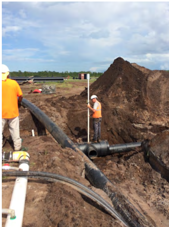
Photograph 36: Confirming slopes of installed pipe.
