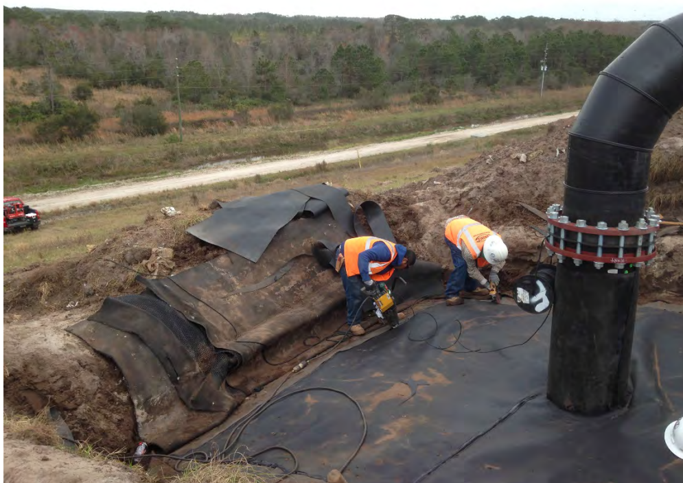
Photograph 67: 18-inch header repair/boot in progress.
