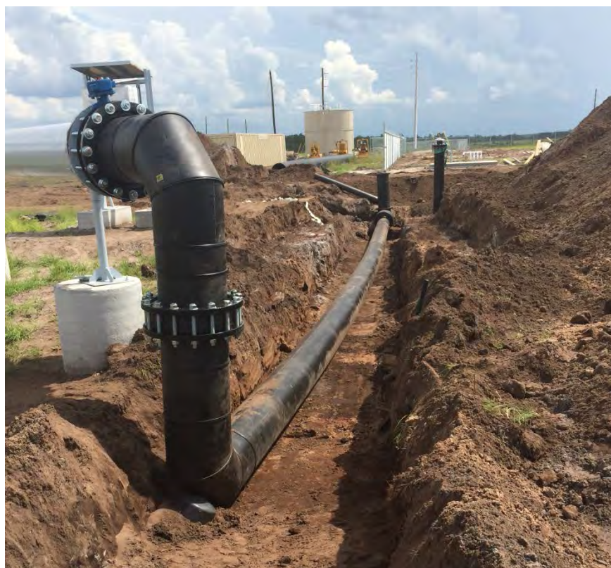
Photograph 52: 16" connection to Flare 2.
