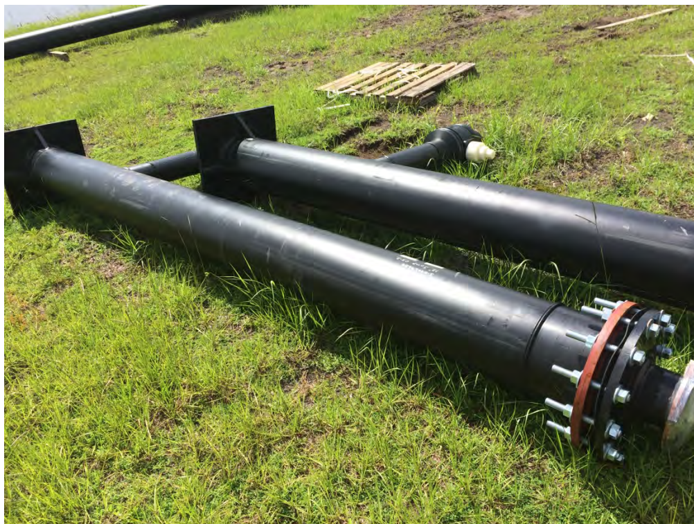
Photograph 39: Prefabricated condensate sump assemblies.
