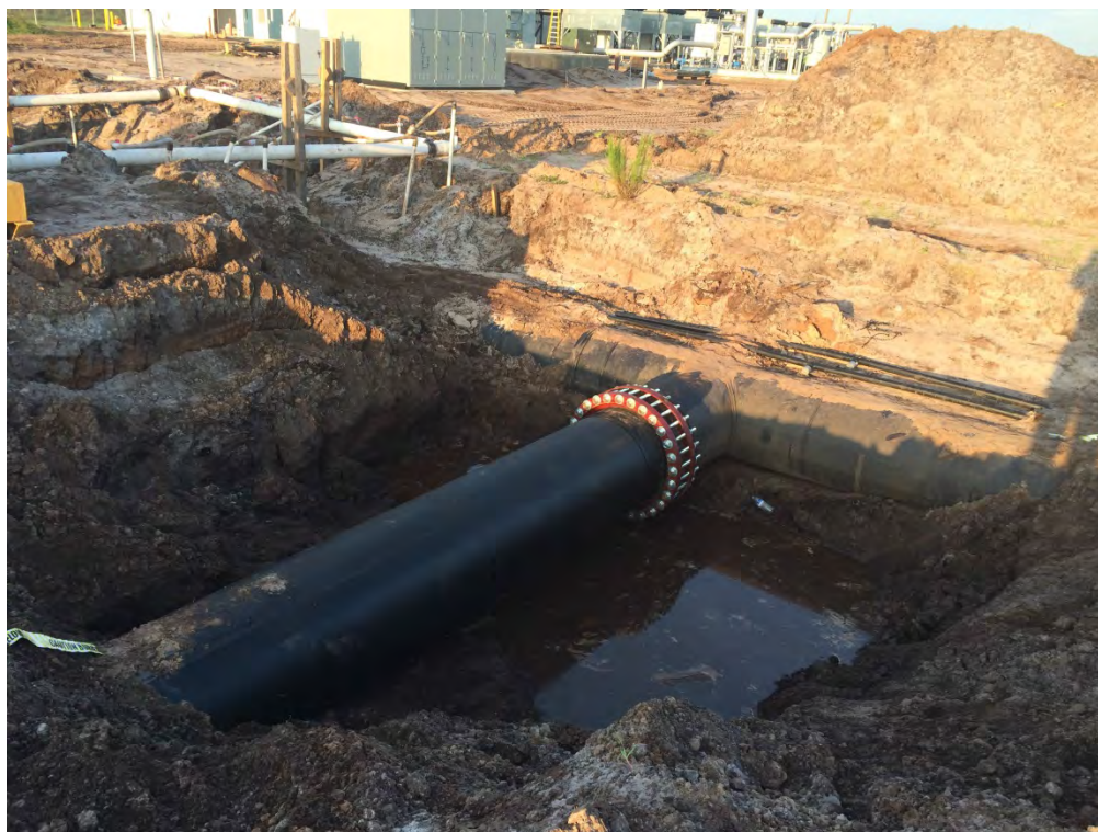
Photograph 40: Installed flanged connection at 30" tee.
