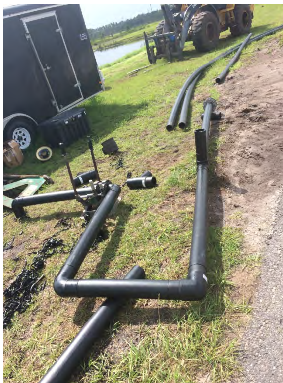
Photograph 46: Constructing J-trap assembly for flare condensate drains to CS-4.
