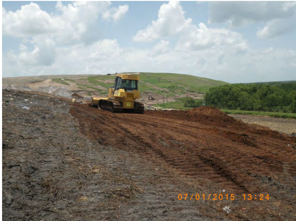
Photograph 18: Regrading slopes with dozer (typical).
