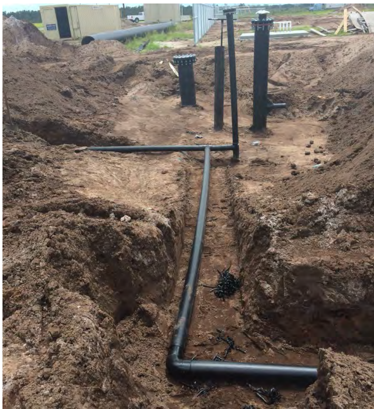
Photograph 49: 4" flare condensate drain from Flare 1 to CS-4.
