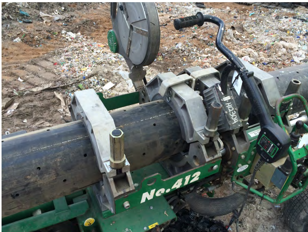
Photograph 21: Fusing of perforated pipe for HGC (typical).
