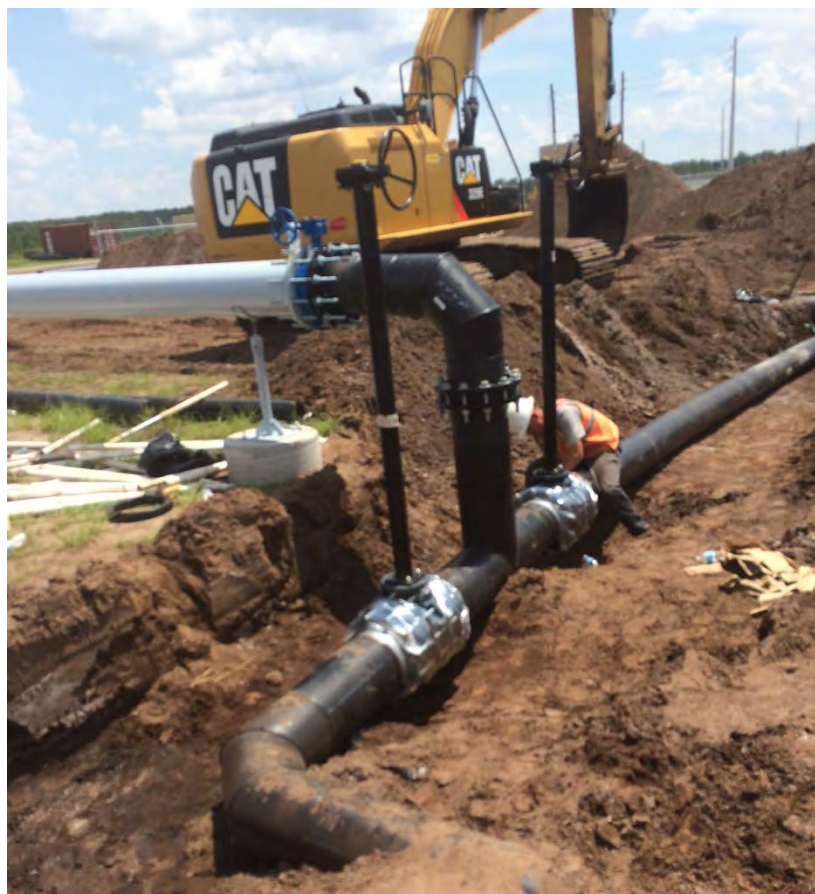
Photograph 54: Completed 12" connection to Flare 1.
