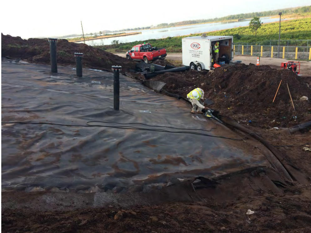
Photograph 57: Cleaning of geomembrane in Cell 1.
