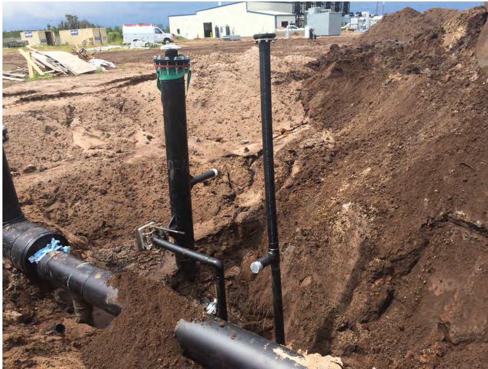
Photograph 47: Welding J-trap to CS-4.
