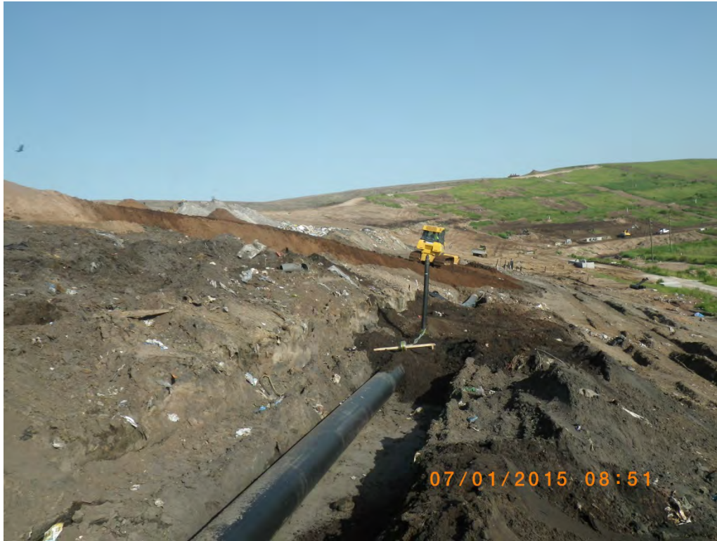
Photograph 17: Backfilling trench. Caution tape applied and survey posts every 50' and at points of interest (typical).
