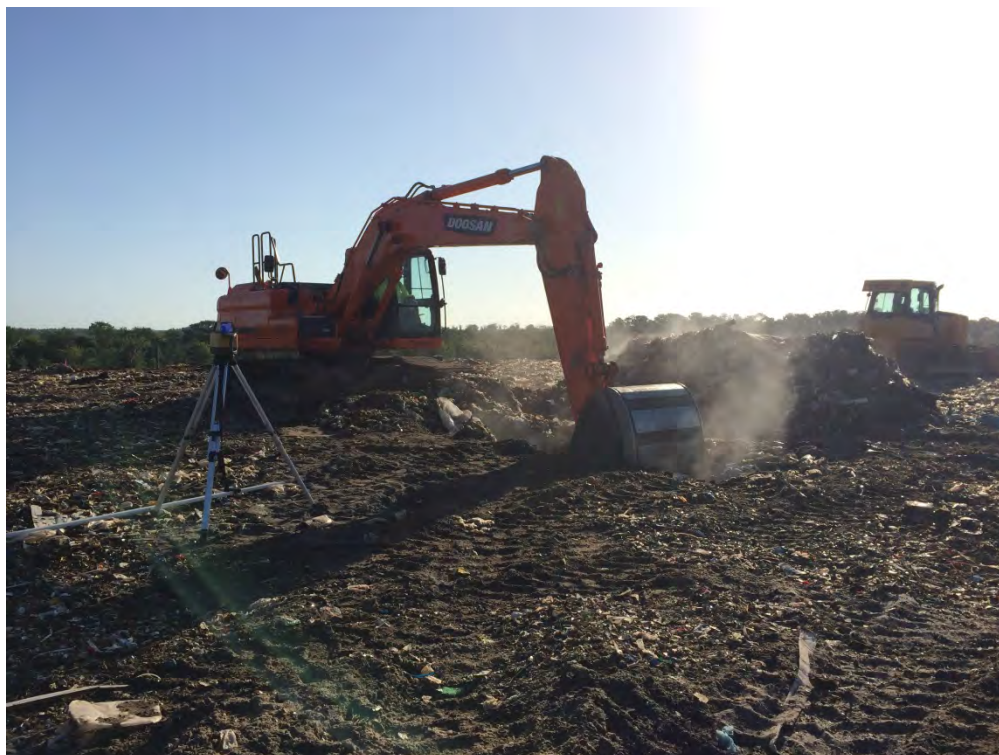
Photograph 22: Excavation of HGC trench (typical).
