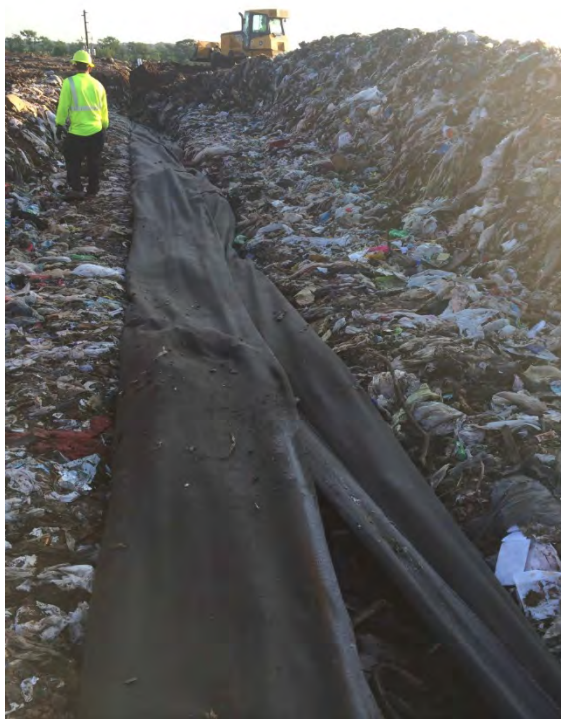
Photograph 25: Wrapping of tire chips and HGC pipe (typical).
