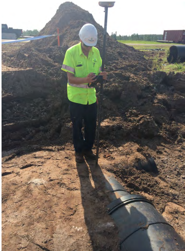
Photograph 41: Progressive staff confirming slopes and elevations of installed pipe.
