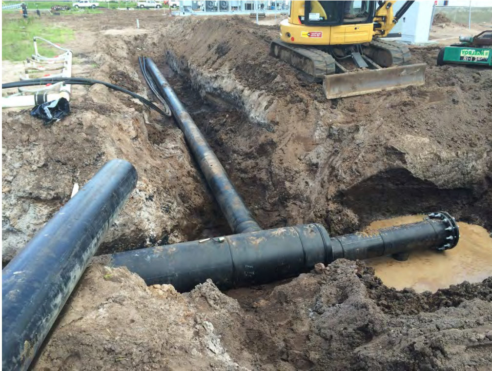
Photograph 37 Installed 24" to 14" assembly.
