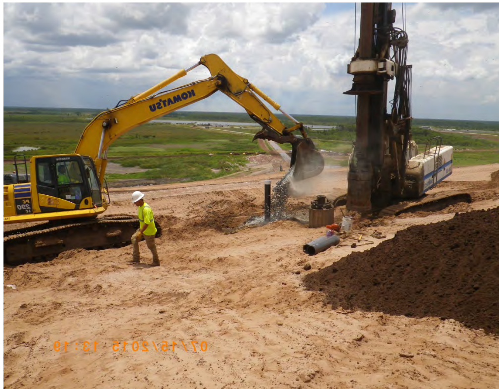
Photograph 8: Backfilling extraction well with approved stone (typical).
