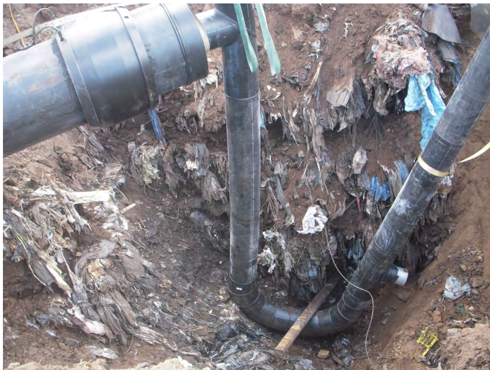
Photograph 27: Installed condensate trap in Cell 1.
