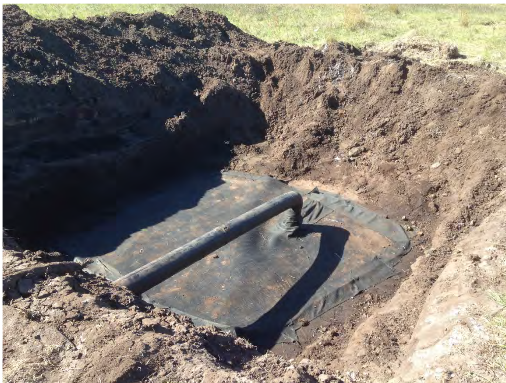
Photograph 64: Lateral tie-in boot/repair (typical)
