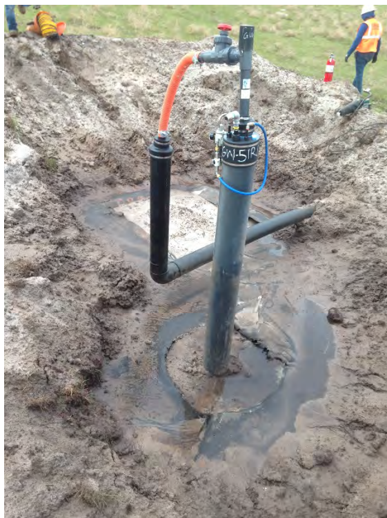
Photograph 59: GW-51R1 booting/repair of geomembrane.
