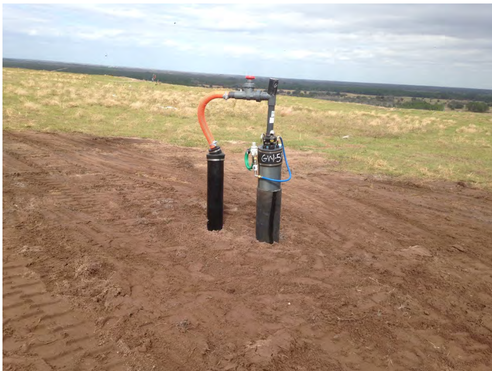
Photograph 63: GW-51R1 completed boot/repair with area regraded.
