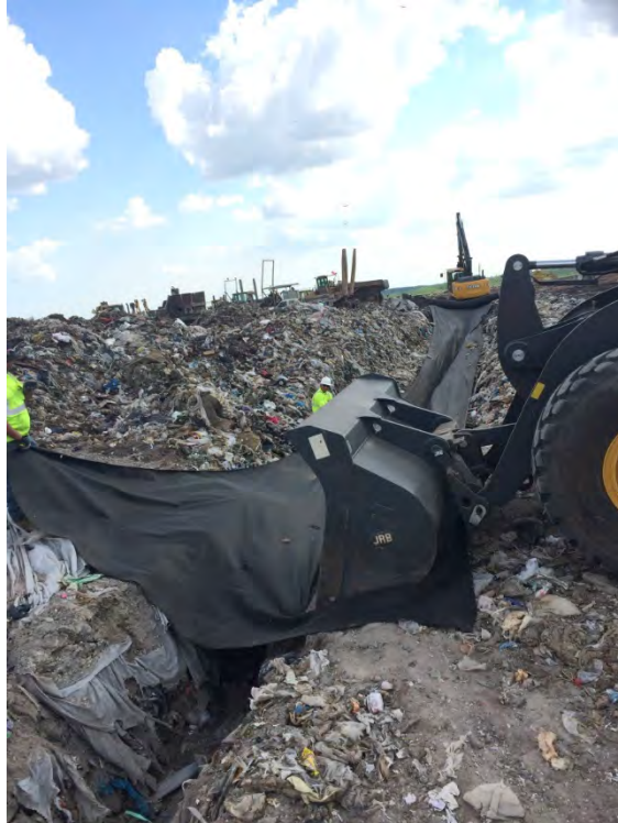
Photograph 23: Installation of 8-ounce geotextile (typical).
