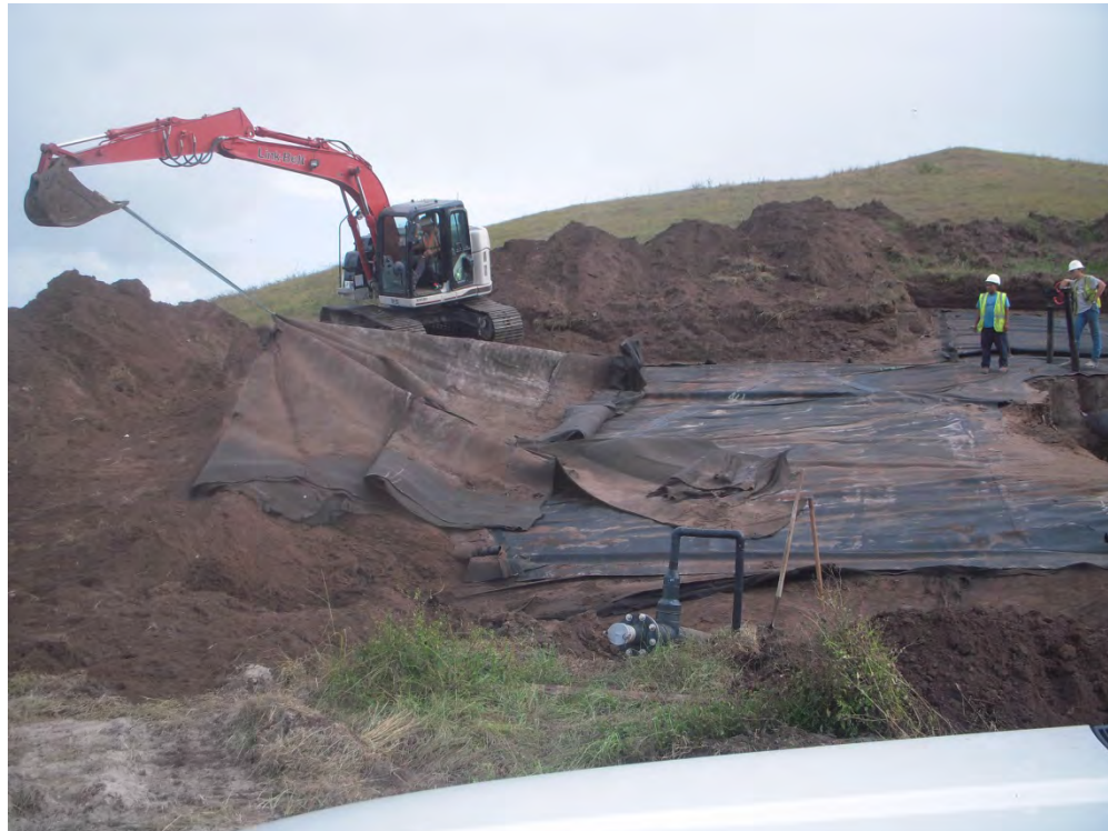
Photograph 26: Removal of geosynthetics in Cell 1 for condensate trap drain line installation.
