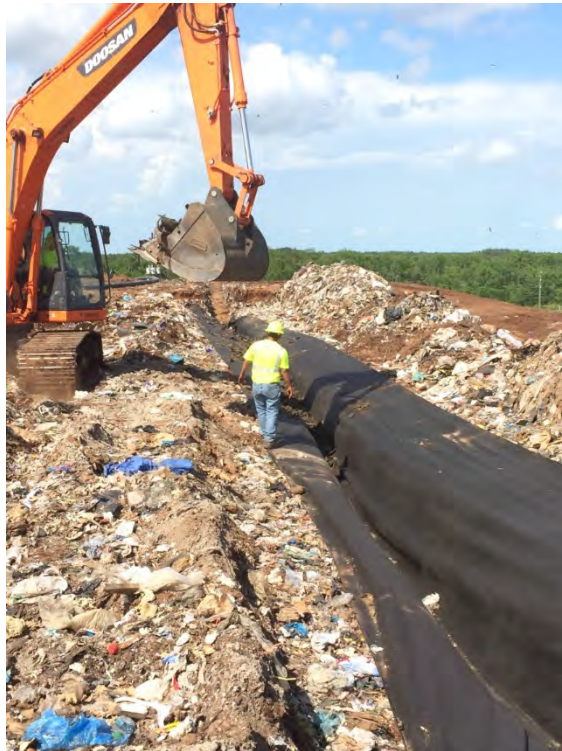
Photograph 24: Placement of tire chips (typical).
