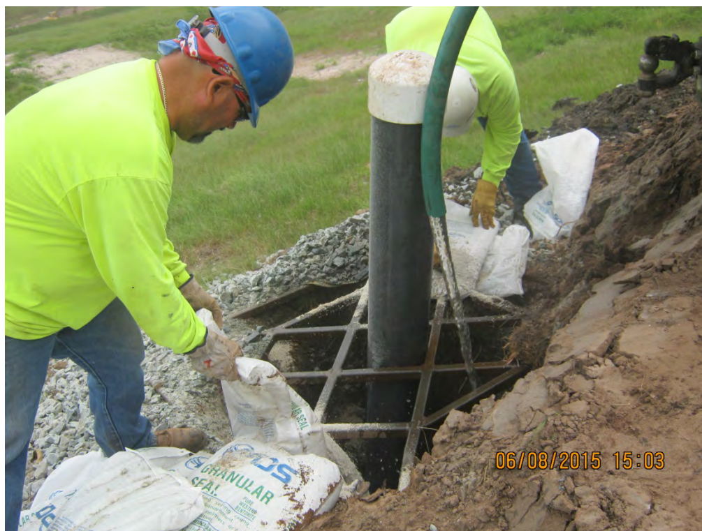
Photograph 9: Hydrating bentonite plug at extraction well (typical).
