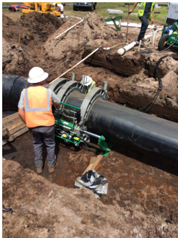
Photograph 34: Welding 30" pipe assembly to 30" elbow.
