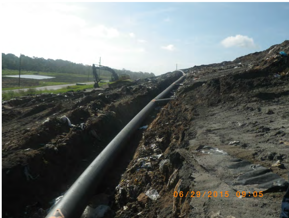
Photograph 15: 18" Header pipe in trench.
