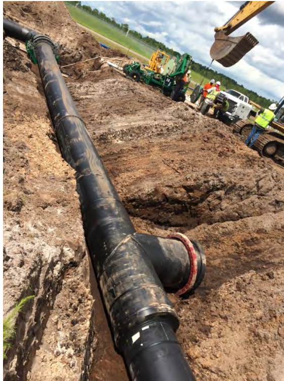
Photograph 35: Installed 30" to 24" pipe assembly.
