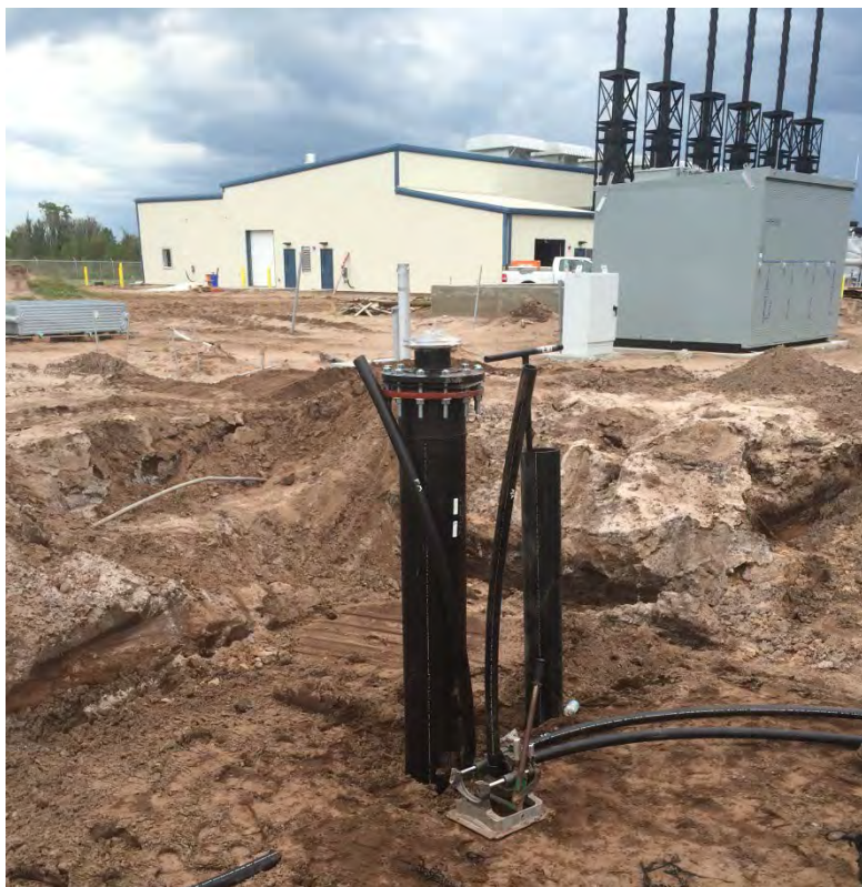
Photograph 45: Welding air and forcemain lines adjacent to CS-2 (typical).
