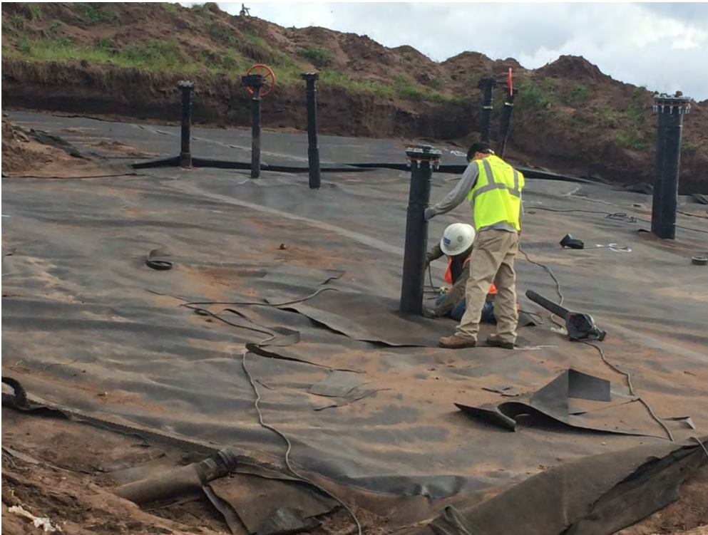
Photograph 56: Geomembrane boot repair in Cell 1.
