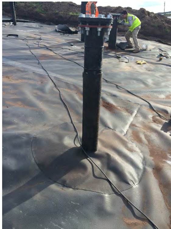
Photograph 58: Geomembrane boot repair prior to welding.
