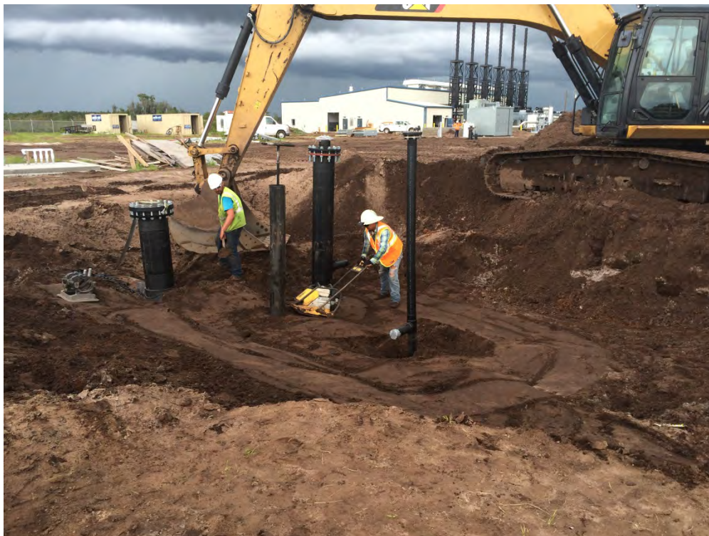
Photograph 48: Backfilling and compacting soil (typical).
