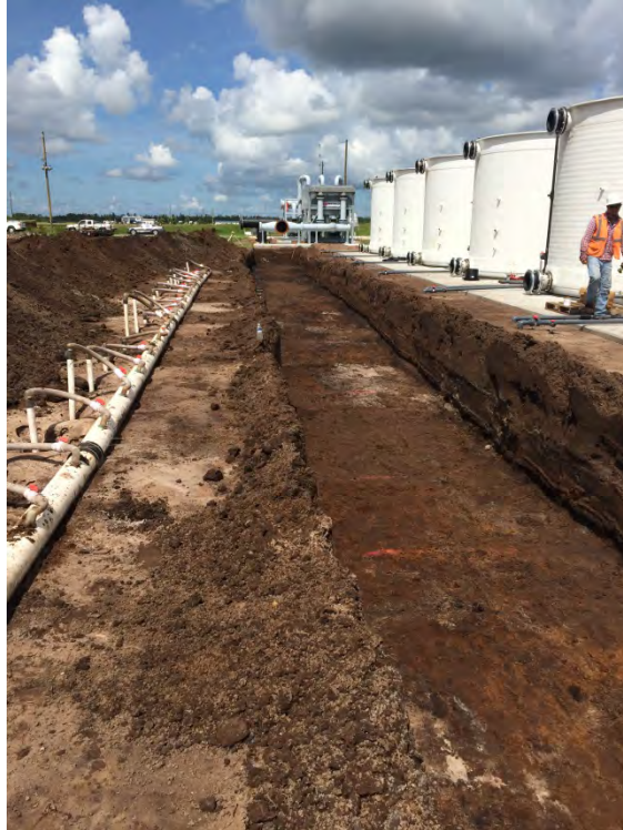
Photograph 29: Trenching for main 30" Headers.
