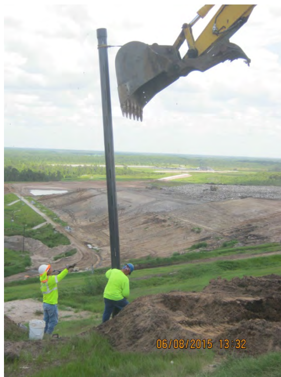
Photograph 11: Setting has well screen (typical).
