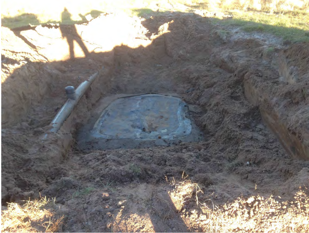
Photograph 65: Abandoned well geomembrane repair (typical).
