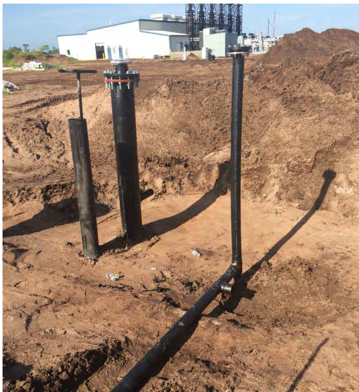
Photograph 51: J-trap cleanout and 4" drain from Flare 2.
