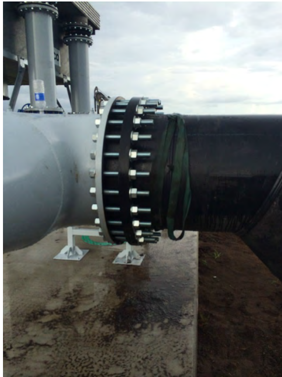
Photograph 33: 30" Flanged connection to Cooling Unit.
