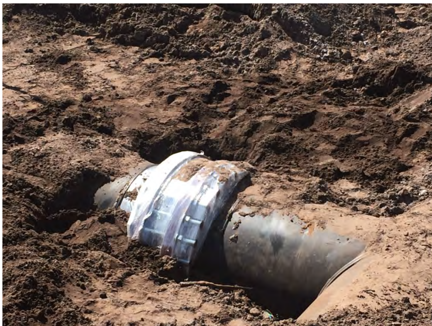
Photograph 53: Flange bolts wrapped with 10 mil plastic and taped to pipe.
