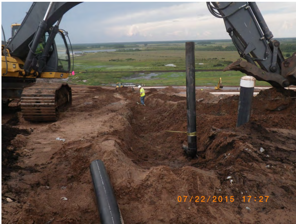
Photograph 14: Installing new lateral assembly (typical).
