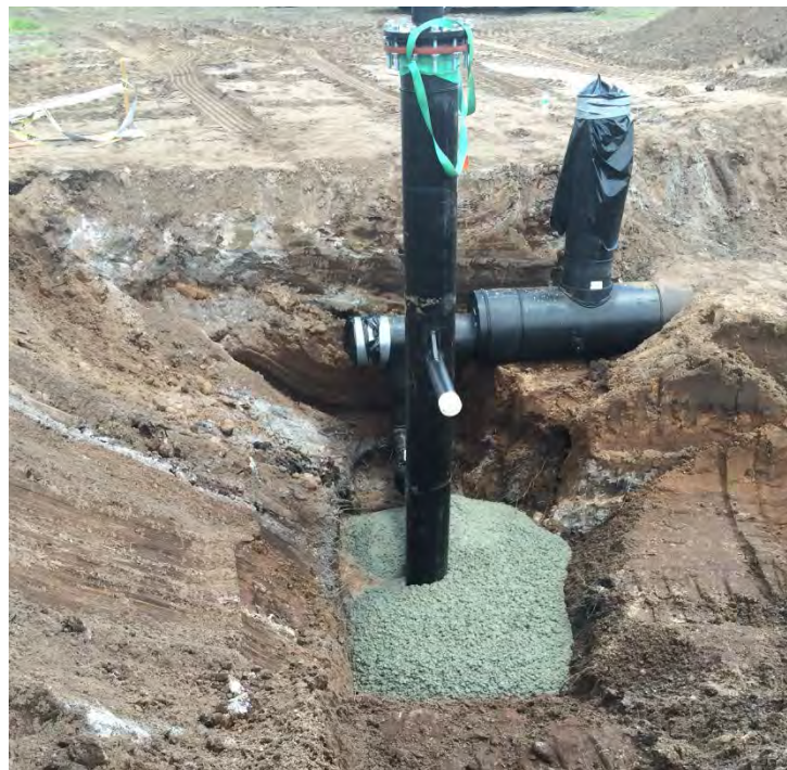
Photograph 44: Concrete placed at base of CS-4 (typical).
