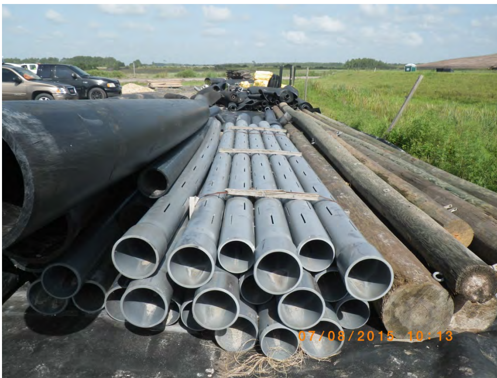
Photograph 2: 8" SCH 80 slotted PVC pipe.
