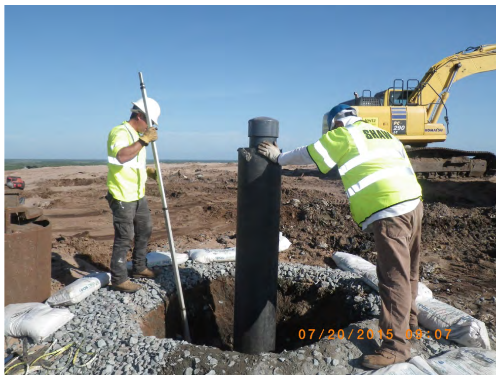
Photograph 10: Encasement pipe at well GW-T100.
