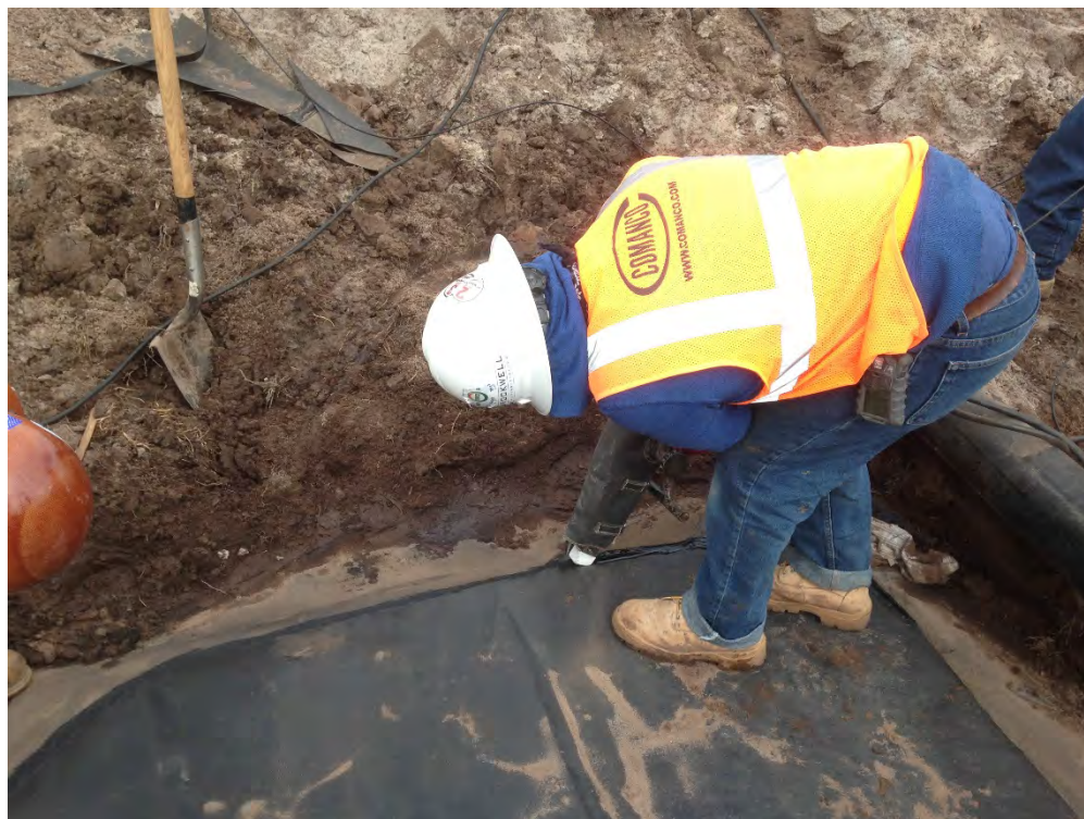
Photograph 60: Welding of geomembrane repair (typical).
