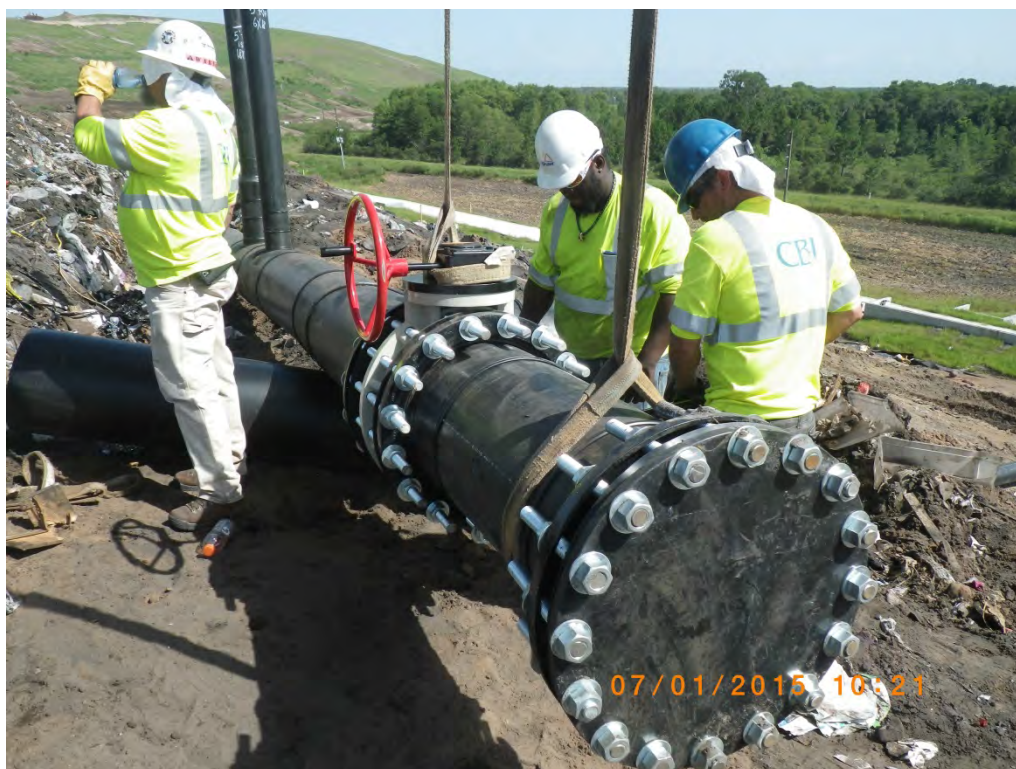
Photograph 16: 18" Valve and blind flange assembly installation in Cell 10.
