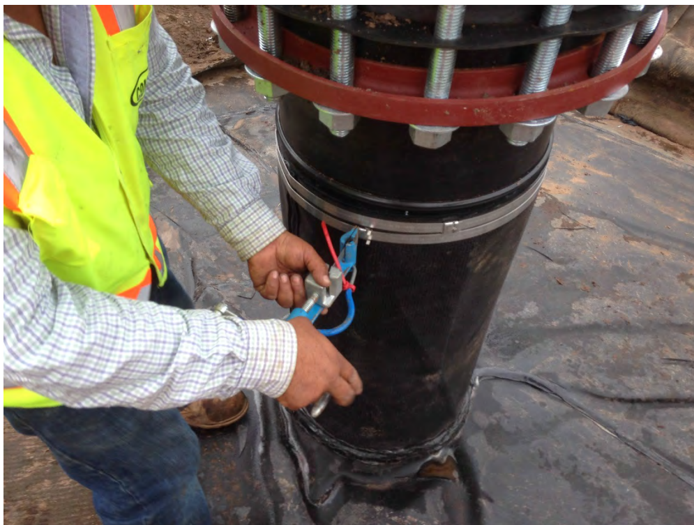
Photograph 68: Banding of boot to 18-inch header.
