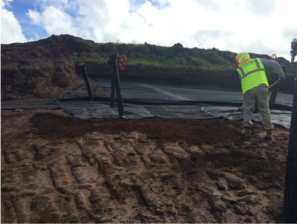
Photograph 55: Raking of geomembrane subgrade in Cell 1.
