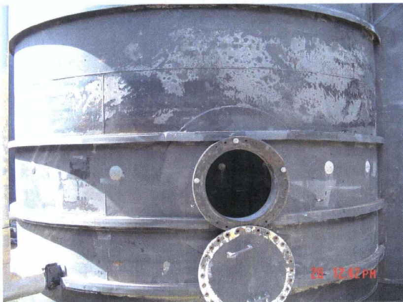
15. Clarifier shell bottom and manway.
