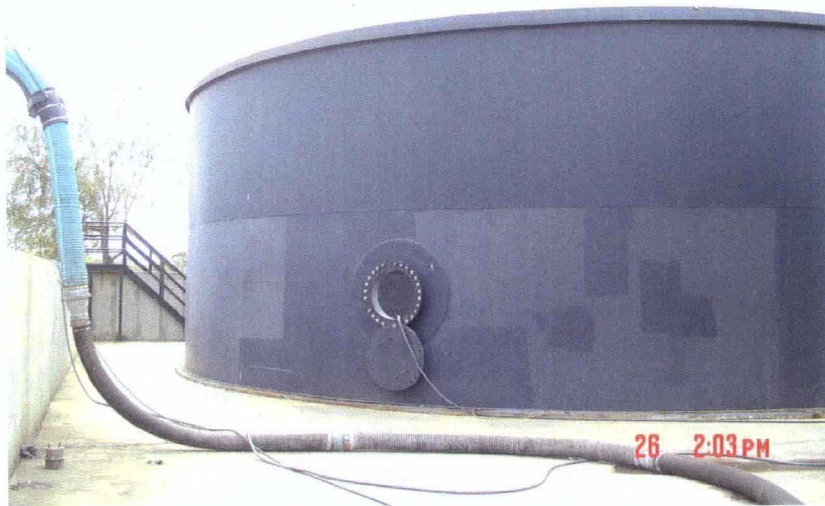
1. Tank north side.
