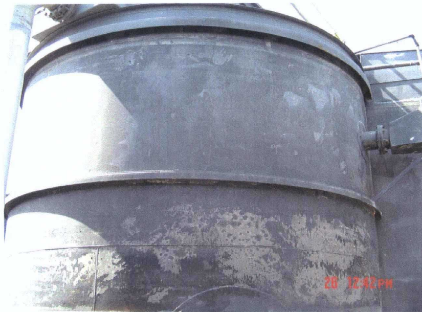
13. Clarifier shell top.
