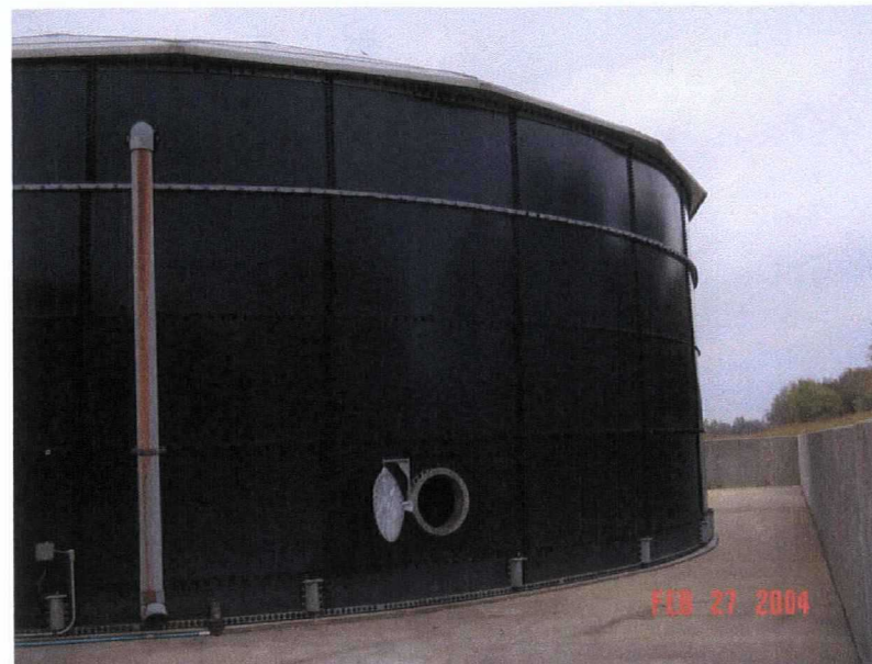
2. Tank south side.
