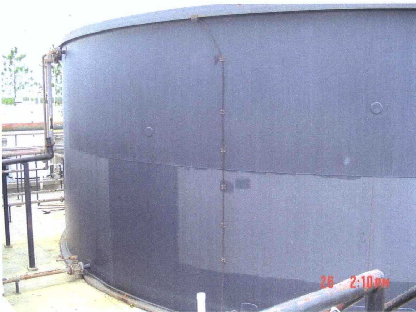
3. Tank south side.
