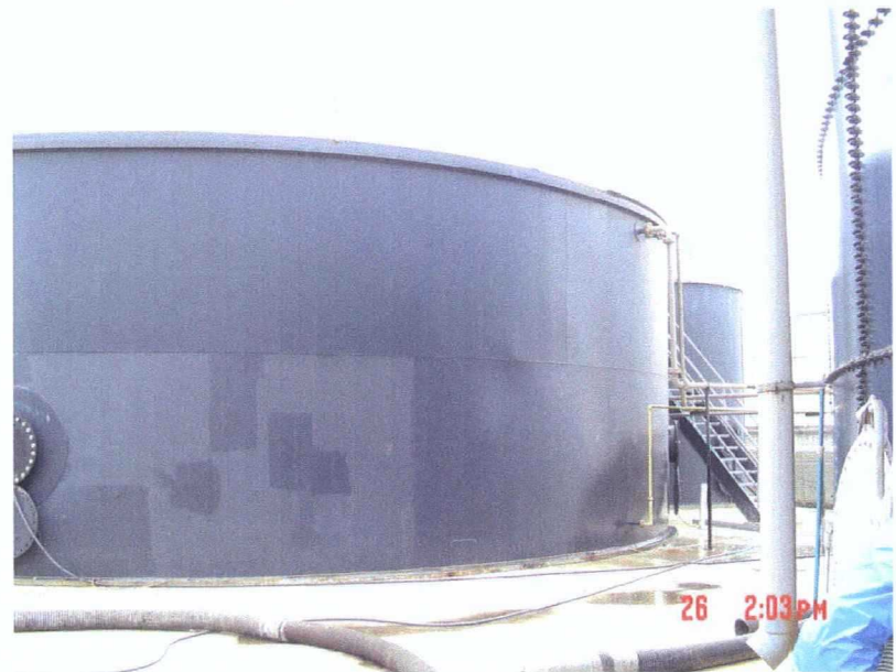
2. Tank north side.
