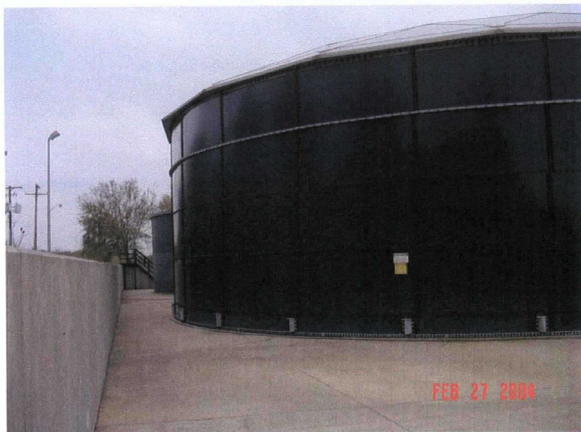
3. Tank north side.
