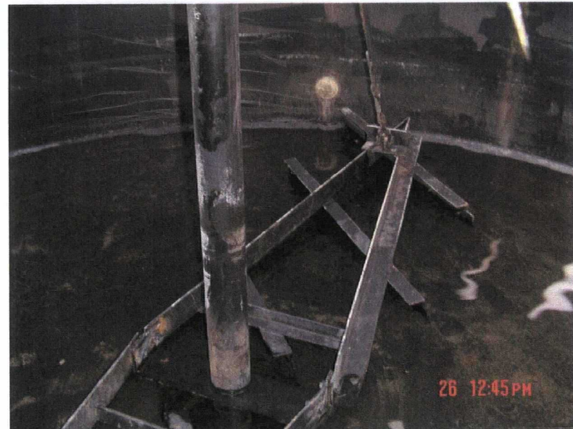
16. Clarifier center bottom.
