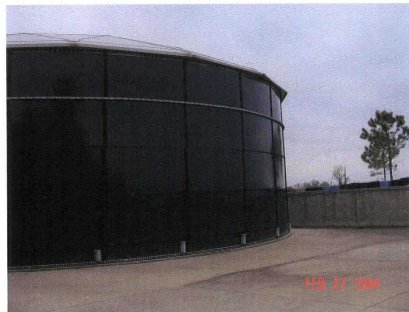
4. Tank north side.
