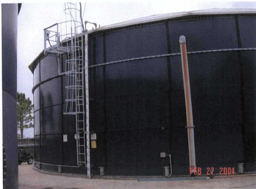
1. Tank south side.
