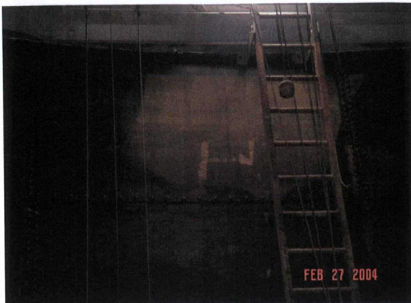
17. Interior ladder top.
