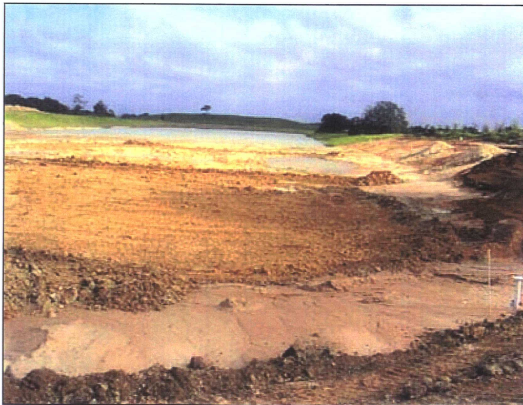
Pit 1, completed lift 1 looking north
