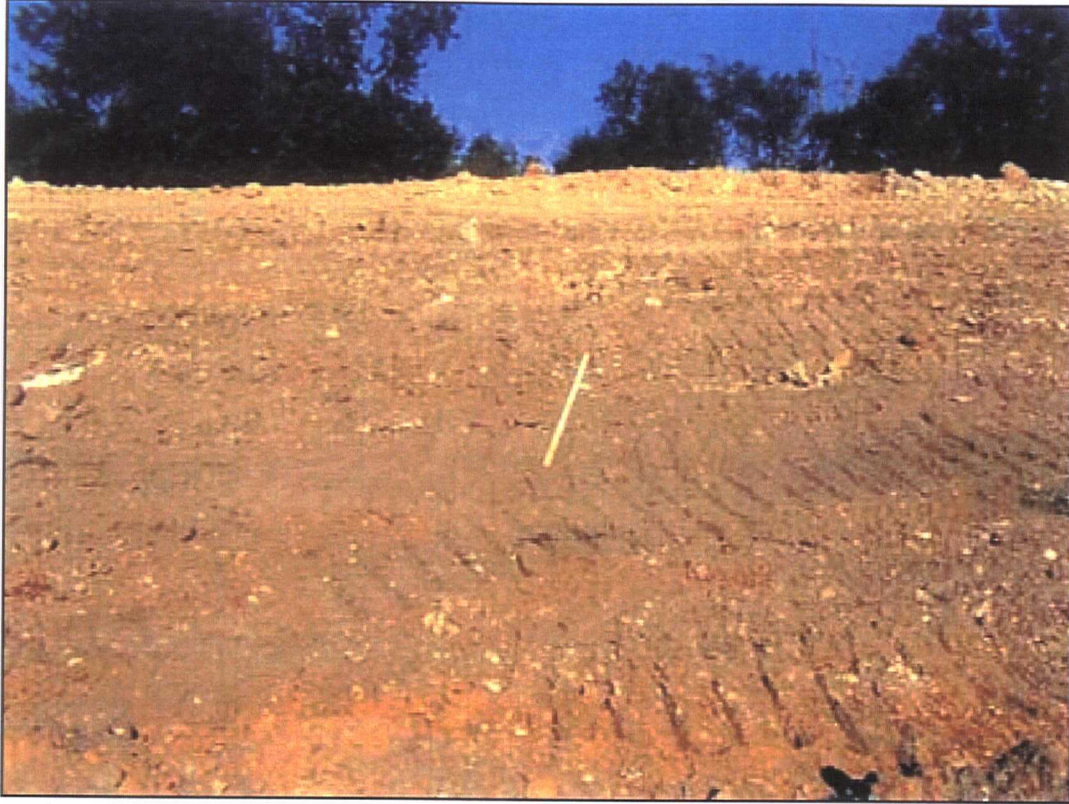
Pit 12, completed lift 3 looking east
