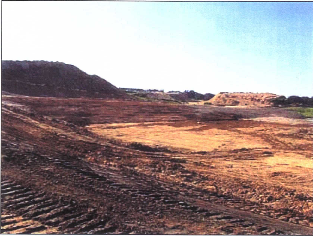
DCP081-DCP086 Completed Cell one beginning sw corner ending se corner
