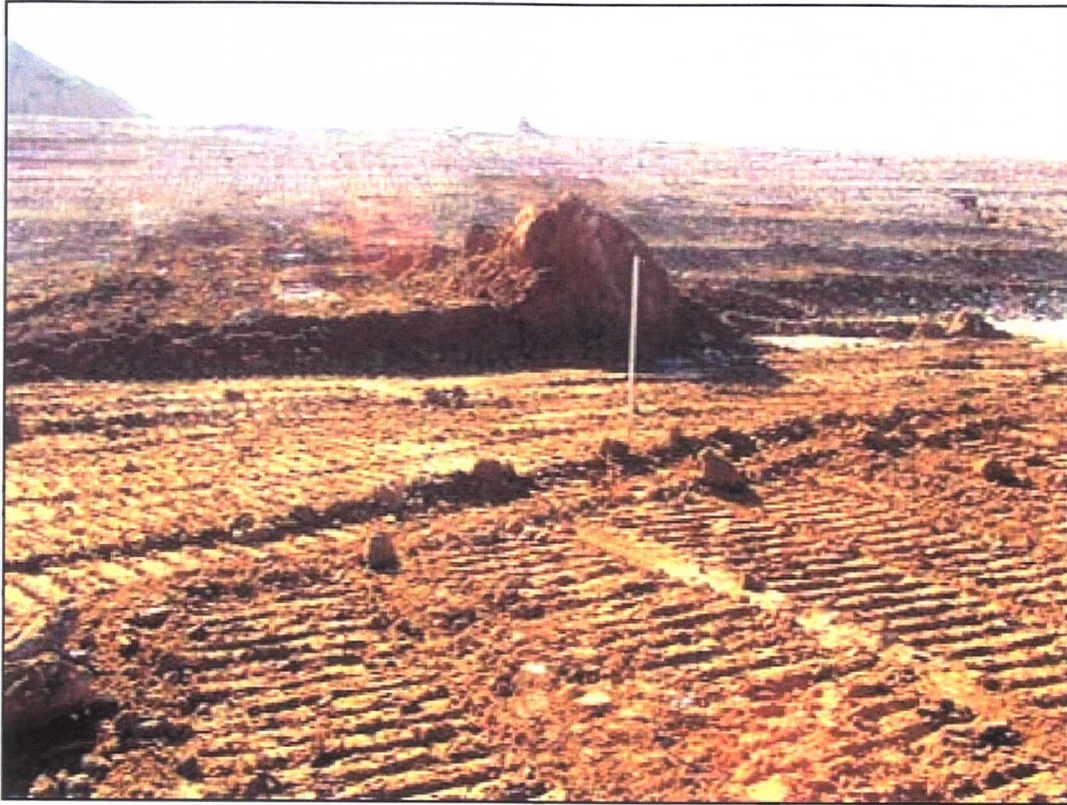
Pit 10, completed lift 3 looking west
