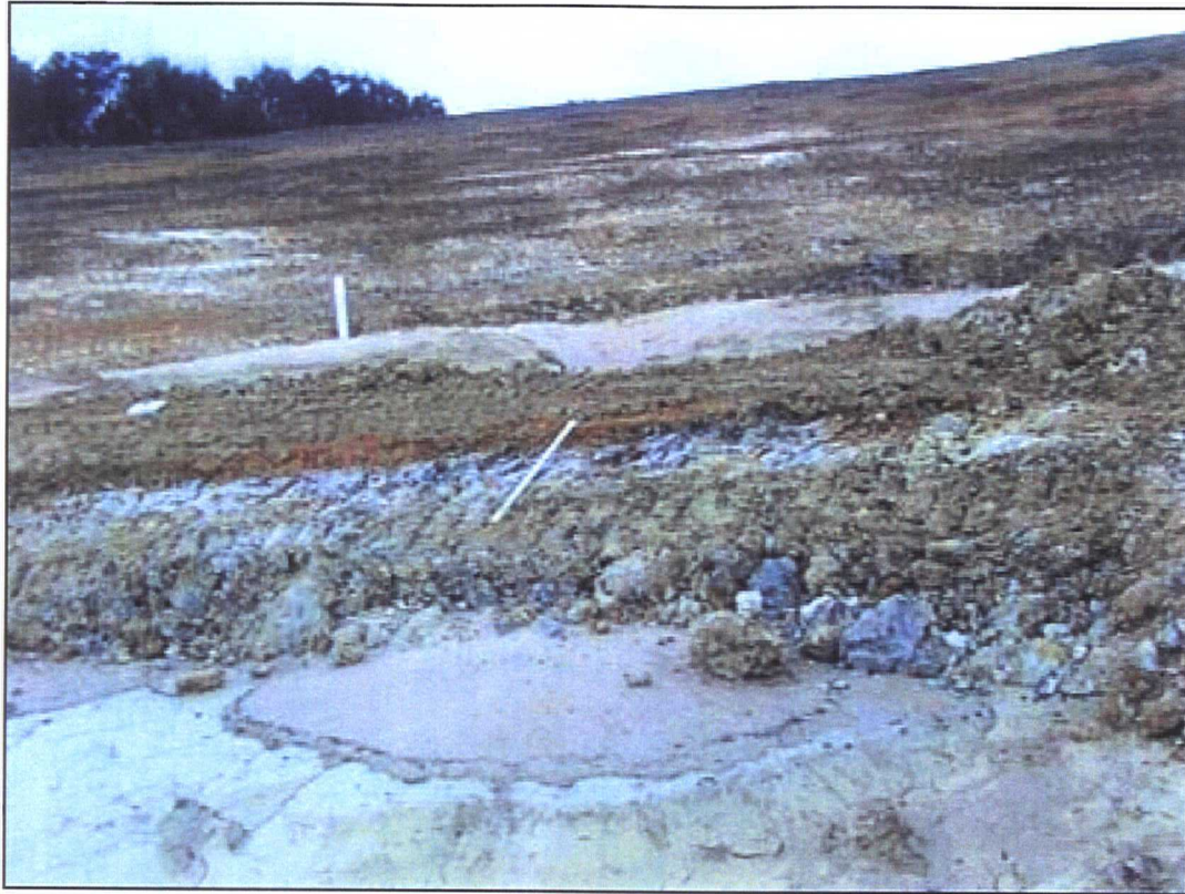
Pit 1, south slope
