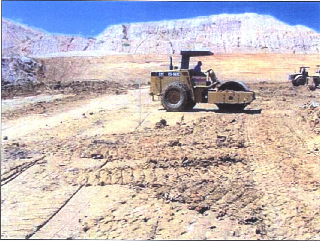
Pit 2, completed lift 3 looking west
