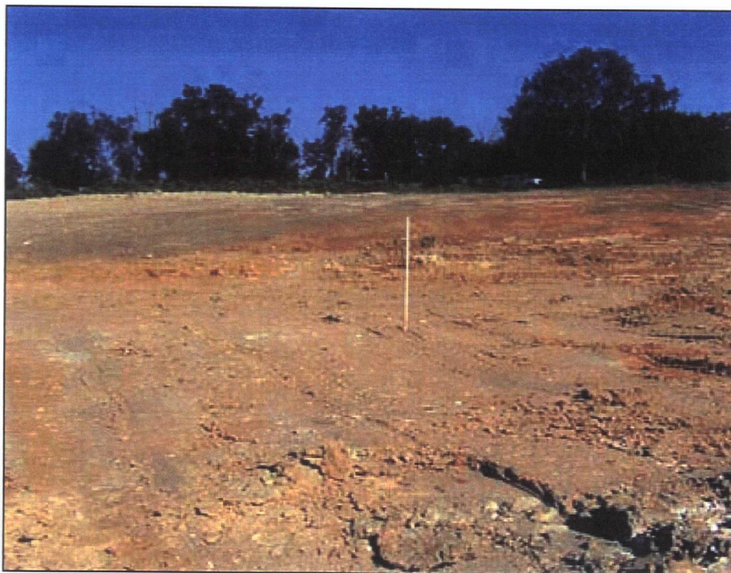
Pit 8, completed lift 3 looking east
