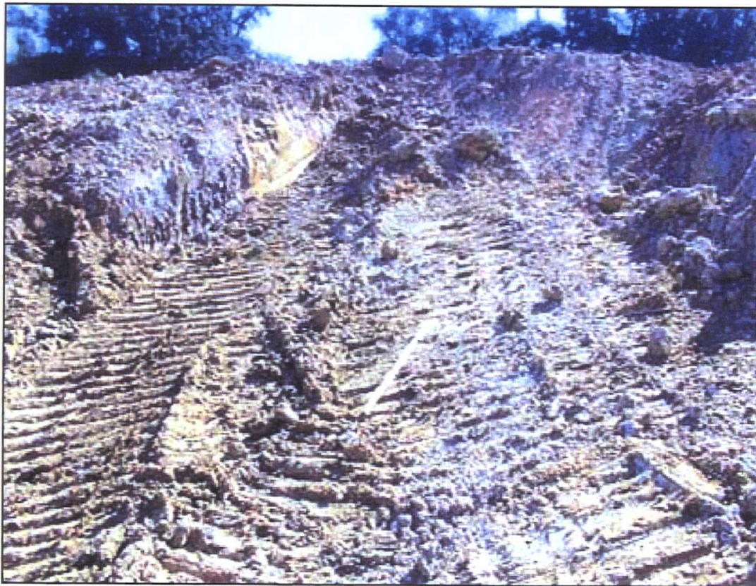
Pit 11, completed lift 1 looking east
