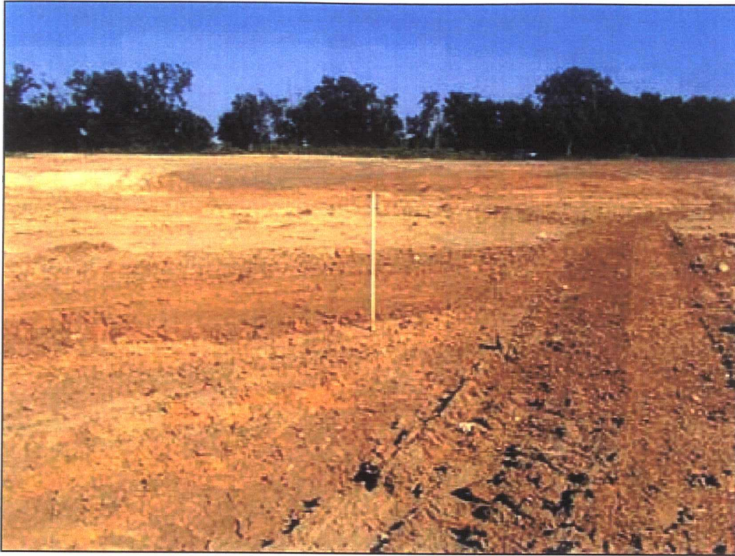
Pit 5, completed lift 3 looking east
