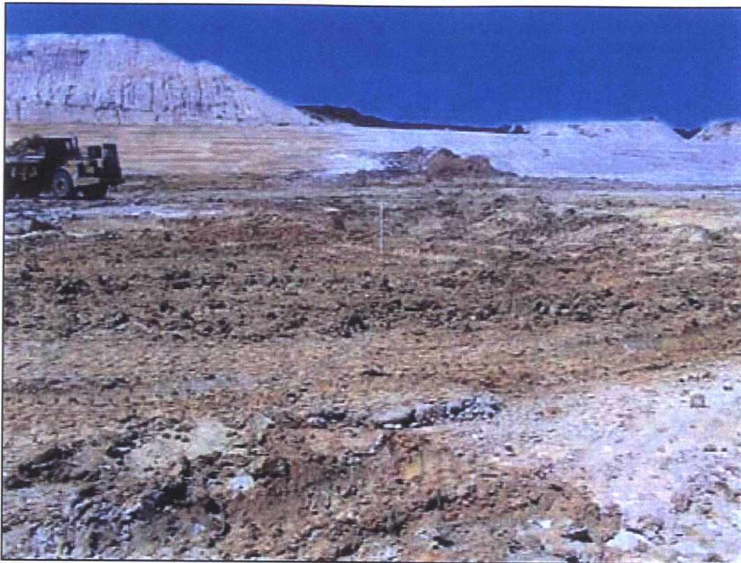
Pit 8, completed lift 2 looking northwest
