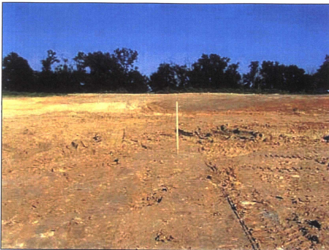
Pit 9, completed lift 3 looking east
