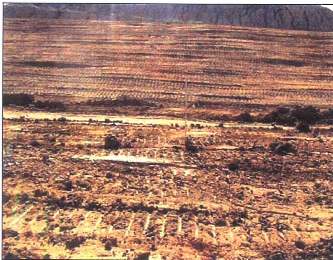
Pit 4, completed lift 3 looking west
