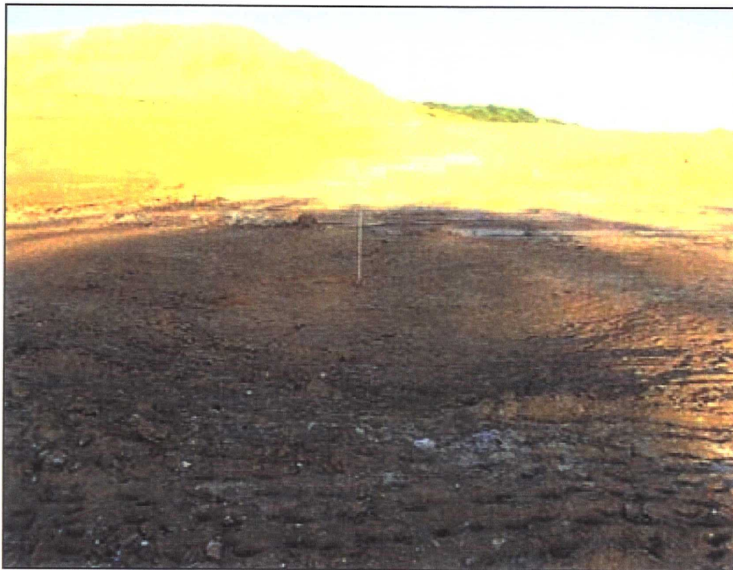
Pit 9, completed lift 1 looking northwest
