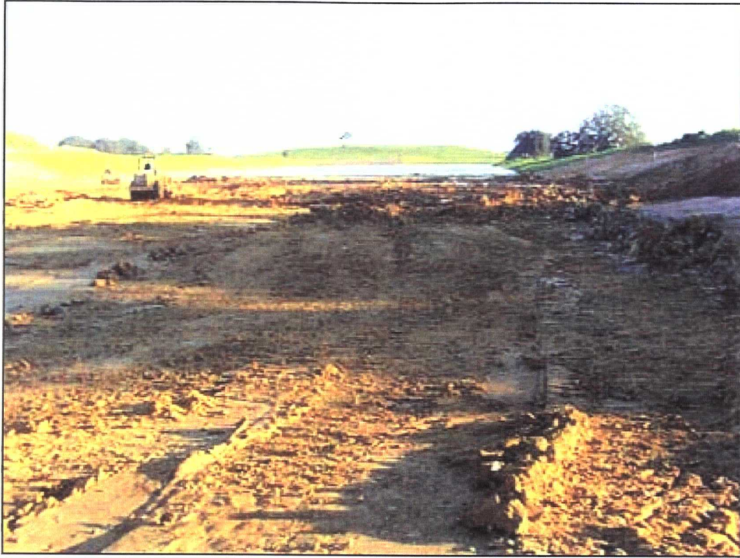
Pit 1, completed lift 2 looking north
