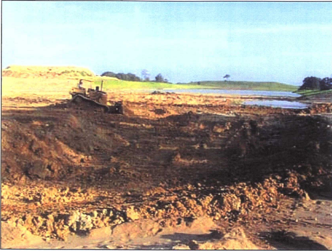
Pit 1, lift 1 looking north
