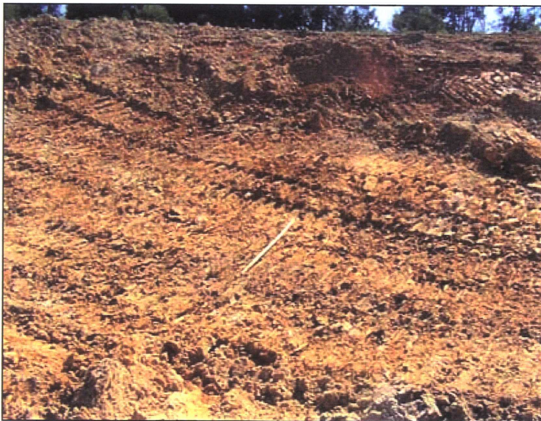
Pit 12, completed lift 1 looking east
