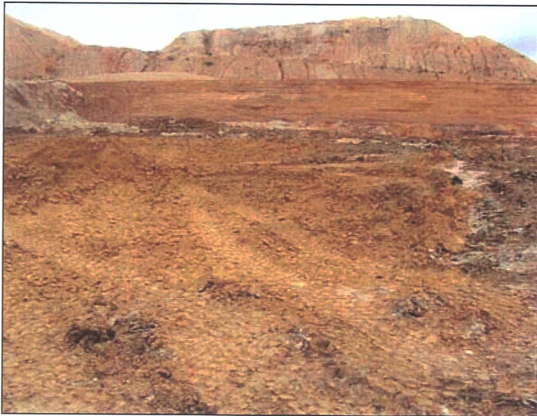
Pit 2, completed lift 1 looking west
