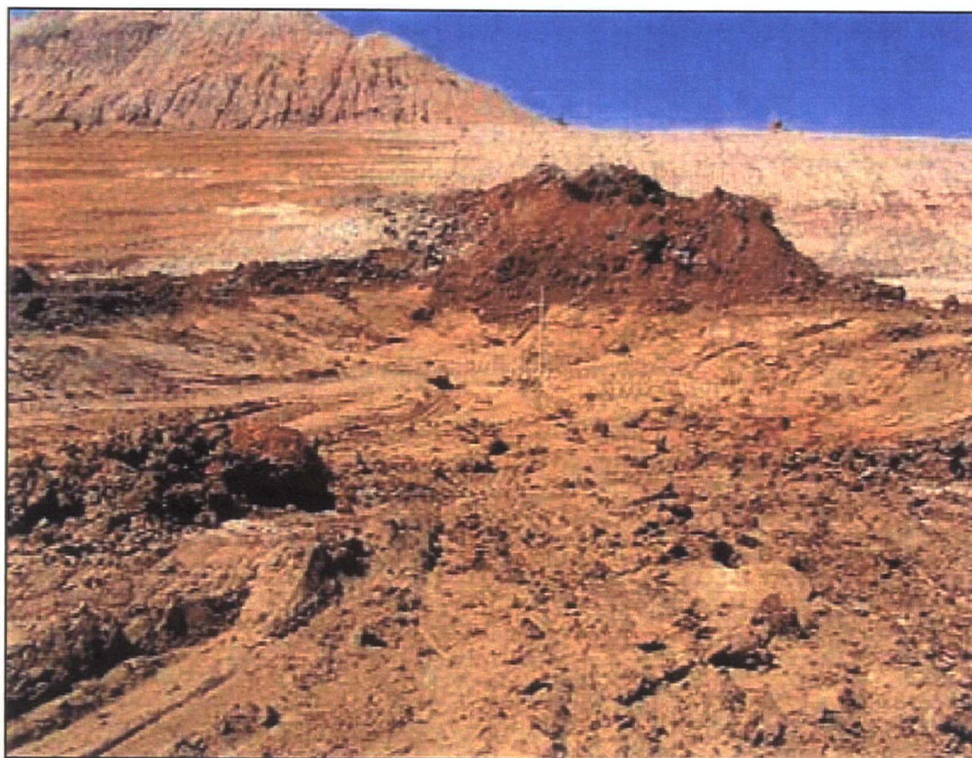
Pit 10, completed lift 1 looking west
