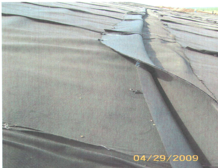
Fig 3: Lateral Drainage Pipes installed during Liner Install.
