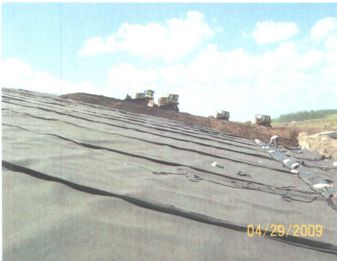
Fig. 1 & 2 – Partial Closure Liner Installation Activities
