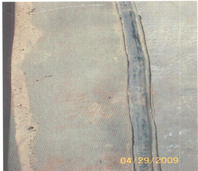
Fig 4: Tie-in of the Base Liner with the Closure liner
