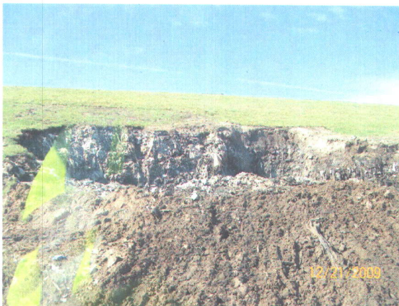
Leachate Seeps Being Repaired
