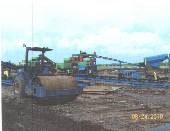
Construction of Auto Fluff Area
