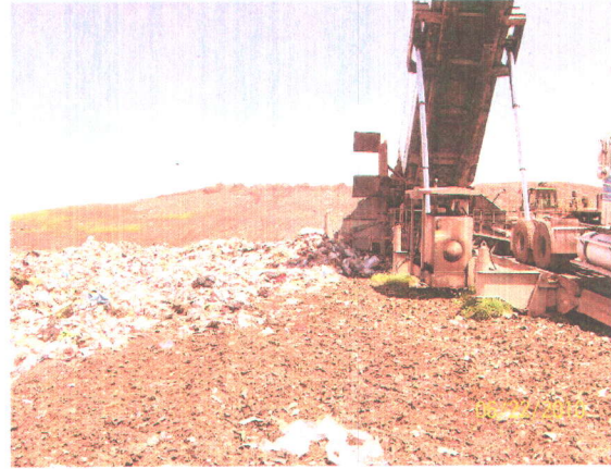
Upper Portion of Working Face
