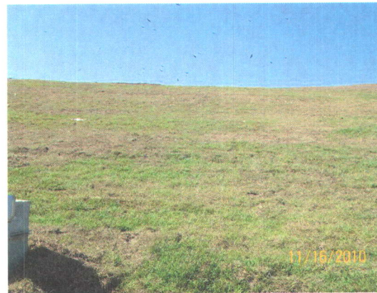
East Side Slope Erosion Repaired
