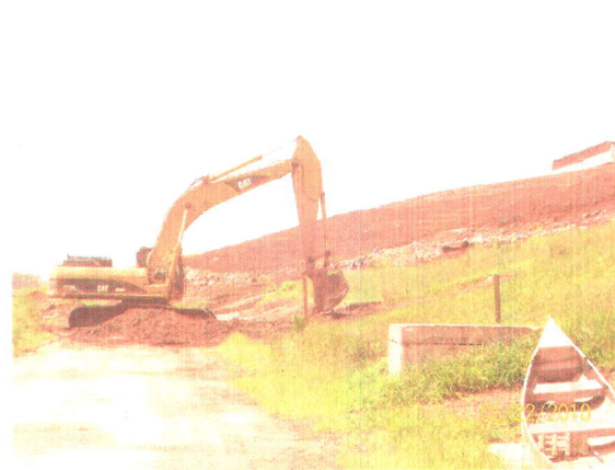
Cell 6 Seepage Repairs
