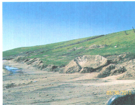
East Side Erosion
