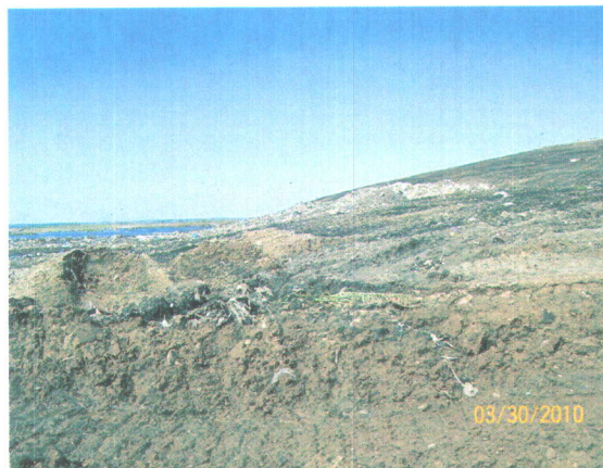
2nd Working Face Area
