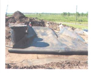
At 3:30 pm Comanco finish repair and G4 complete 10<sup>th</sup> lift at 4:00 pm passing compaction test.
