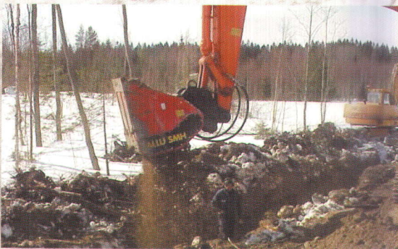
6. Screening of aggregate back into the pipe ditch speeds up the filling process.
