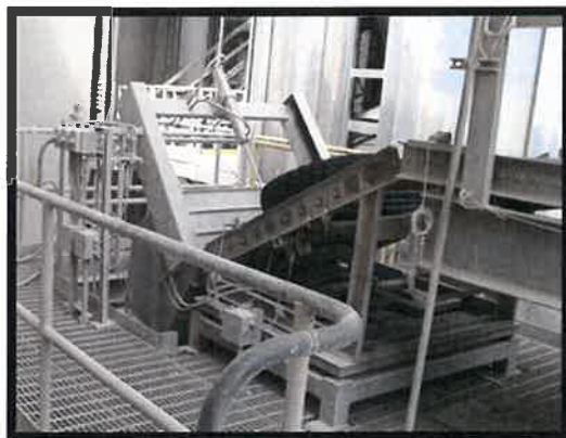
Figure 1. Whole Tire Chute into the Base of the Preheater Tower
