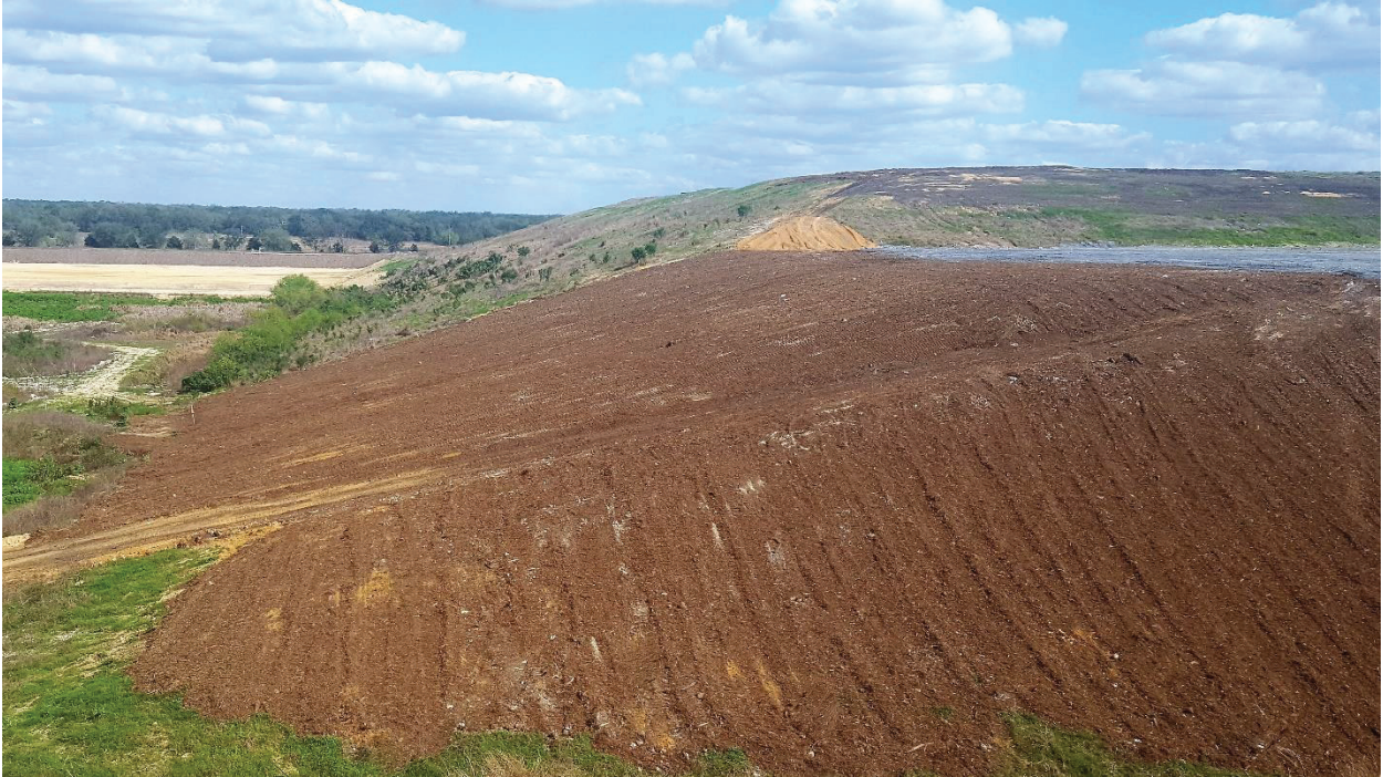
North and Northwest Cells 6 and 7 Initial Cover Maintenance
