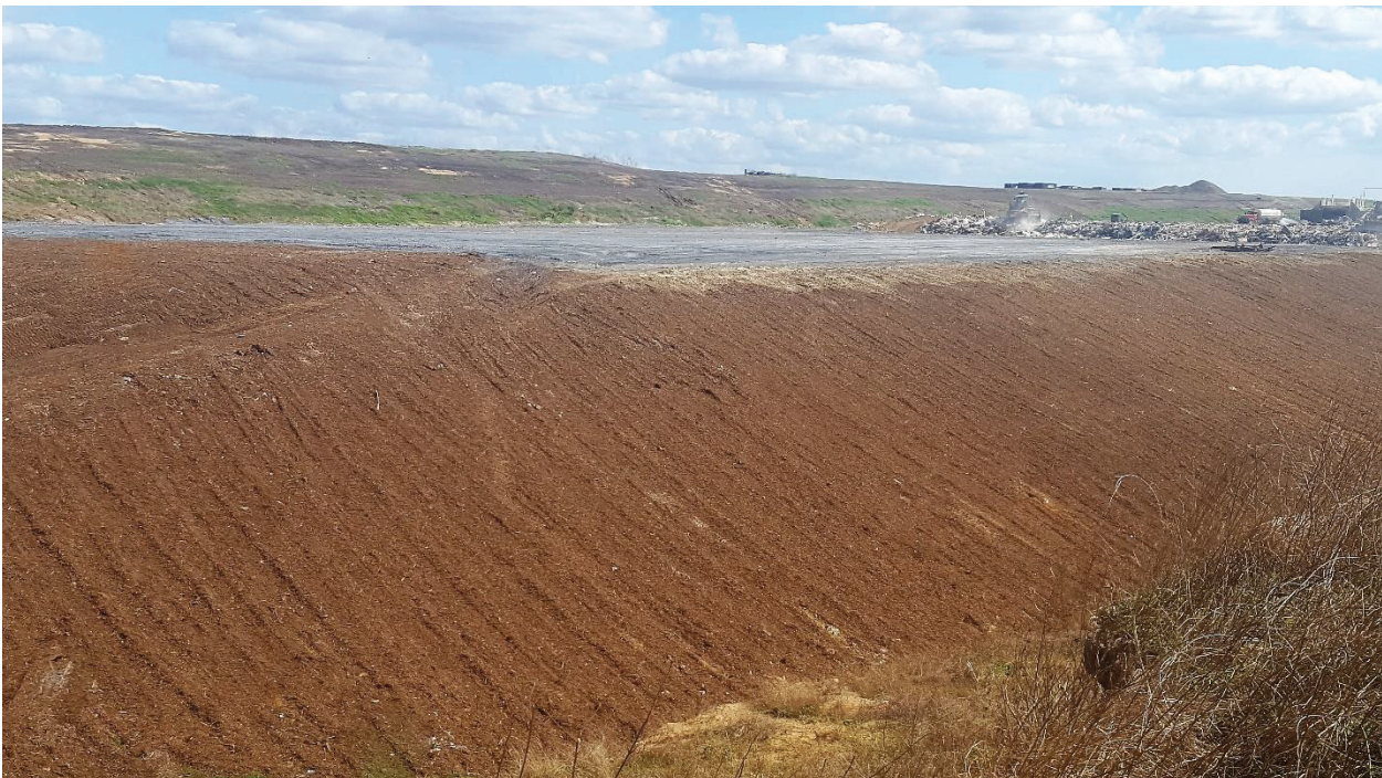
Northwest and West Cell 7 Initial Cover Maintenance
