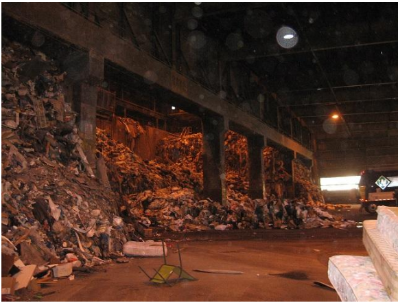
WTE Facility Tipping Floor
