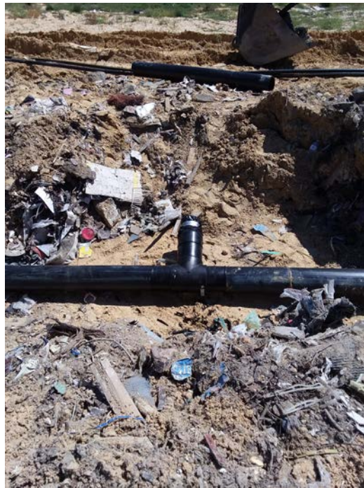
(Photograph 14: 8" tee with 8"x6" reducer for Cell 3 cleanout connection)
