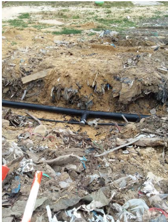
(Photograph 20: 8" tee with 8"x6" reducer for EW-16)
