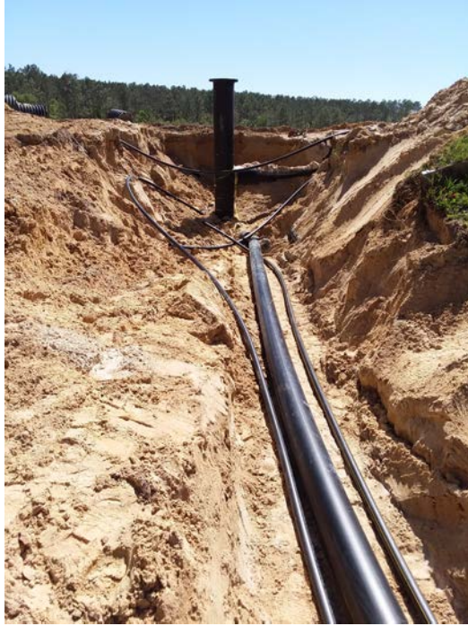
(Photograph 57: 8" header, 2" air, and 2" forcemain placed in same trench starting at CS-4)
