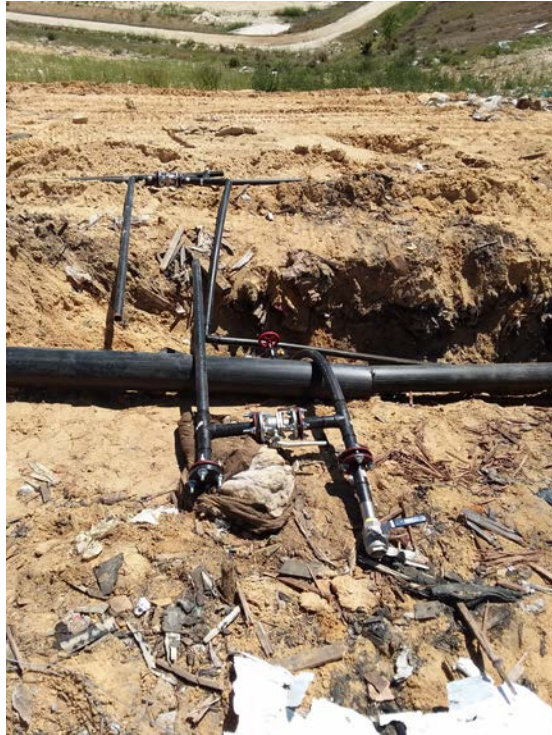
(Photograph 7: 8" valve and 2" air and force main valves)
