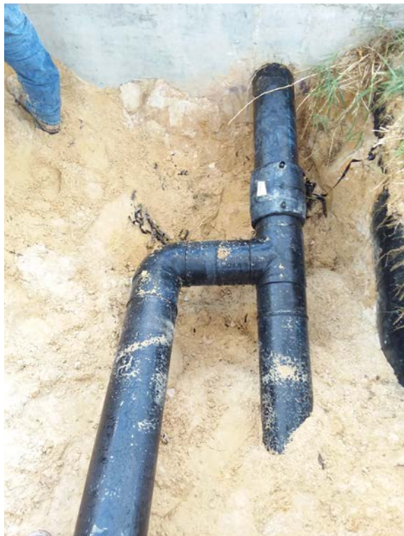
(Photograph 72: 6" tie into Cell 3 cleanout connection)
