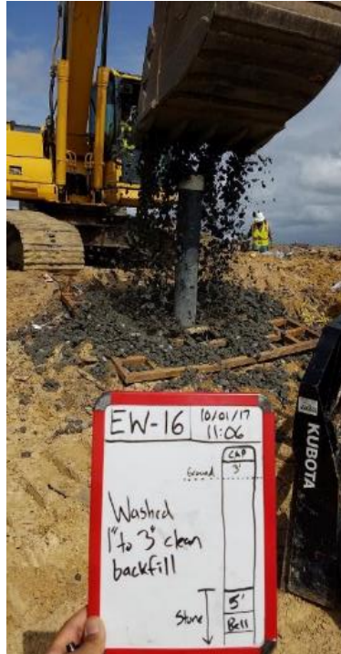
(Photograph 115: W-16 Stone backfill)
