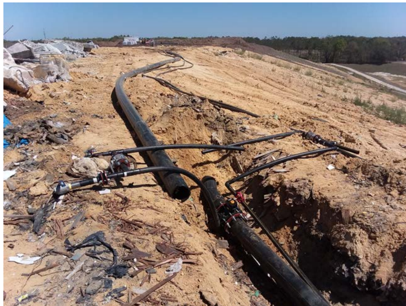
(Photograph 8: 8" header weld with 2" stub ups)
