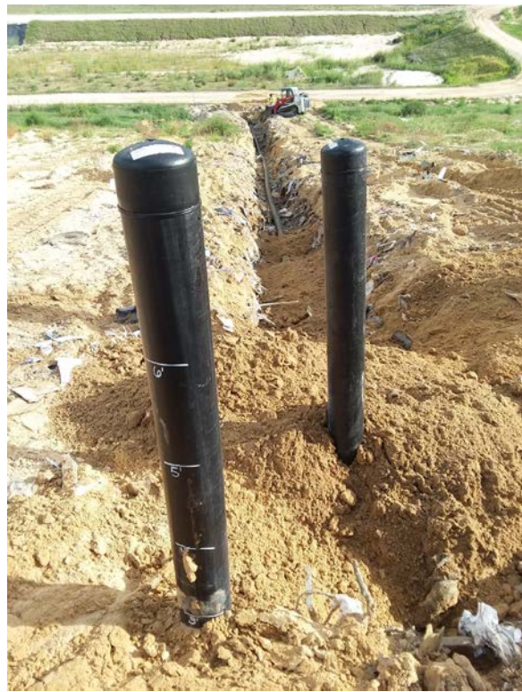
(Photograph 70: 6" riser for Cell 3 cleanout connection)
