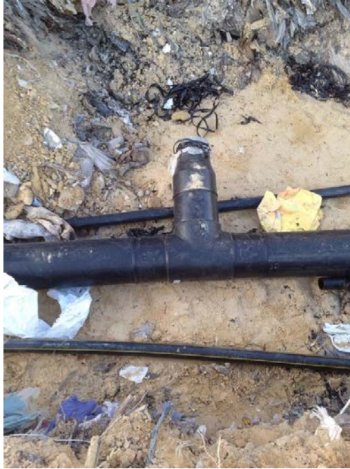
(Photograph 17: 8" tee with 8"x6" reducer for EW-15)
