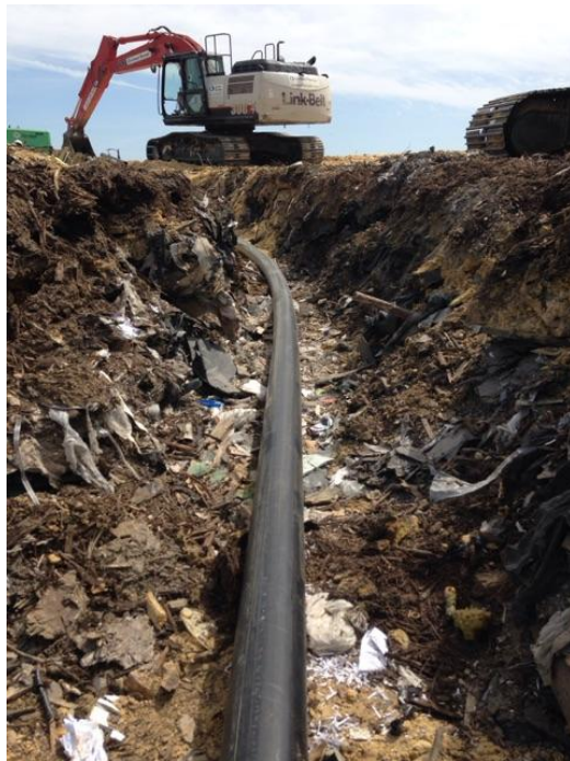
(Photograph 50: 6" lateral to EW-10, HC-11 and HC-12)
