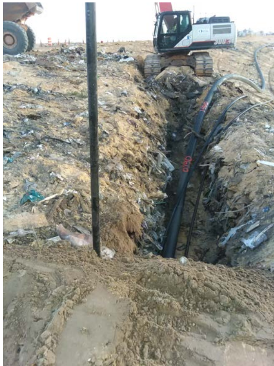
(Photograph 4: 12" pipe placing in trench)
