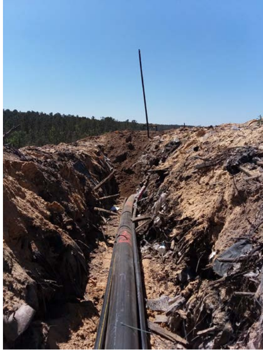
(Photograph 5: 8" header, 2" air, and 2" forcemain placed in same trench)
