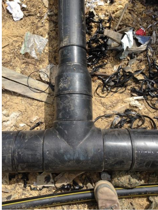
(Photograph 49: 8" tee with 8"x6" reducer to EW-10, HC11, and HC-12)
