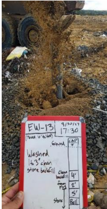
(Photograph 105: W-13 Soil backfill)
