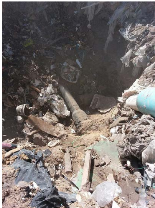
(Photograph 44: Northside tie in point for 8" header)
