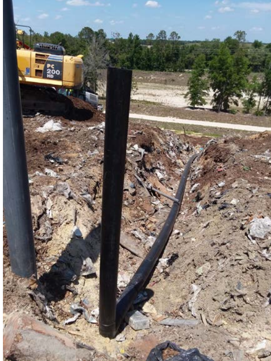
(Photograph 67: 6" lateral and 6" riser for EW-12)
