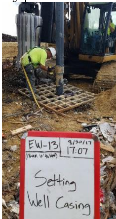
(Photograph 102: W-13 Pipe installation)
