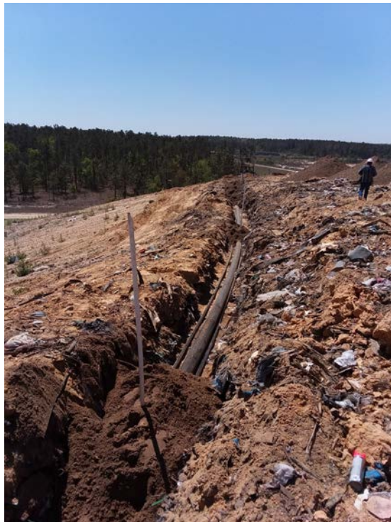
(Photograph 6: 8" header, 2" air, and 2" forcemain placed in same trench)
