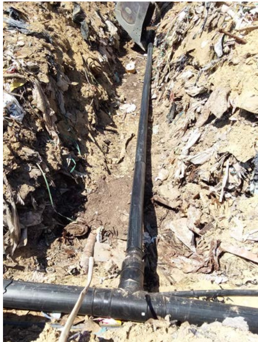
(Photograph 28: 8" tee with 8"x6" reducer and 6" lateral to EW-16)
