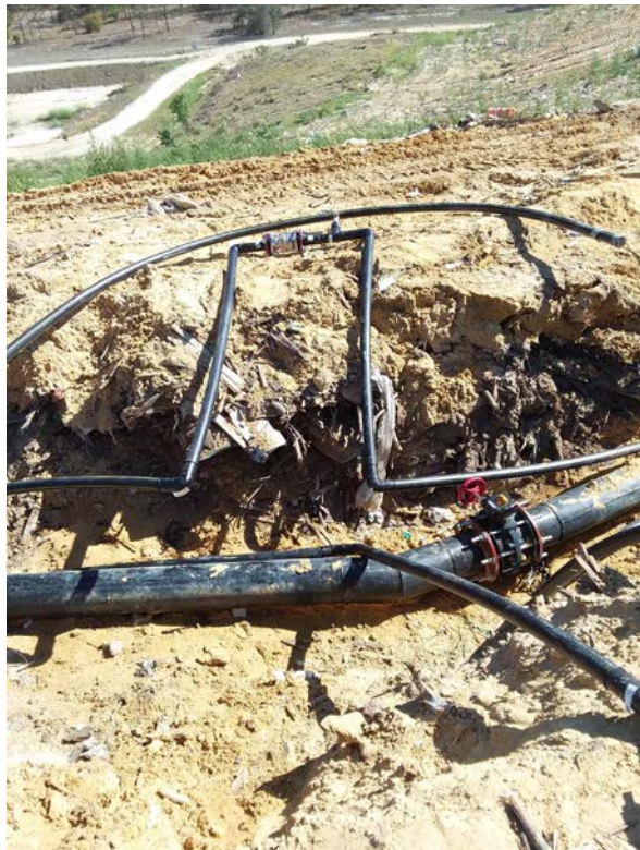
(Photograph 10: 8" valve and 2" air and force main valves)
