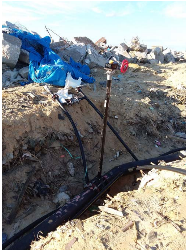
(Photograph 36: 8" valve, 2" air and 2" forcemain valves on northside)
