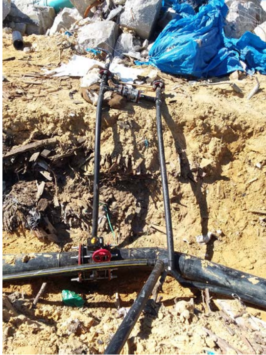
(Photograph 11: 8" valve and 2" air and force main valves)
