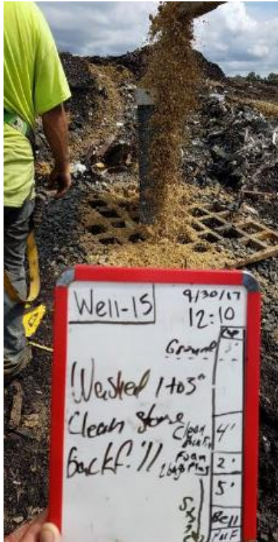
(Photograph 129: W-15 Soil backfill)
