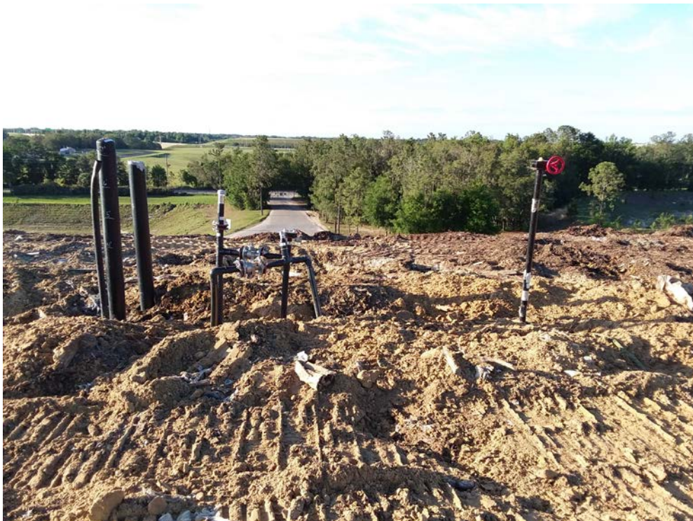
(Photograph 40: Backfilled valve location)
