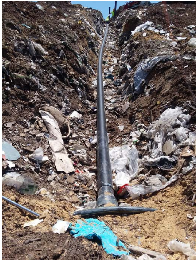
(Photograph 66: 8" tee with 8"x6" reducer and 6" lateral to EW-12)
