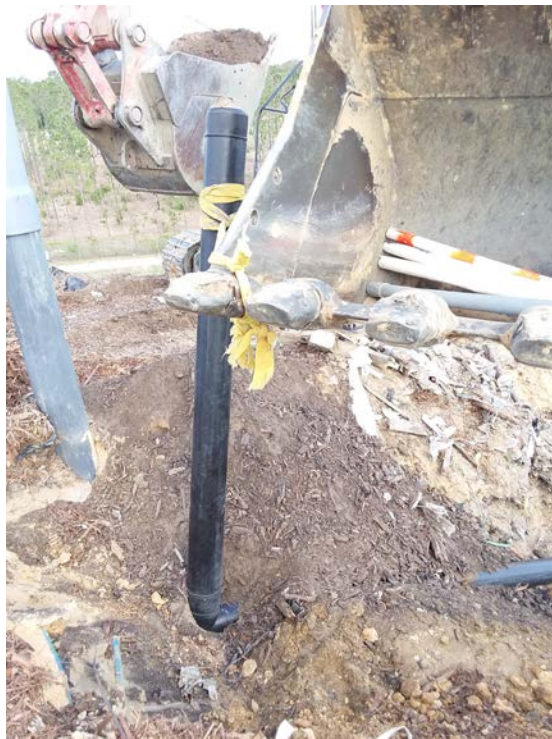
(Photograph 30: 6" riser trench backfill)
