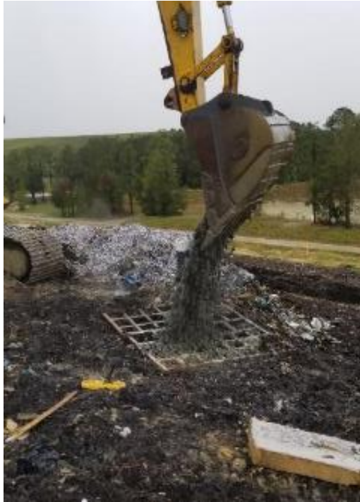
(Photograph 91: W-12 Stone backfill)
