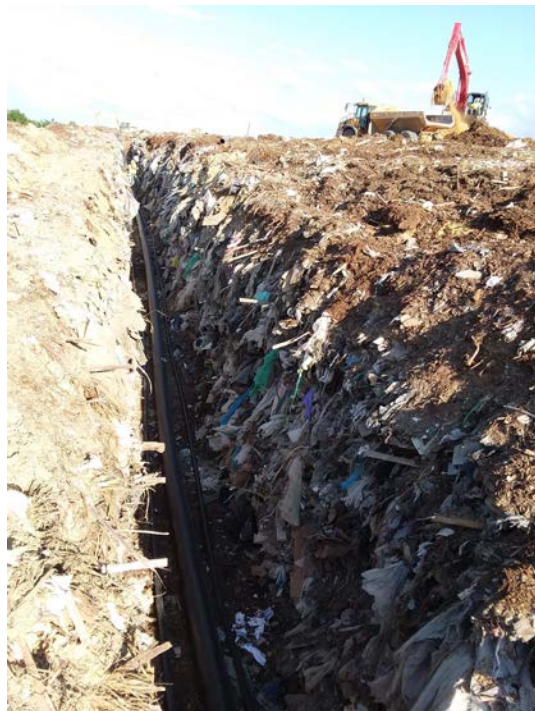
(Photograph 46: 8" header, 2" air, and 2" forcemain placed in same trench)
