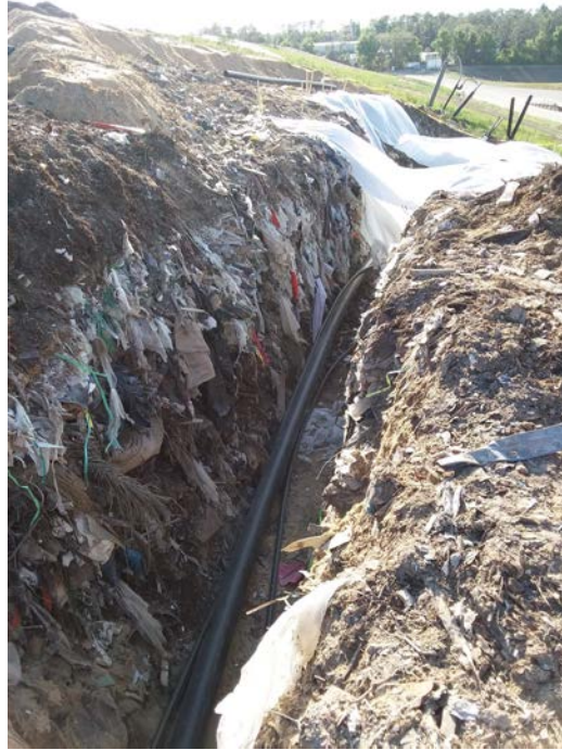
(Photograph 45: 8" header, 2" air, and 2" forcemain placed in same trench)
