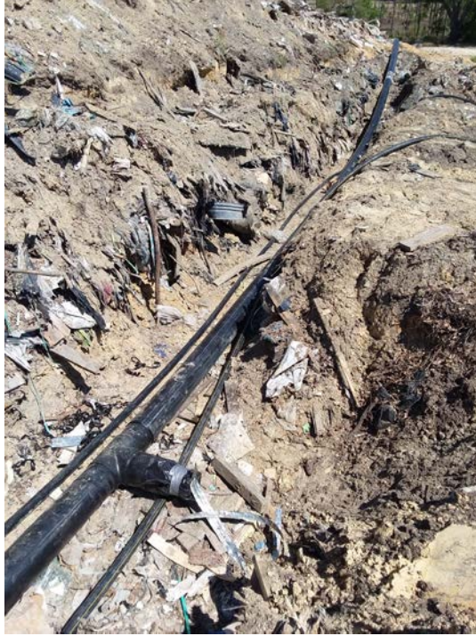
(Photograph 19: 8" tee with 8"x6" reducer for Cell 4 cleanout connection)
