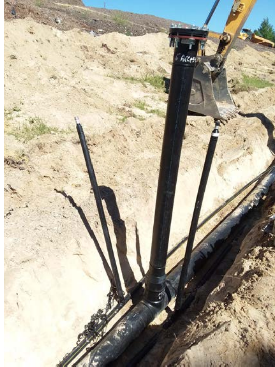
(Photograph 61: 8" tee with 8"x6" reducer and access riser with 2" air and 2" forcemain stub ups)
