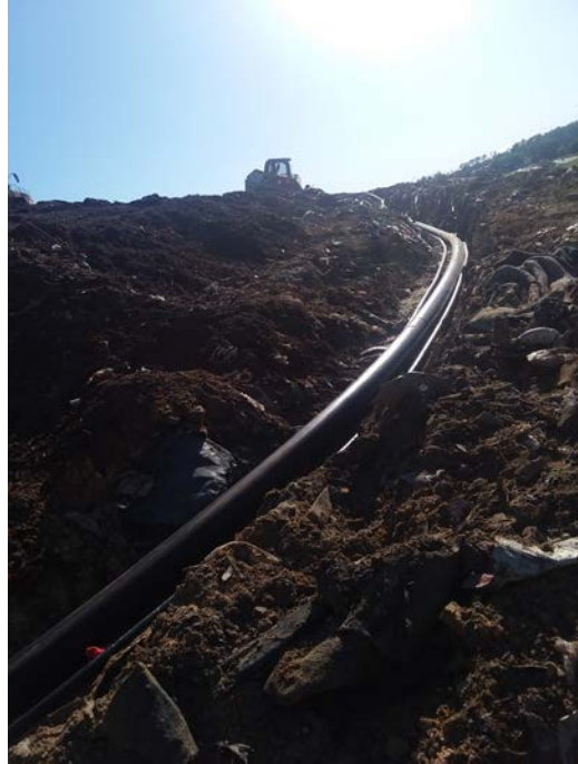
(Photograph 63: 8" header, 2" air, and 2" forcemain placed in same trench)
