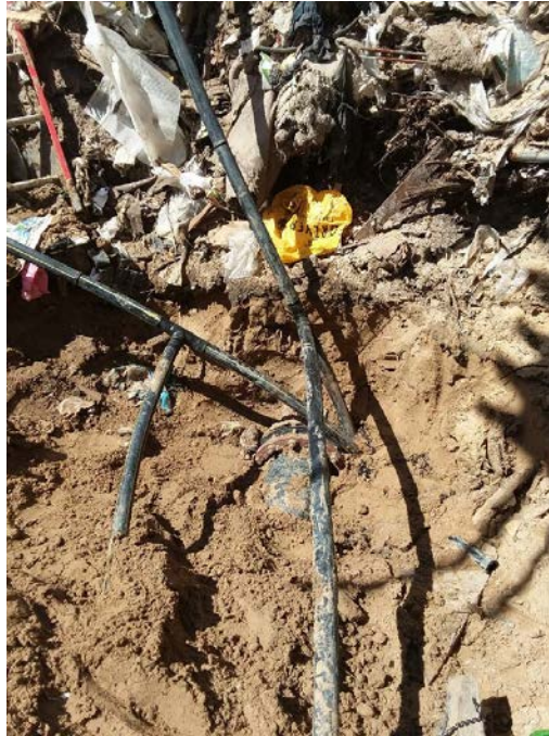
(Photograph 43: 2" air and 2" forcemain tie in on southside)
