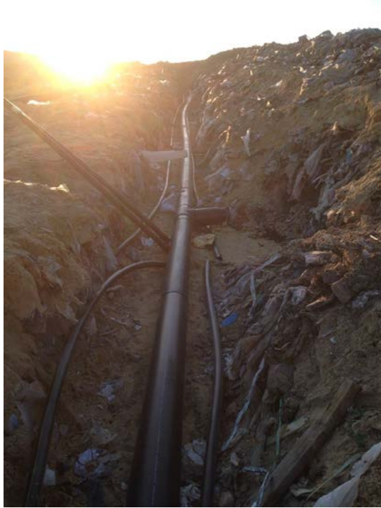
(Photograph 15: 8" header, 2" air, and 2" forcemain placed in same trench with 8" tee with 8"x6" reducer for EW-15)
