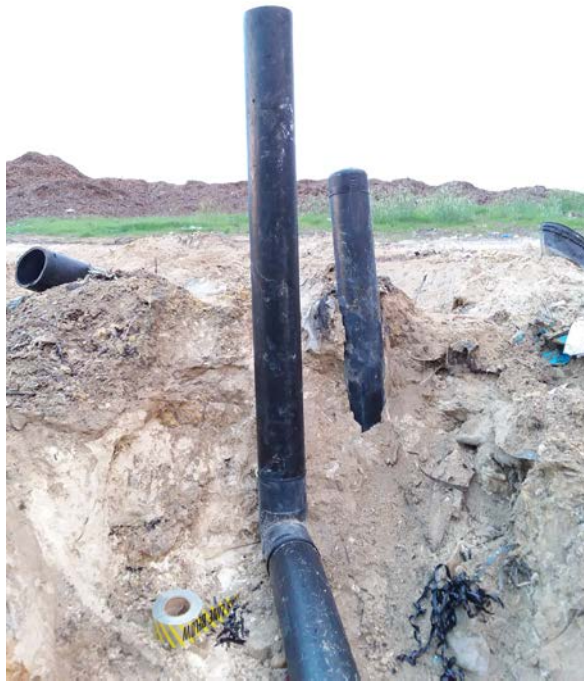
(Photograph 73: 6" riser for Cell 3 cleanout connection)
