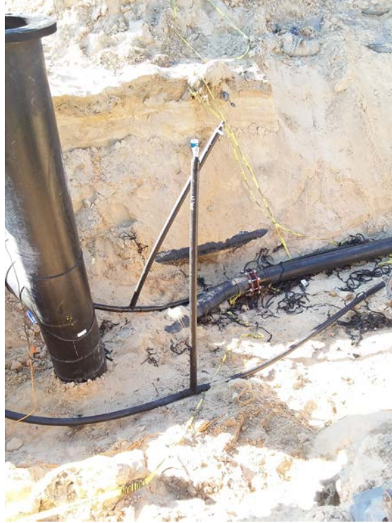
(Photograph 39: 2" air and 2" force main stub ups at CS-4)
