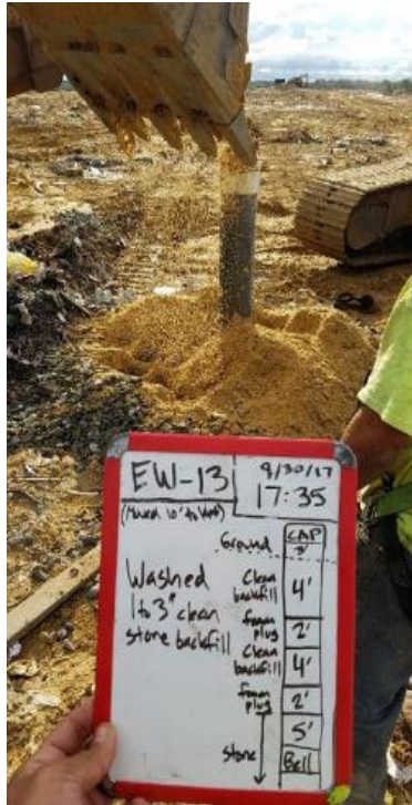
(Photograph 107: W-13 Soil backfill)
