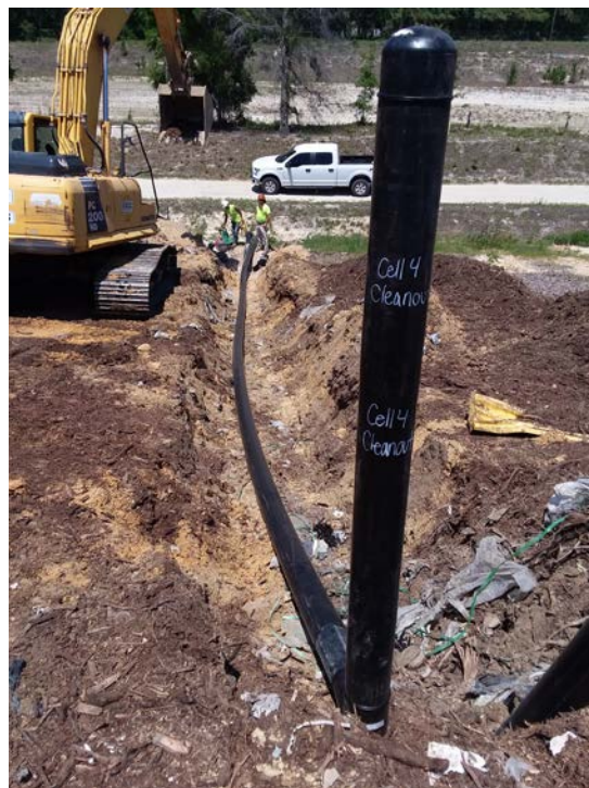
(Photograph 68: 6" riser for Cell 4 cleanout connection)
