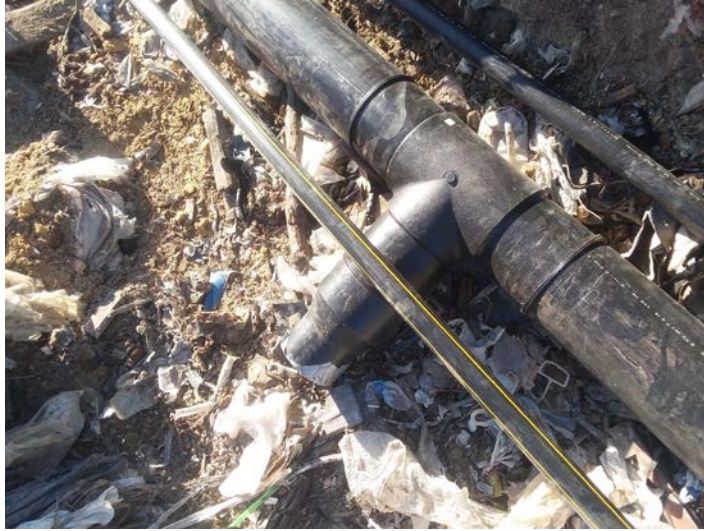
(Photograph 65: 8" tee with 8"x6" reducer for Cell 4 cleanout connection)
