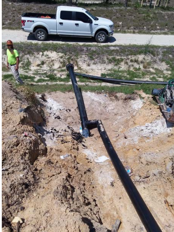
(Photograph 69: 6" tie into Cell 4 cleanout connection)
