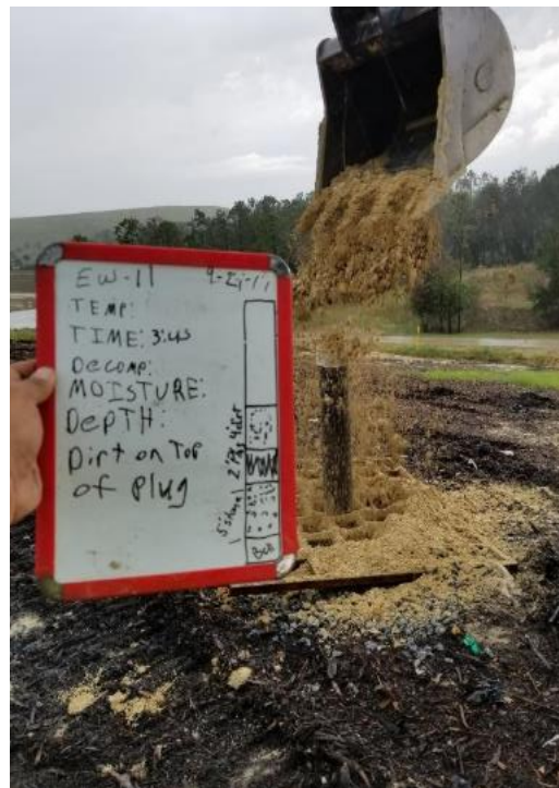
(Photograph 82: W-11 Soil backfill)
