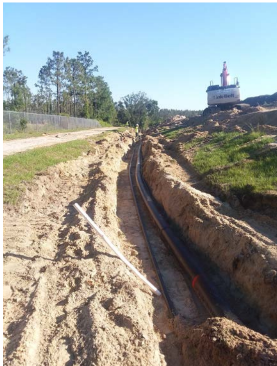
(Photograph 62: 8" header, 2" air, and 2" forcemain placed in same trench)
