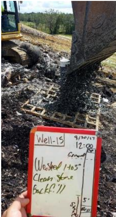
(Photograph 127: W-15 Stone backfill)
