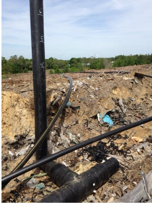
(Photograph 51: 8" tee with 8"x6" reducer and 6" riser for Cell 3 cleanout)
