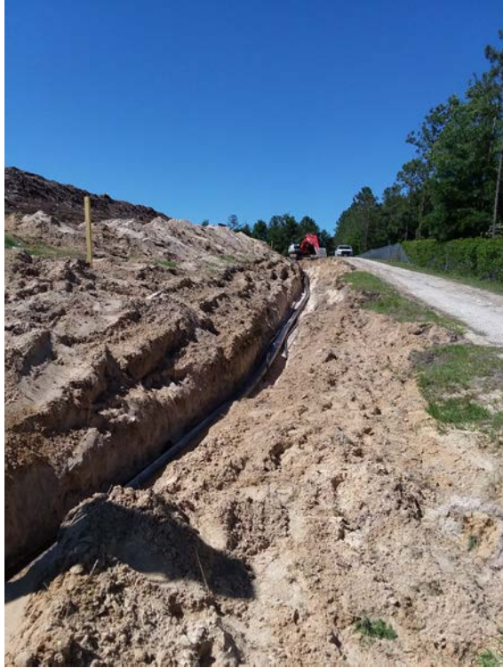
(Photograph 59: 8" header, 2" air, and 2" forcemain placed in same trench)
