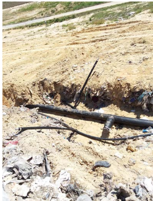
(Photograph 18: 8" tee with 8"x6" reducer for EW-16)
