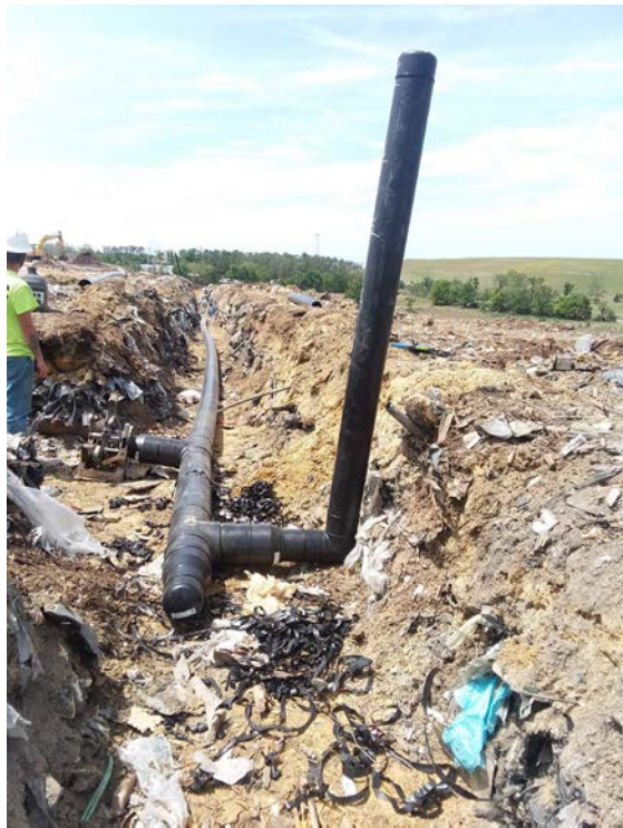
(Photograph 48: 8" tee with 8"x6" reducer and 6" riser for Cell 3 cleanout)
