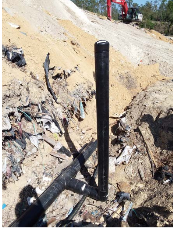
(Photograph 29: 6" riser for Cell 4 cleanout connection)
