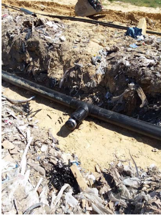
(Photograph 13: 8" tee with 8"x6" reducer for EW-14)
