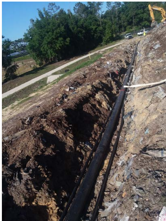
(Photograph 64: 8" header, 2" air, and 2" forcemain placed in same trench)
