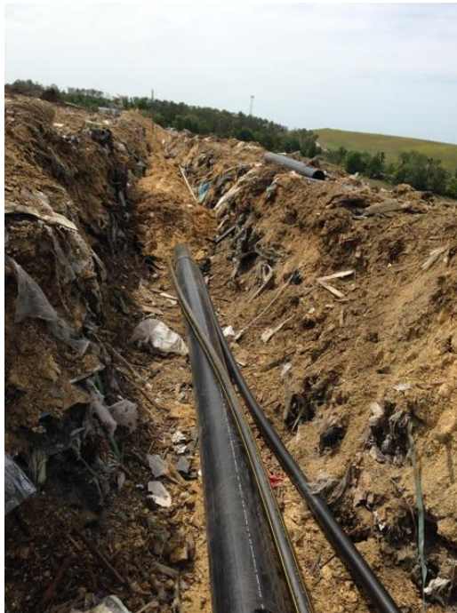
(Photograph 52: 8" header, 2" air, and 2" forcemain backfilling)
