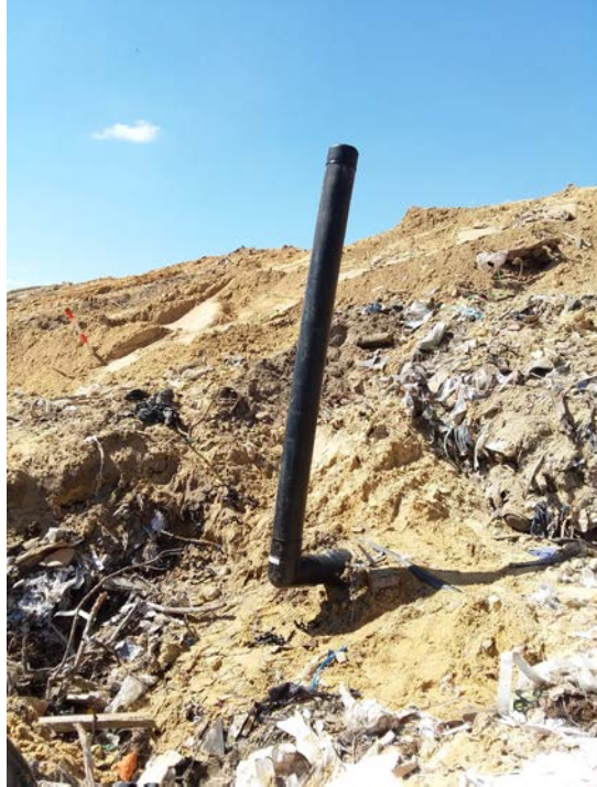
(Photograph 27: 6" riser for Cell 3 cleanout connection)
