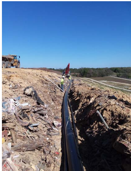
(Photograph 12: 8" header, 2" air, and 2" forcemain placed in same trench)
