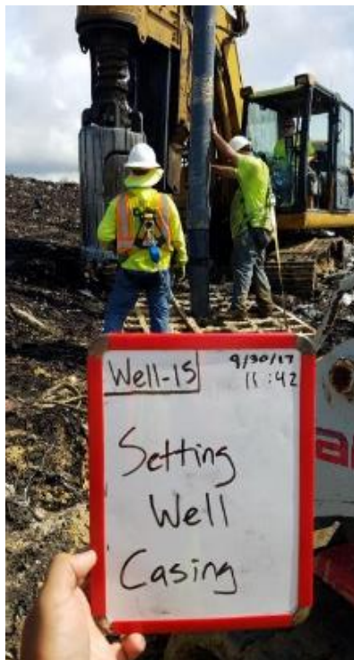
(Photograph 126: W-15 Pipe installation)
