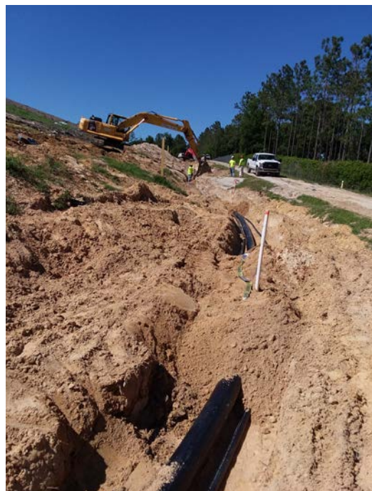
(Photograph 58: 8" header, 2" air, and 2" forcemain backfilling and placing caution tape)
