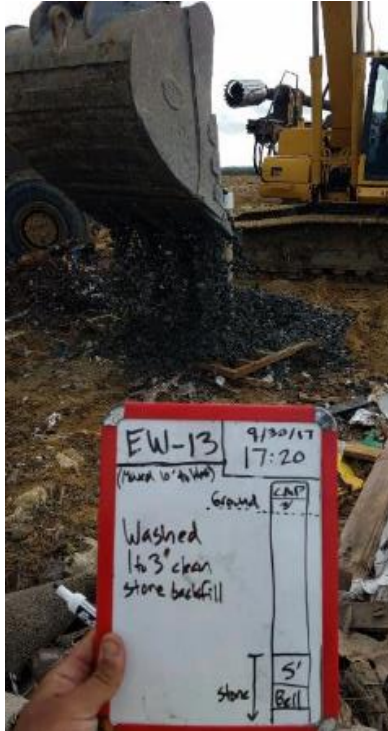
(Photograph 103: W-13 Stone backfill)
