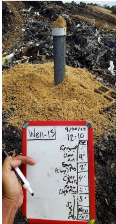
(Photograph 131: W-15 Soil backfill)
