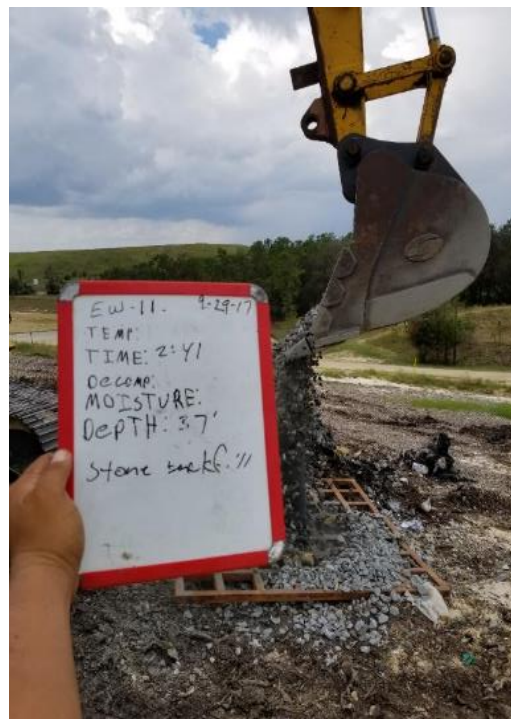
(Photograph 80: W-11 Stone backfill)
