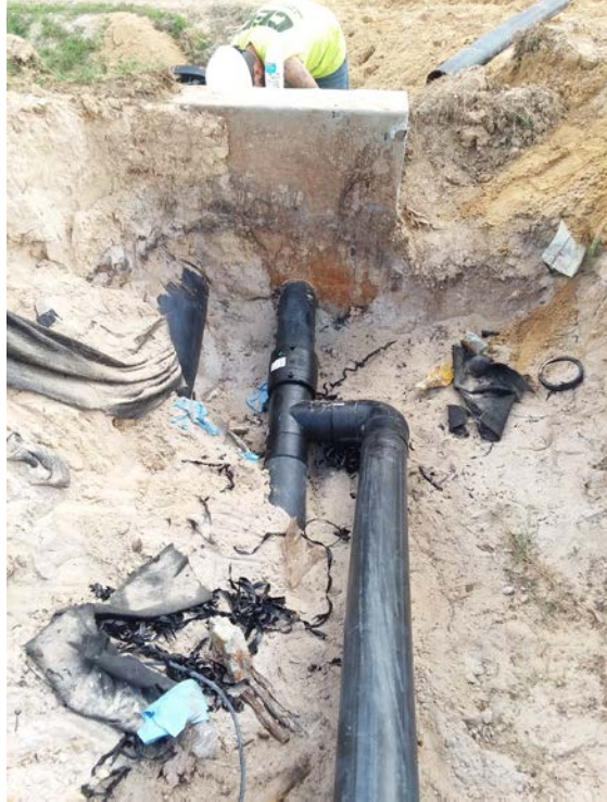
(Photograph 71: 6" tie into Cell 4 cleanout connection)
