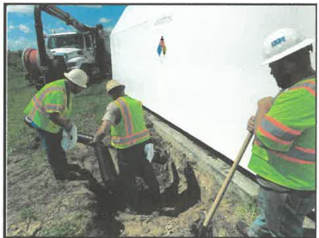
Excavation of Impacted Soil
