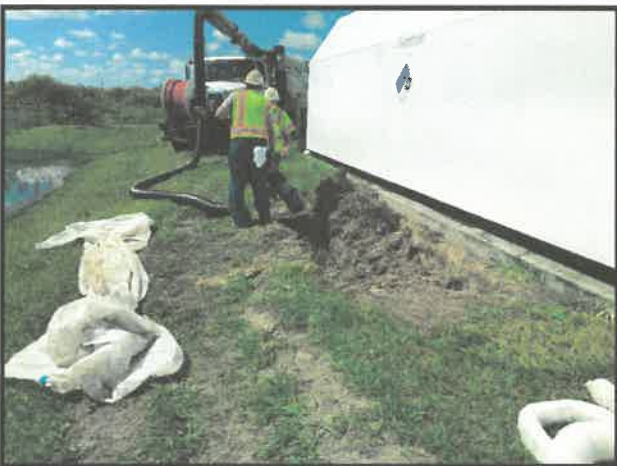
Excavation of Impacted Soil
