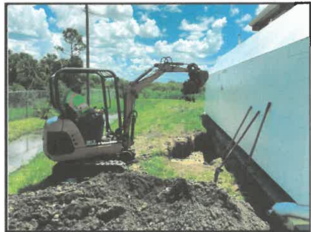
Backfilling Excavation
