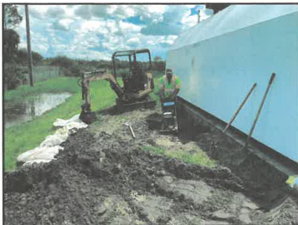
Compacting Backfill
