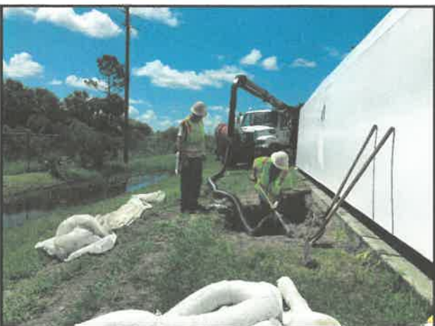
Excavation of Impacted Soil
