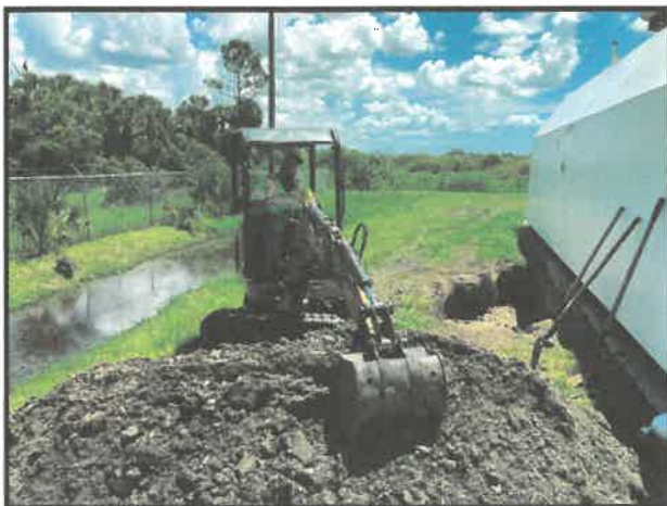
Backfilling Excavation
