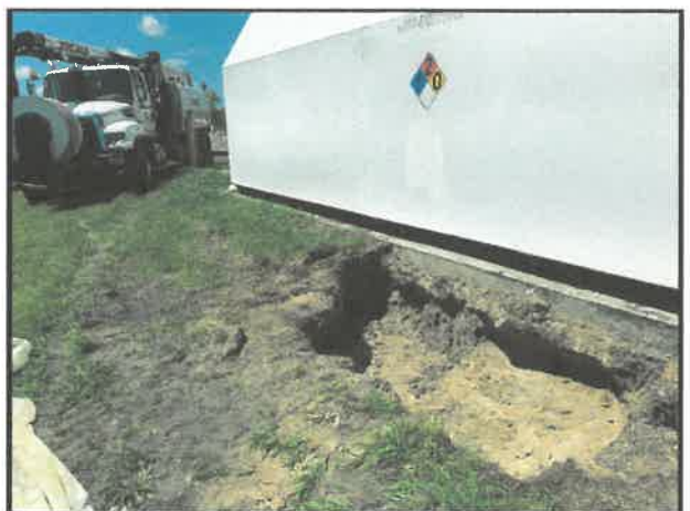
Excavation of Impacted Soil
