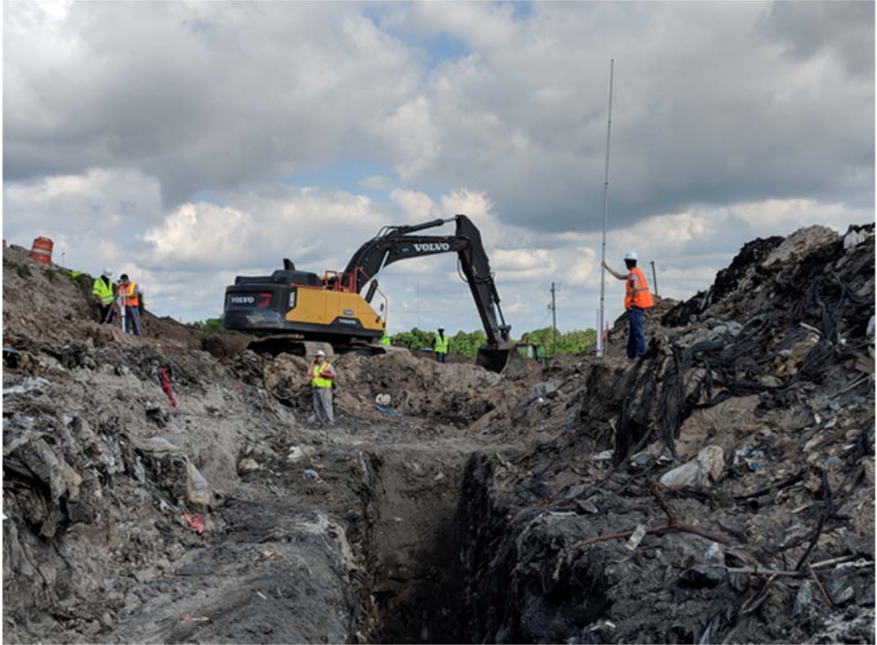
Figure 5-6. Determining the height of the piezometer above the ground surface with a surveying level.
