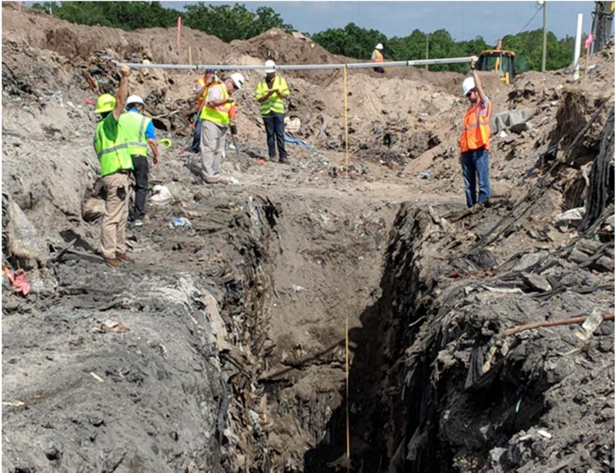
Figure 5-7. Measuring the depth to the top of the clay liner.
