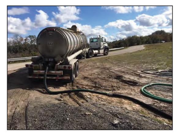
Photograph 5. Tank Truck Used to Pump 6,000 Gallons of Water with Tracer Dye "Donut" into the Phase II Header Access Point
