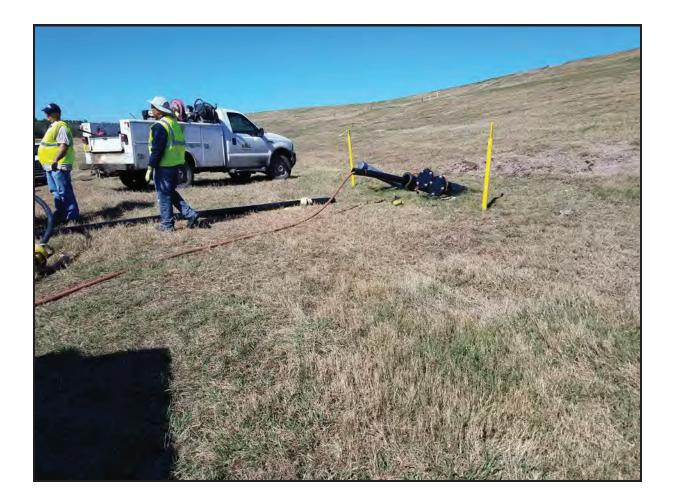
Photograph 4. <sup>3</sup>/<sub>4</sub>" Hose from the Tank Trailer Pump Delivering the Dye Mixture into CO 1-1
