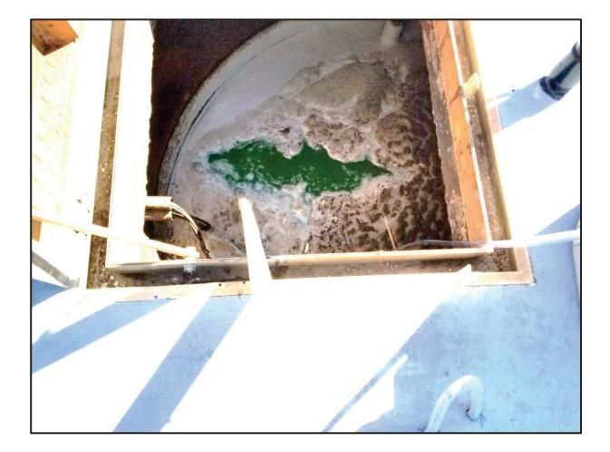
Photograph 6. First Observation of Dye in the PS-A Wet Well at 12:25 p.m.
