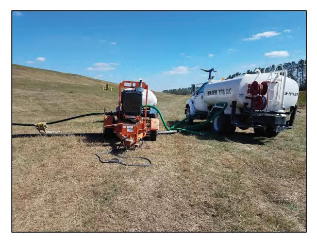
Photograph 5. Portable Pump Used to Inject 2,000 Gallons of Water
