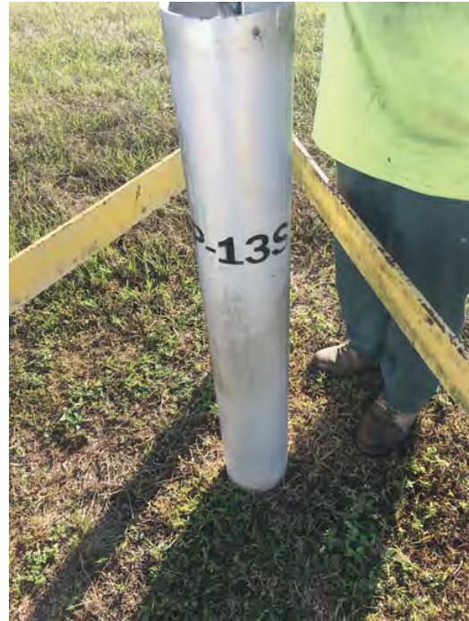
Date: 11/8/2018 Description: Preparing P-13S for grouting
