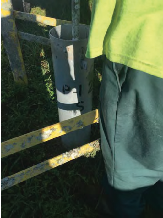
Date: 11/8/2018 Description: Inserting tremmie tube into P-12S
