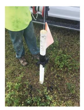
Date: 11/5/18 Description: Measuring the depth of SB-03 prior to grouting
