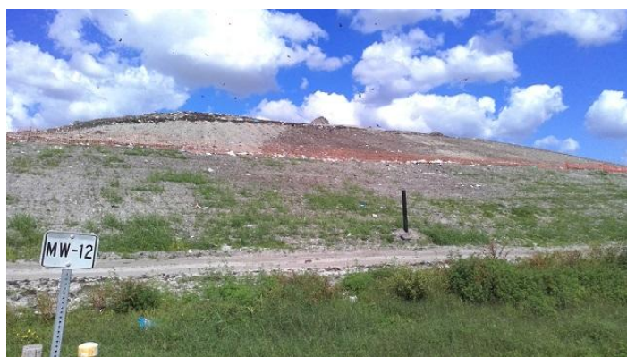
Area with Poor Intermediate Cover
